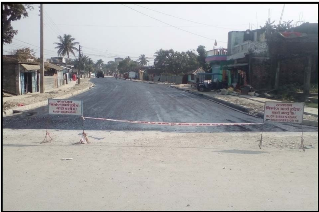
Prime coat work at R2 (Tinpaini to Pani Tanki)
