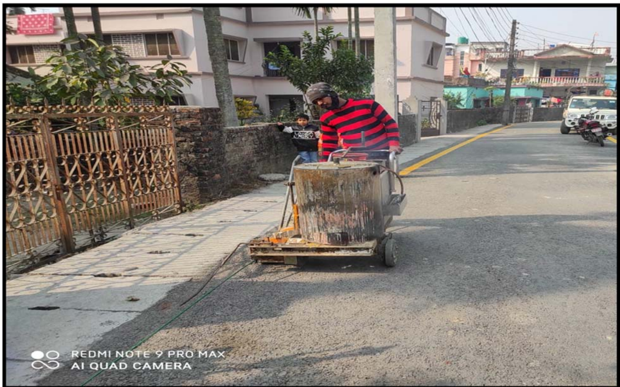
Thermoplastic work at T3Line22A
