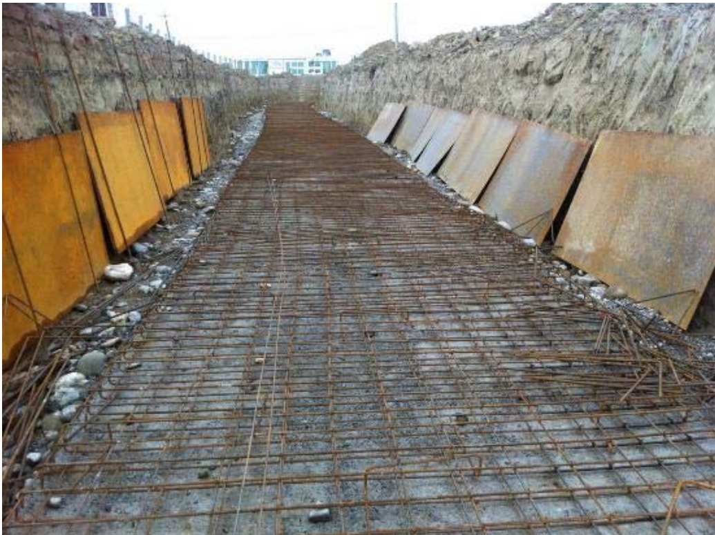
24. RCC Drain Construction at Line B2
