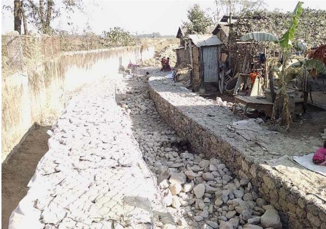
14. Gabion works at Outlet S11
