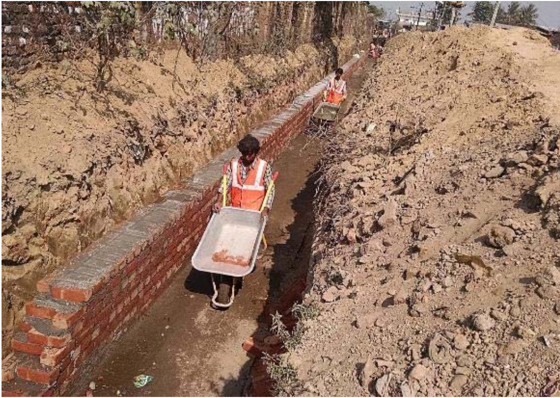
1. Construction of Brick Drain at R2
