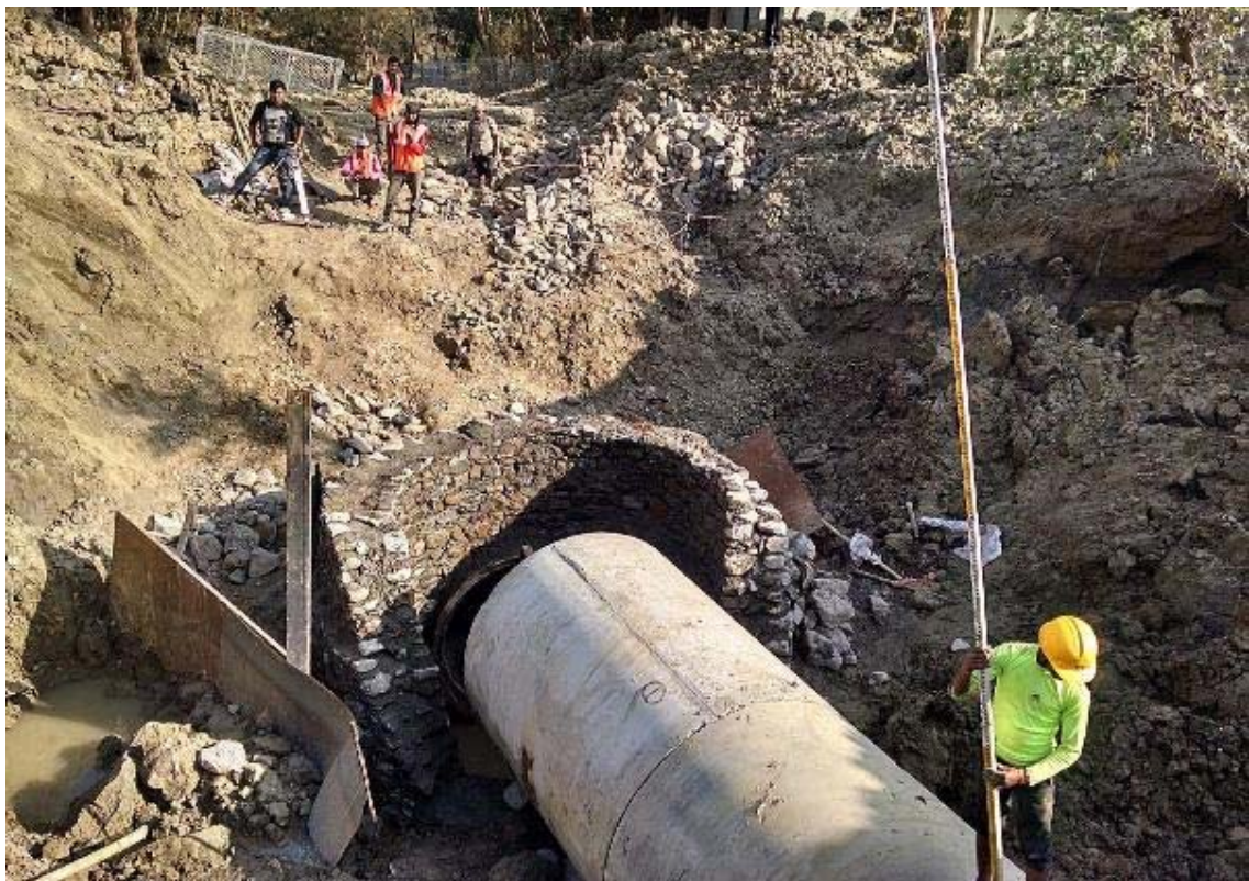
15. Manhole construction and Pipe laying at S13
