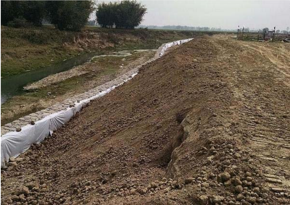
5. Gabion wall final layer completed at WWTP, Jatuwa
