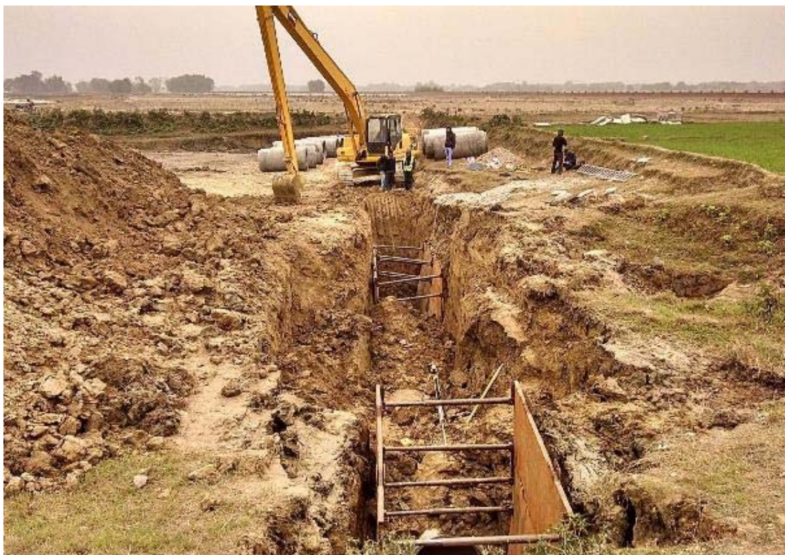
11. Pipe Laying using Shoring at T2
