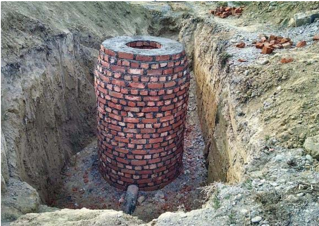
2. Brick Manhole Construction at T3 Secondary Line
