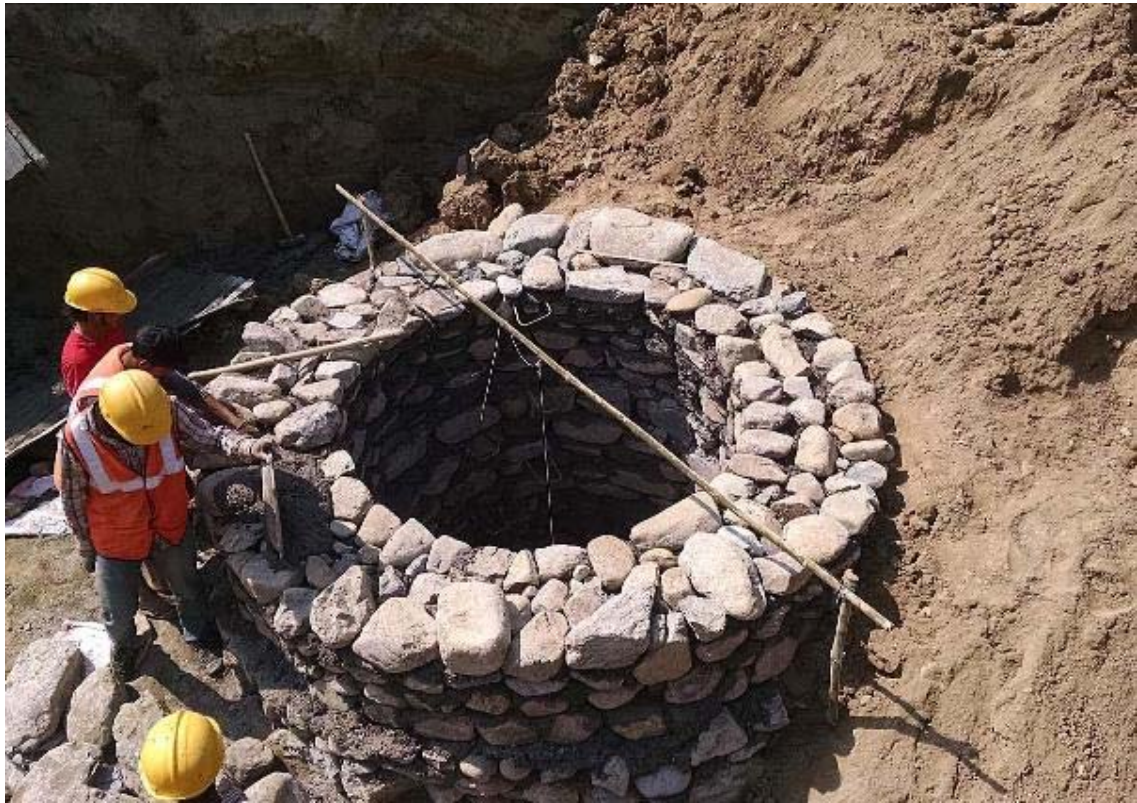
10. Construction of Stone Masonry Manhole at Line T2
