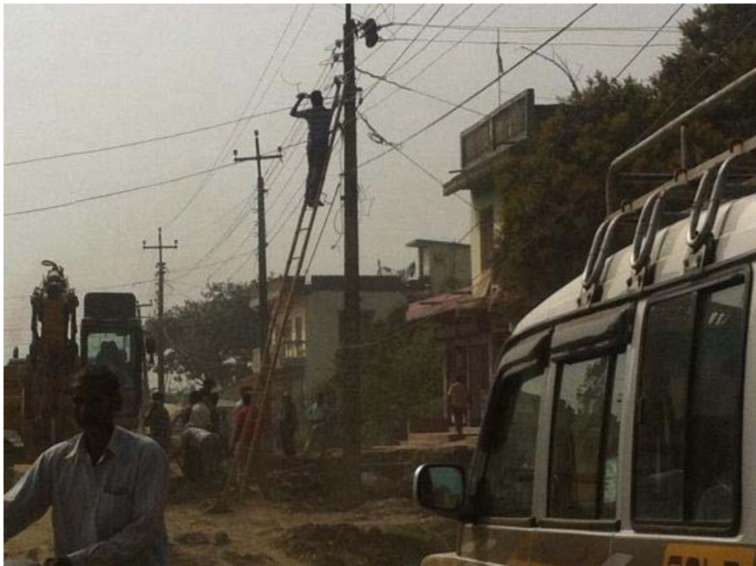
19. Electric Pole Shifting at Road R2
