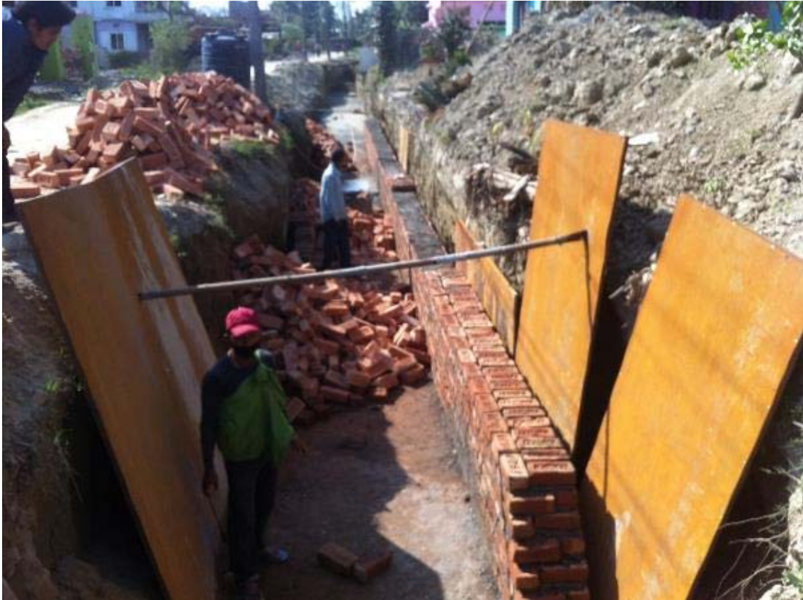
21. Brick Drain Construction at Line S13
