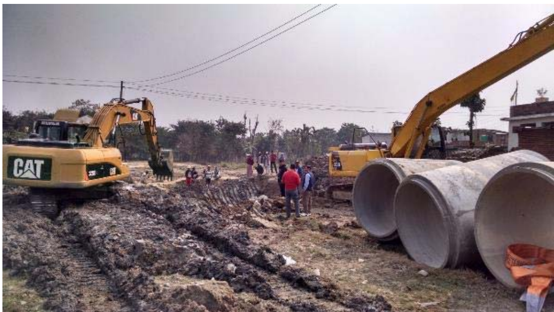
4. Installation of 1600 dia Hume Pipe at S13
