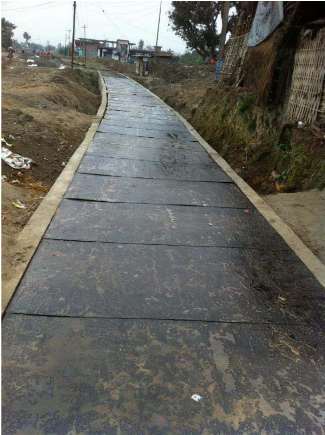
22. Formworks for Slab at Line B1
