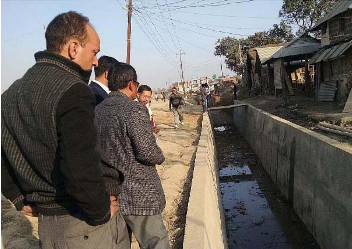
16. RCC Drain construction visit at S13
