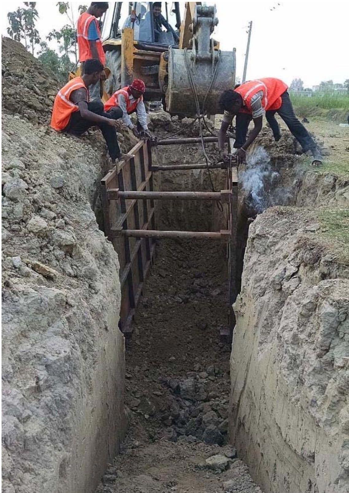
7. Shoring of trenches at Secondary lines
