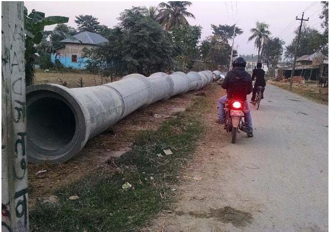
13. Hume pipe stacked for laying at T3
