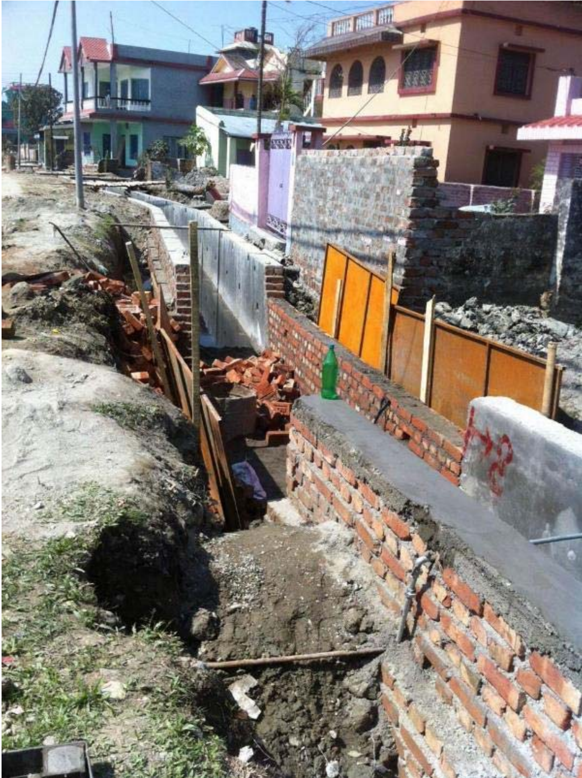
20. Brick Drain Construction at Line B2
