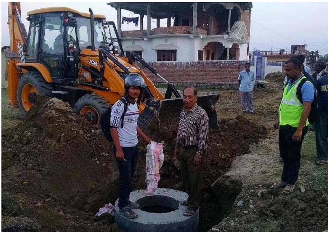
9. Installation of Precast Manhole
