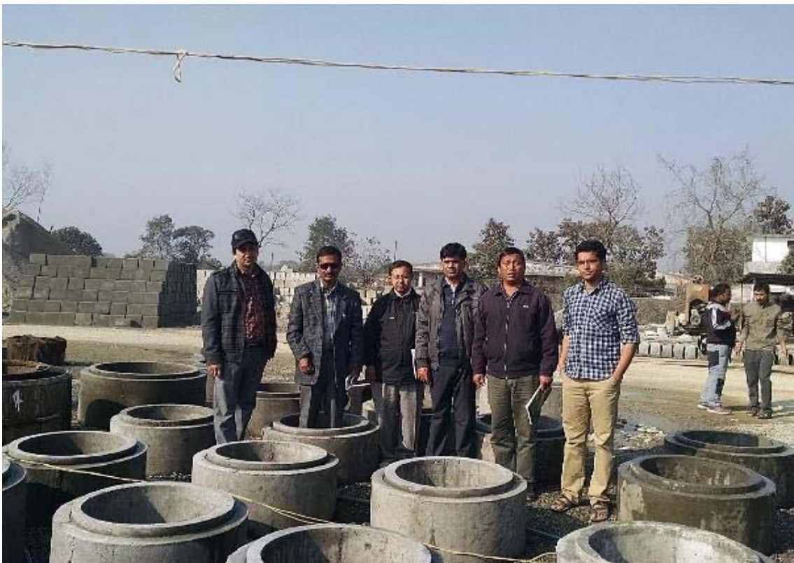
17. Precast chamber units at Yard
