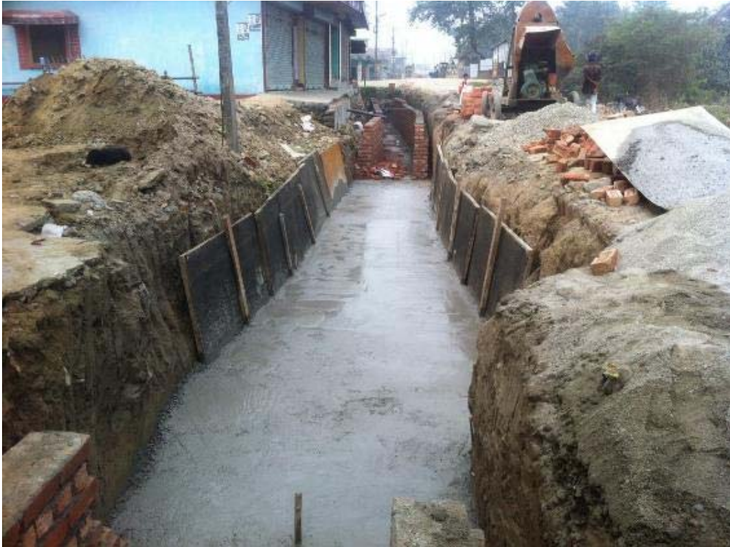
18. Brick Drain Construction at CN2
