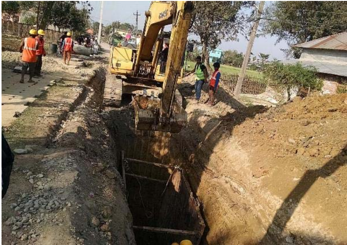
8. Shoring before pipe laying at Line T3 Trunk
