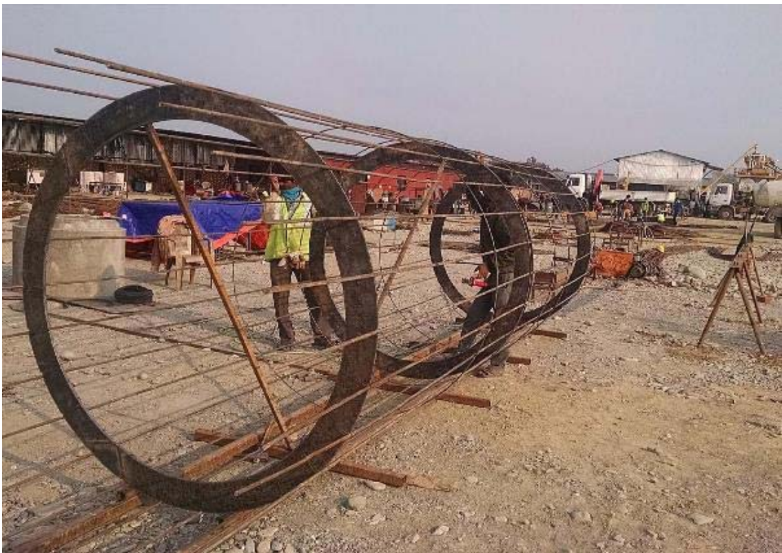
6. Rebar preparation for RCC manhole
