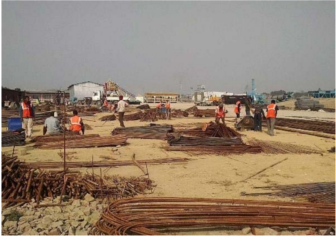
12. Bar cutting and bending at Yard
