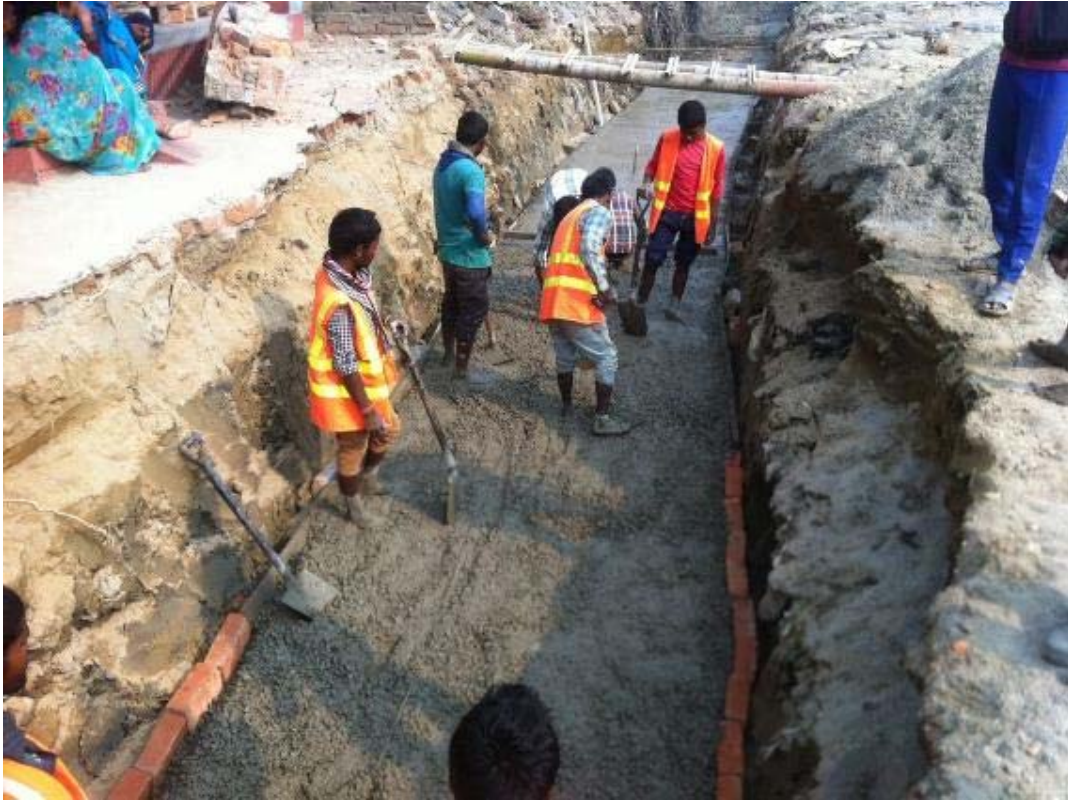
23. Brick Drain Concreting at CN2
