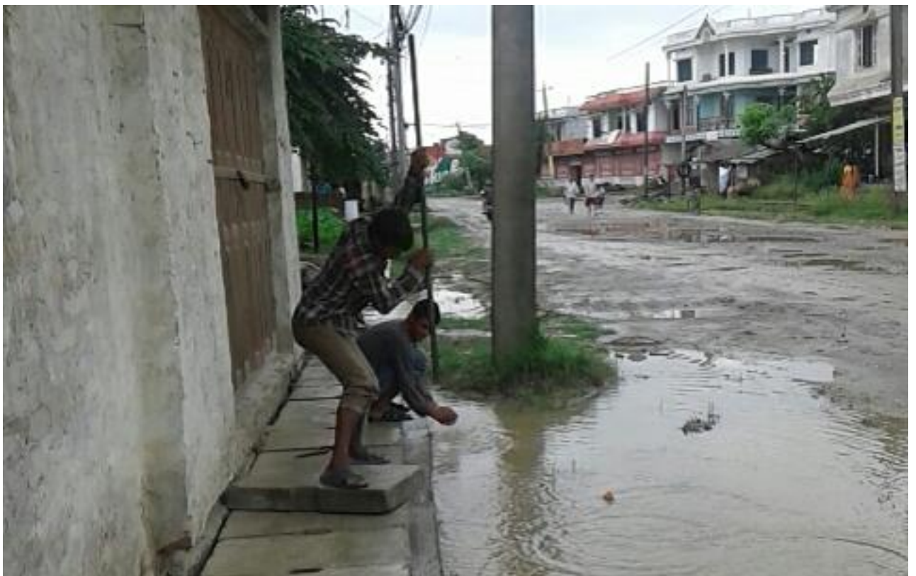
Figure 6 Draining of road surface water
