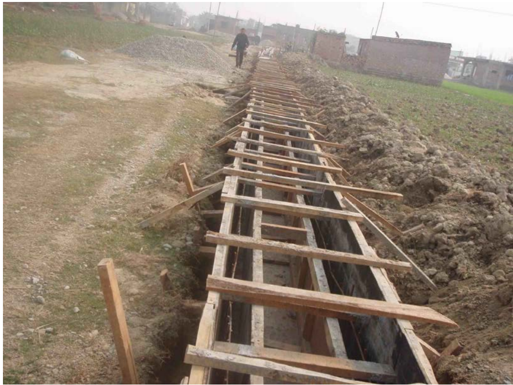
Formwork for Road Side Drain at Sewer Lines
