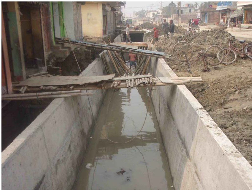
RCC Drain at B3
