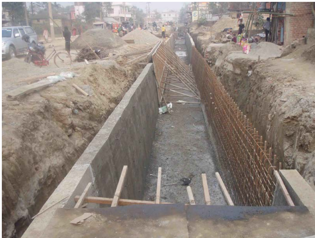
RCC Drain at B1
