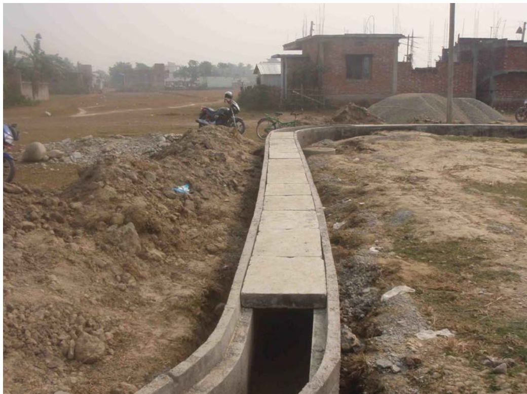
Concrete Road Side Drain at Sewer Lines
