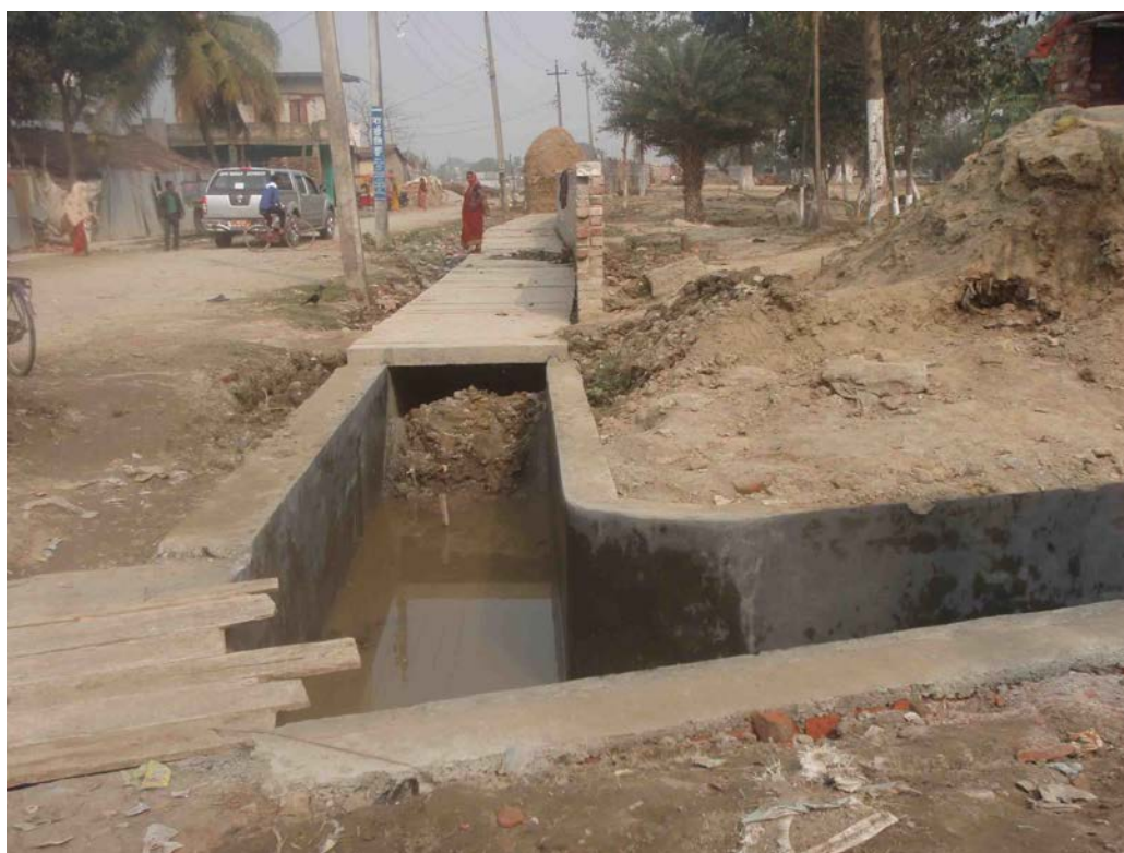
Brick Masonry Drain at Rani
