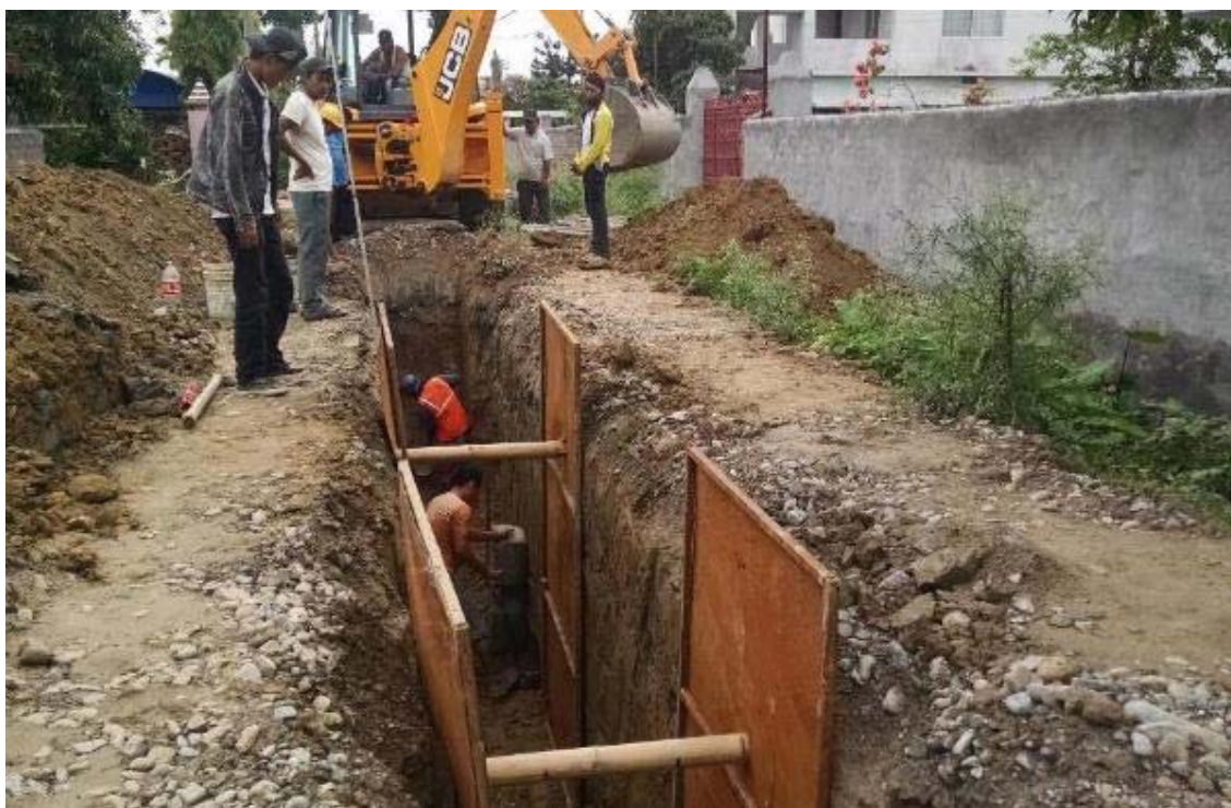
Figure 12 HDPE pipe laying at sewer line T2 secondary
