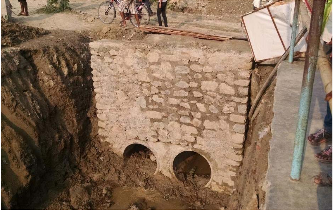
Figure 5 Syphon head wall of Line B1
