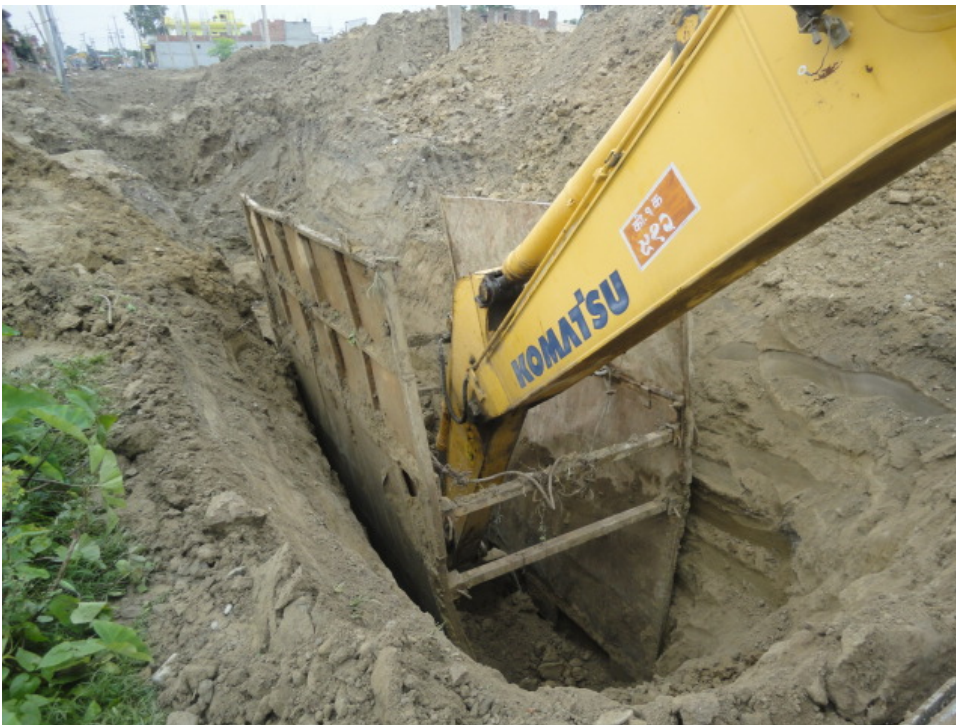
Trench excavation of Trunk line at T3, Dharambandh Road
