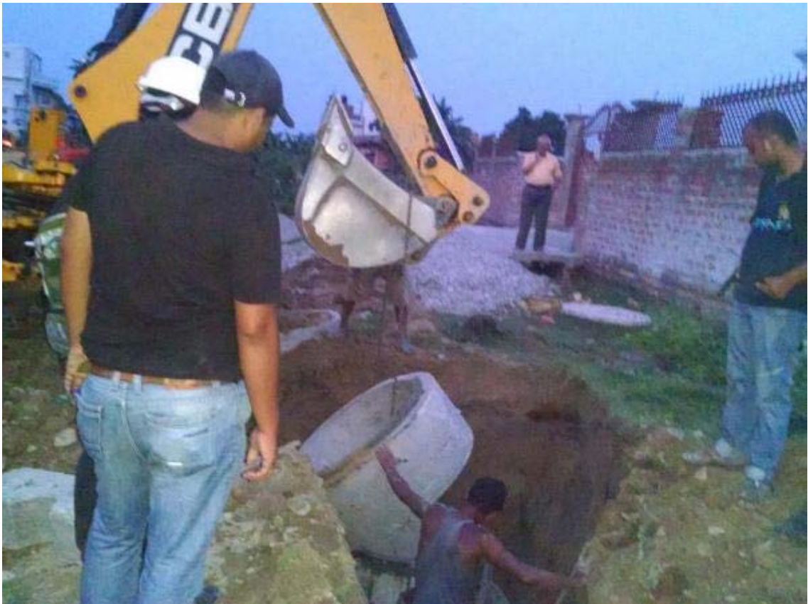
Figure 6 Precast Chamber Installation at Sewer line T2 Secondary
