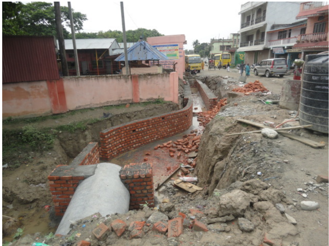
Connection of Syphon and Storm Drain of CN3, near Sagarmatha H S School
