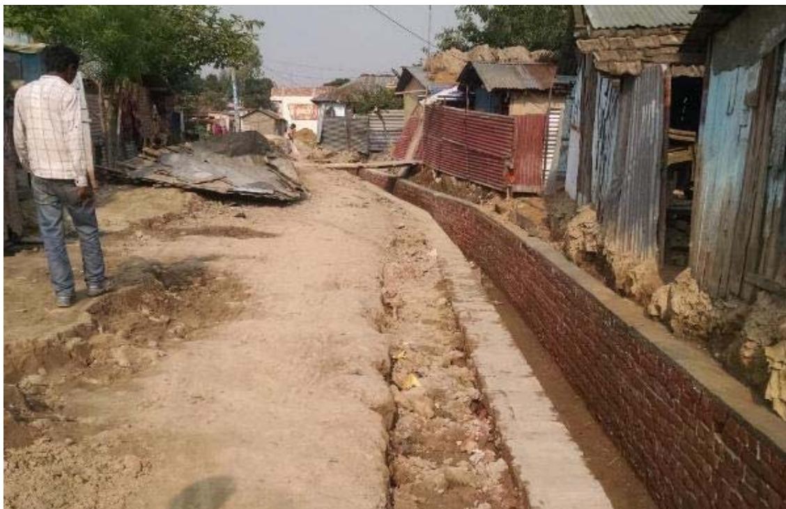
Figure 15 Brick Drain construction at Line Rani
