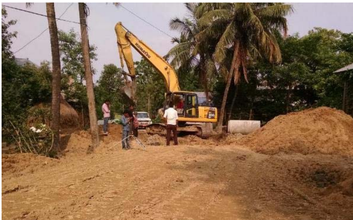
Figure 18 Hume pipe laying at Trunk line T2
