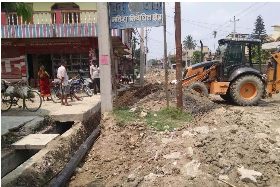
Figure 3 HDPE pipe laying for water supply at R2 Road
