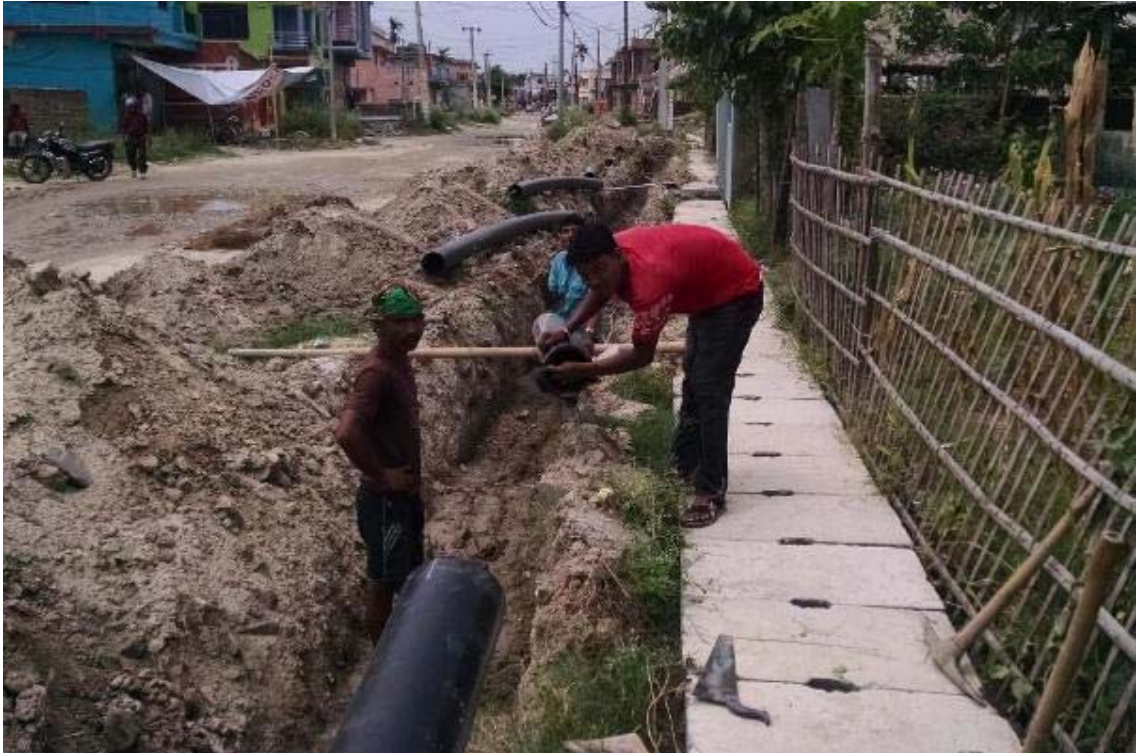
Figure 7 HDPE pipeline laying for water supply at R2
