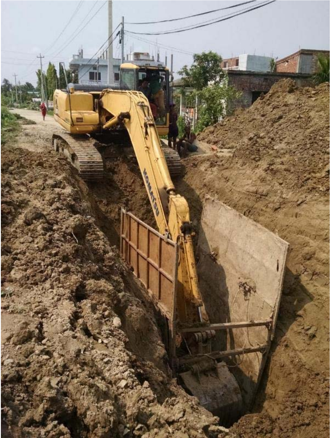
Figure 17 Hume Pipe excavation at line T3 Trunk
