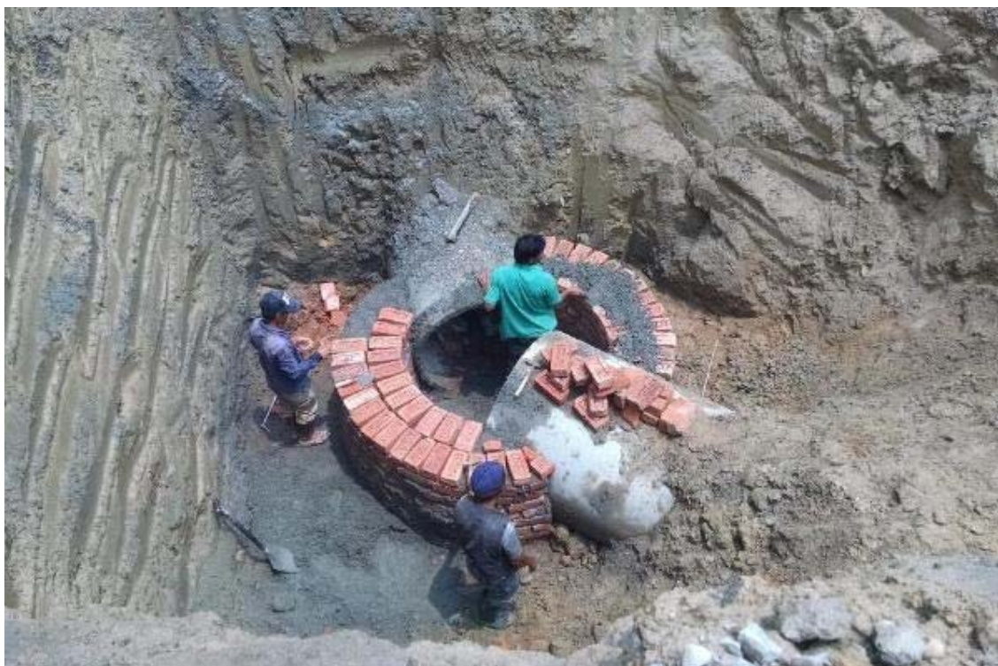
Figure 16 Brick manhole construction at line T2 Trunk Jatuwa Chowk
