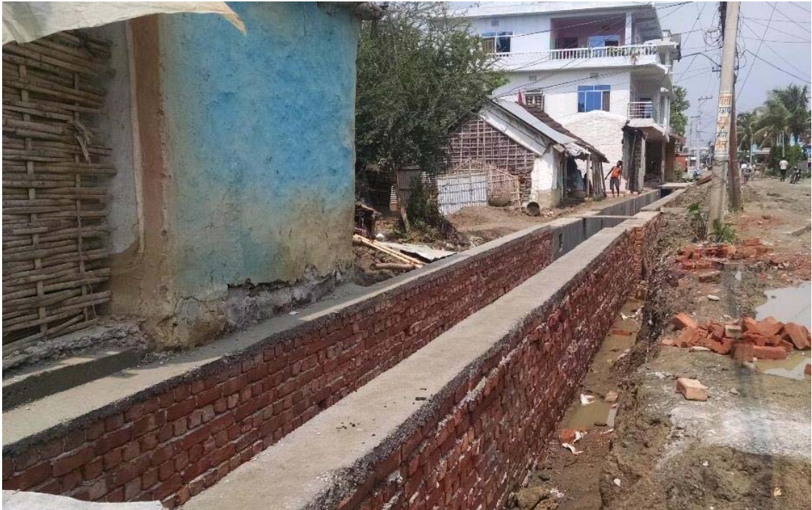
Figure 1 Brick Drain Construction at Rani
