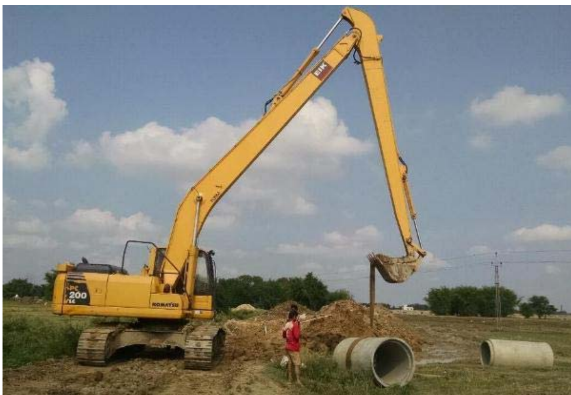
Figure 10 Hume Pipe Laying at Jatuwa (T2 Trunk)
