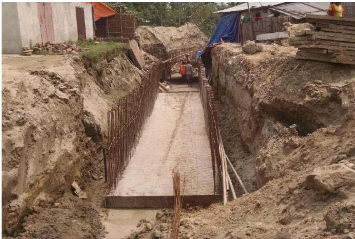
Figure 13 RCC Drain construction at line B2 near outlet
