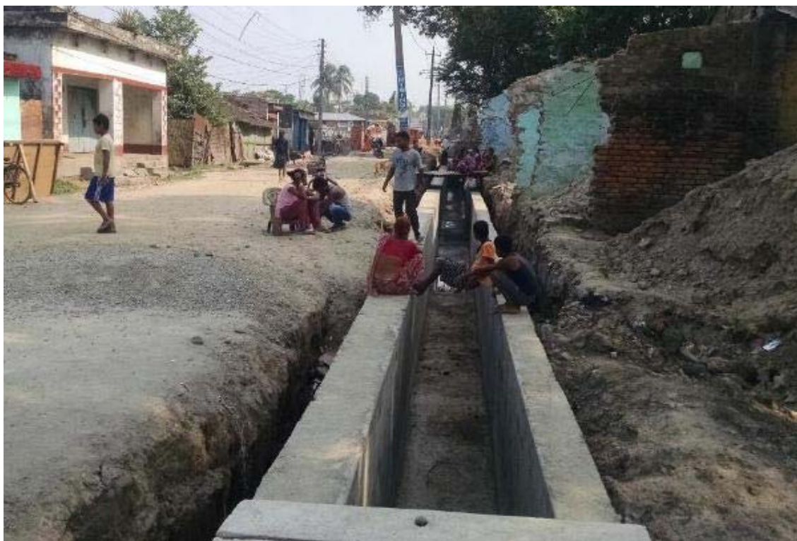
Figure 14 Brick drain construction at line Rani
