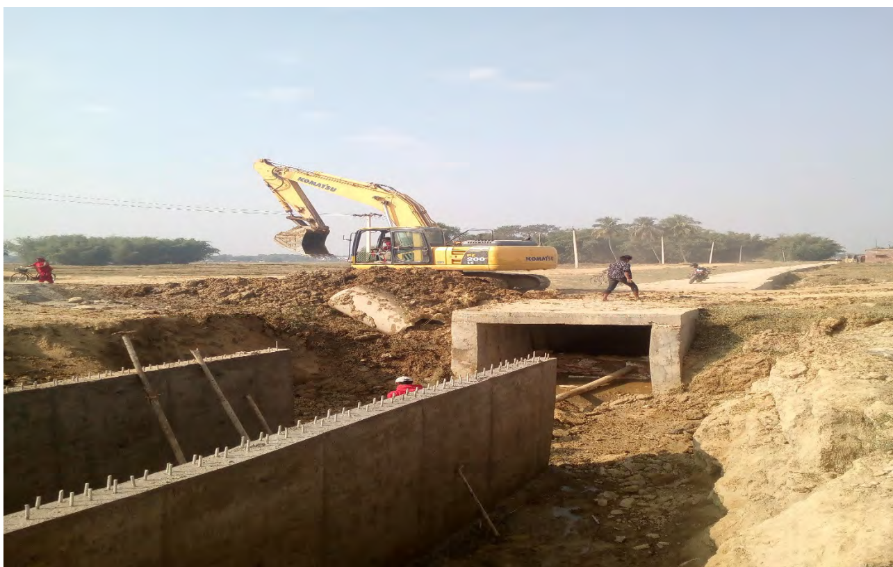
Picture 2 RCC Drain Construction work at S5(Jatuwa)
