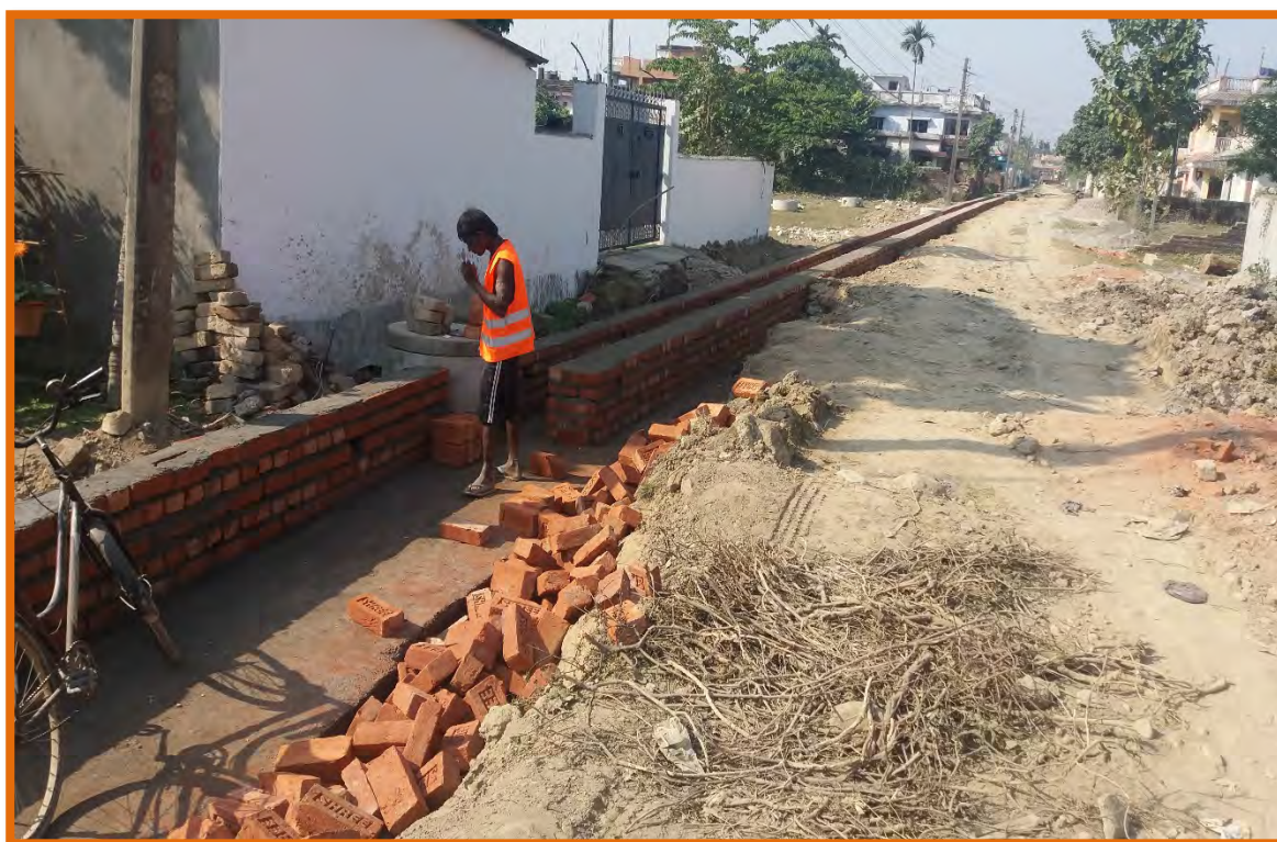
Road side drain at R25
