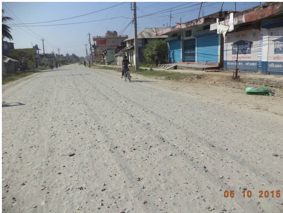
Gravel Sub-base Surface at R2 road (100m) found in good grade and camber after rainy season
