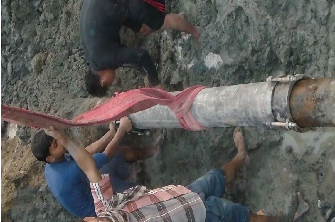
Picture 1 Repair and maintenance work of water supply pipe
