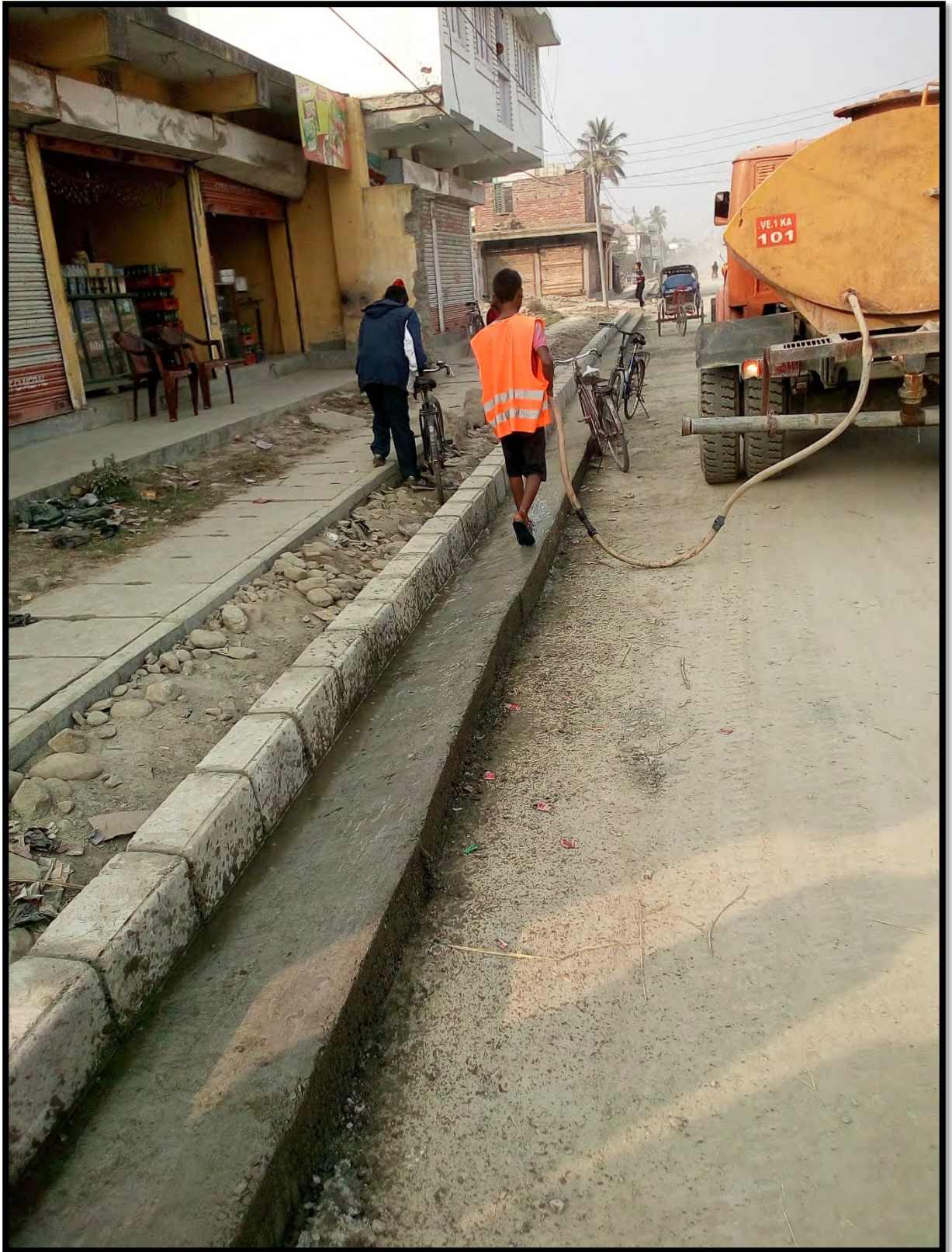
Kerbstone and Gutter curing at R2 Road
