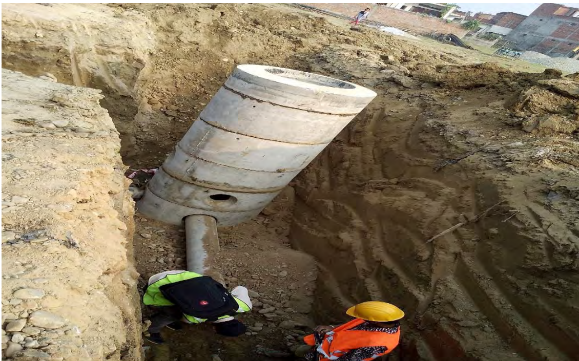
Picture 2 Construction of Sewer line
