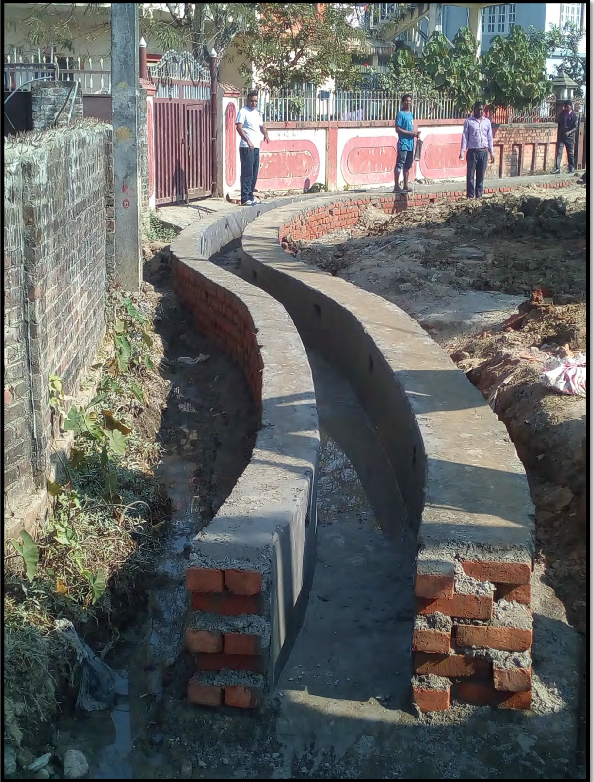
Brick Masonry road side drain at R28 road
