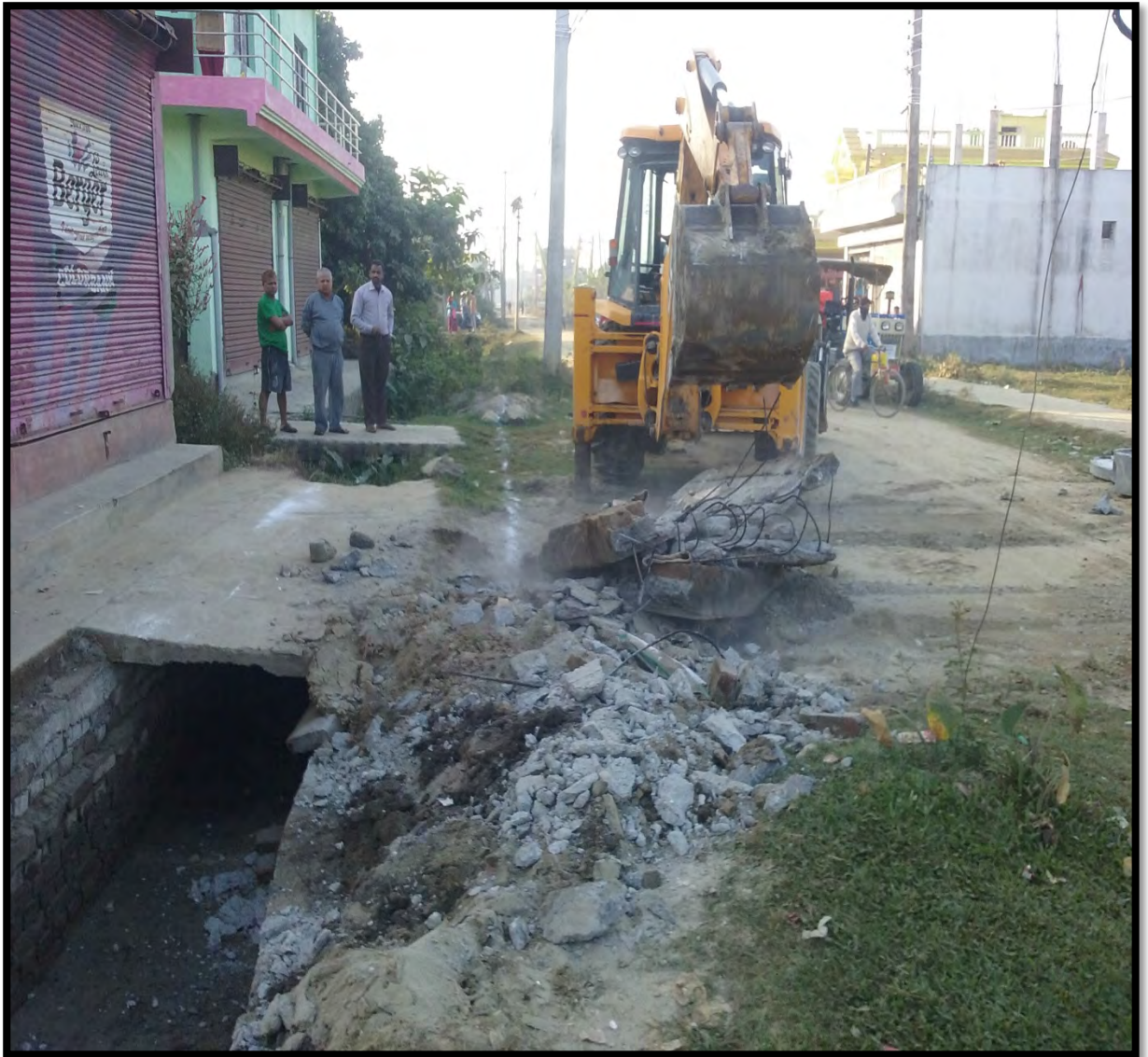
Dismantle Existing RCC Slab and Brick Masonry drain at R3 road
