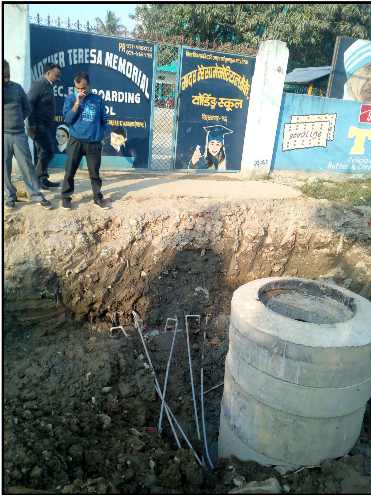
Repair and maintenance water supply pipe
