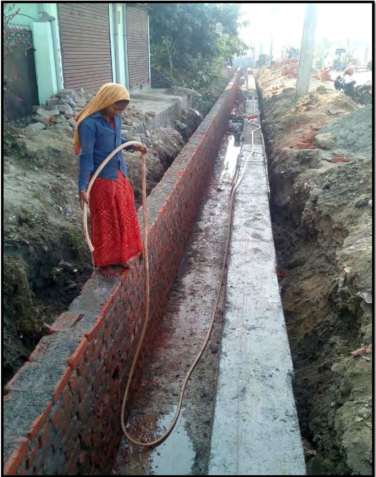
Brick Masonry road side drain at R3 road
