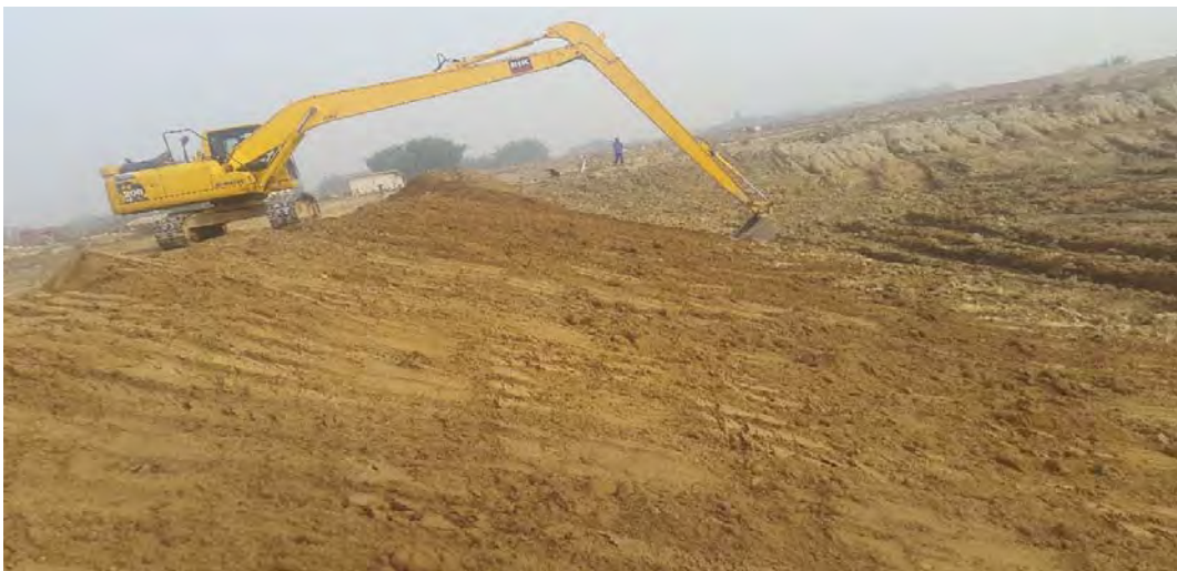
Picture 4 Slope preparation of anaerobic pond on WWTP.
