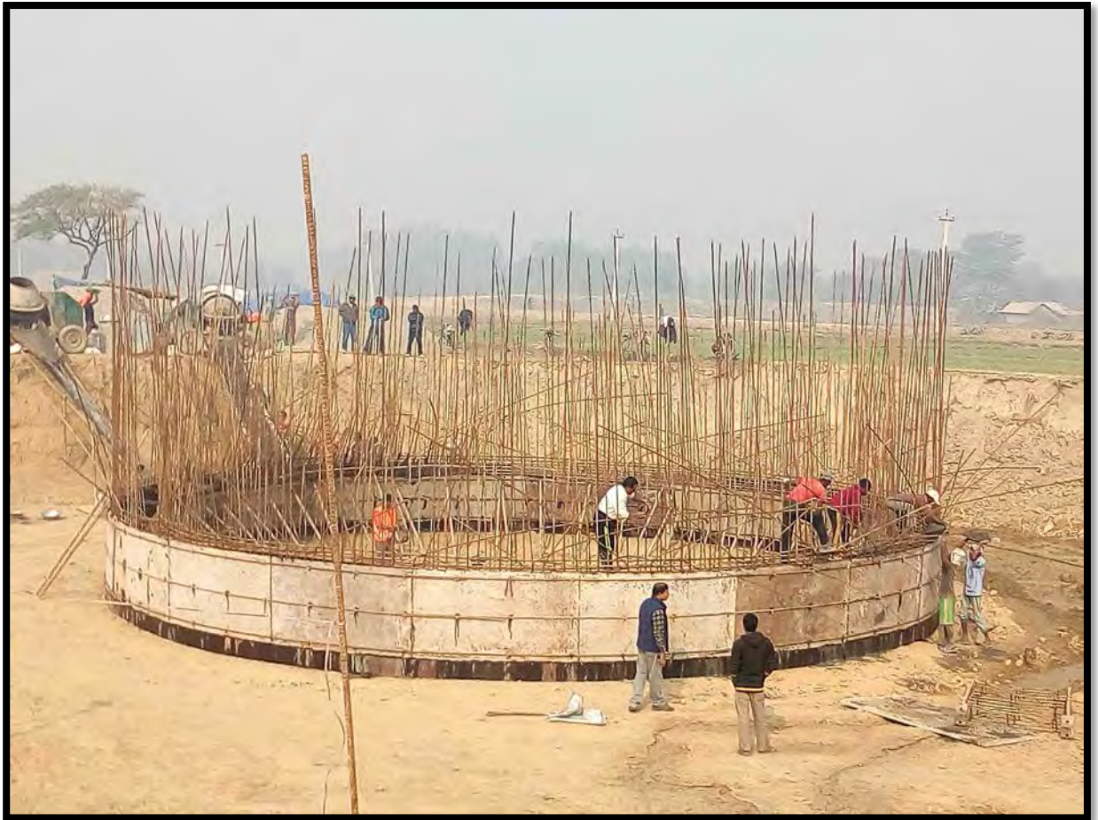
Concreting of Cutting edge at Sump Well
