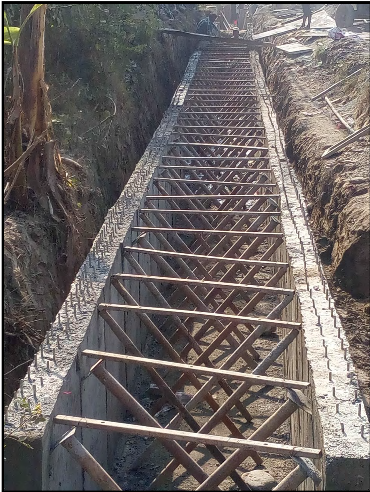
RCC road side drain at R3 road
