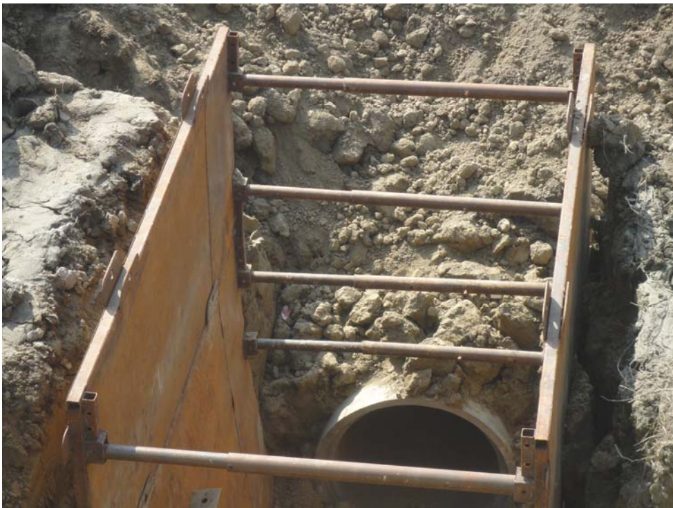
RCC pipe of Dia. 1,000 mm laid along T2 near WWTP, Jatuwa
