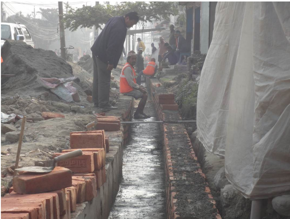
Brick Masonry Drain in progress at Pushpalal Road (R2)
