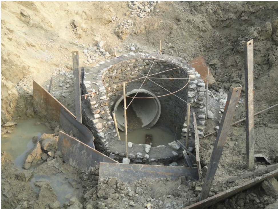
A Stone Masonry Manhole in Progress at S13 Storm Drain Site
