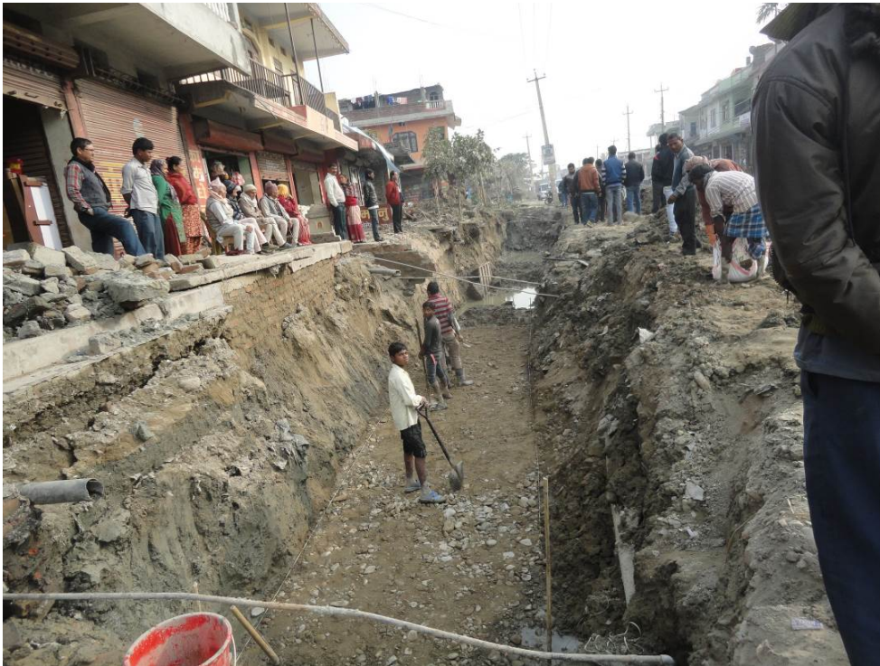
Foundation For Brick Masonry Drain at Pushpalal Chowk
