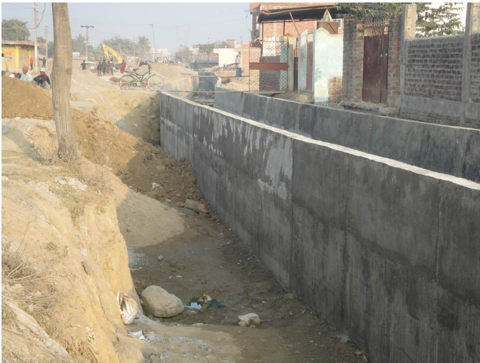
Back filling in progress at B3 Storm Drain
