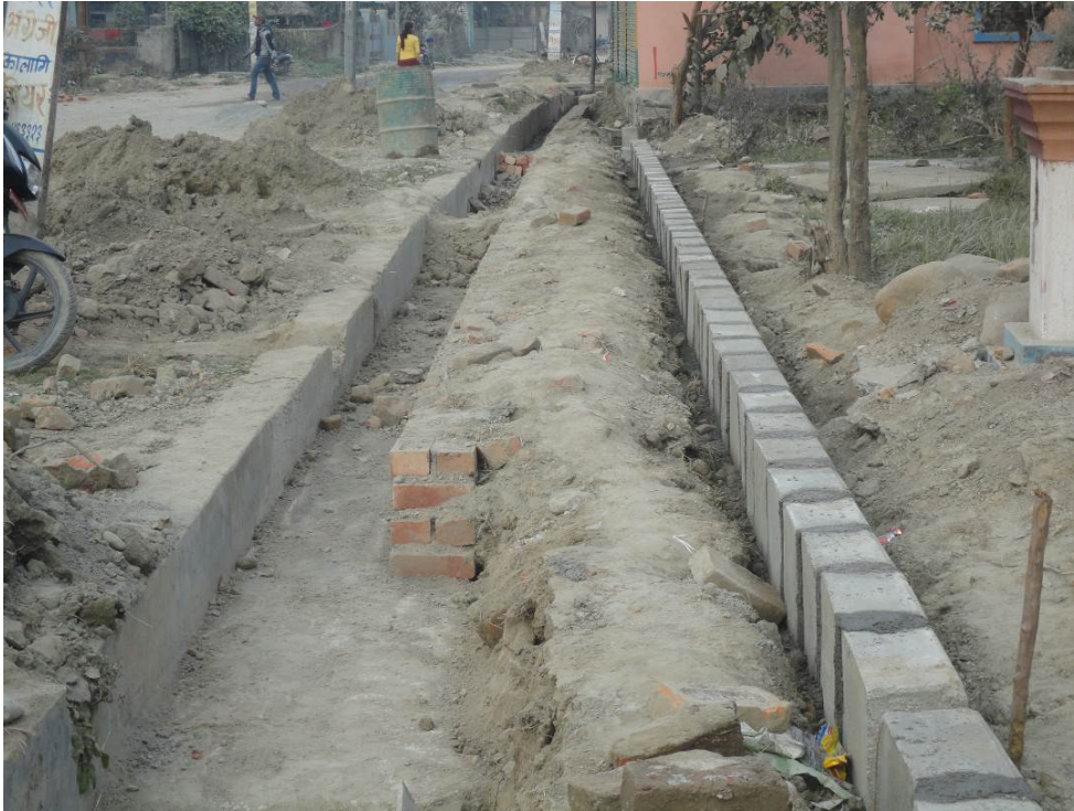
Placing of Kerbs for Footpath in progress at Pushpalal Road
