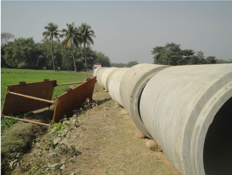
RCC pipe of Dia. 1,000 mm ready for installation along T2 near WWTP, Jatuwa
