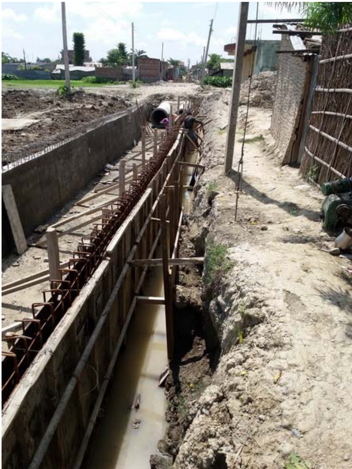
Figure 21 Drain and Hume pipe laying site B2
