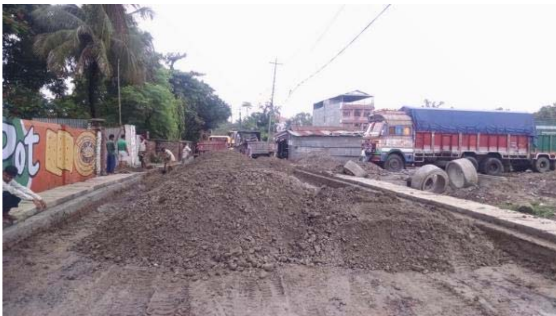
Figure 8 Sub base laying at Road R5 (Satghumti)
