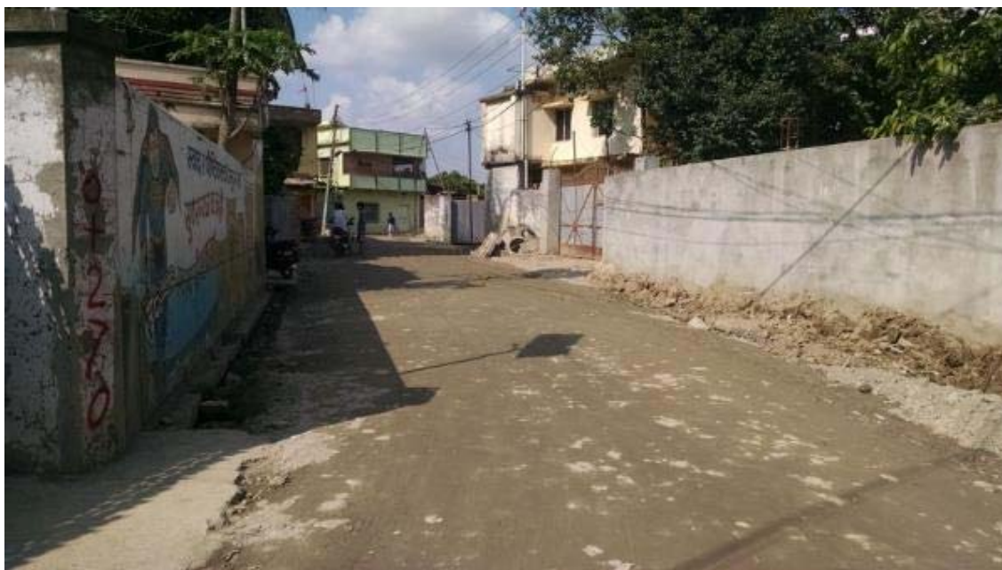
Figure 23 Sub base completed road section road R65 (Satghumti)
