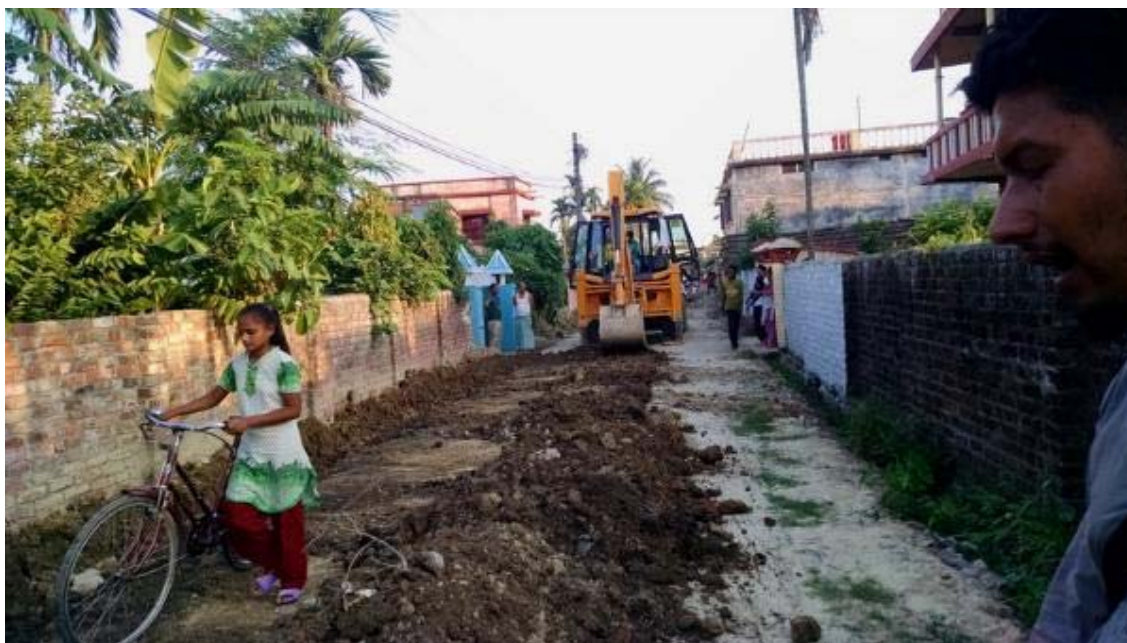
Figure 22 Backfilling at secondary line 13F
