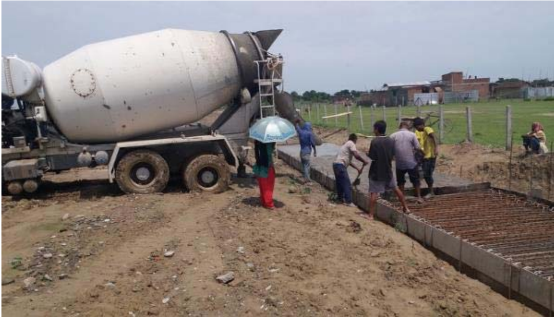
Figure 26 Concreting at drain B2
