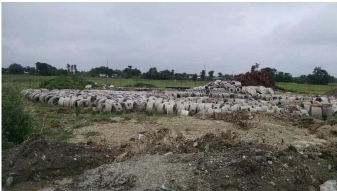
Figure 2 Stock precast Chambers at Yard
