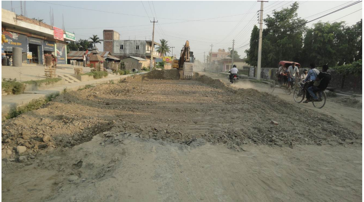
Scarification of Existing Road Surface of R2 (Pushpalal) Road for Sub-grade Preparation
