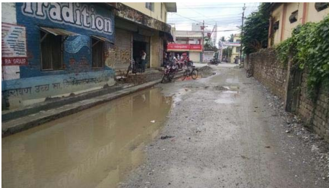
Figure 7 Completed drain and sub base road inundated due to lack of outfall at R65
