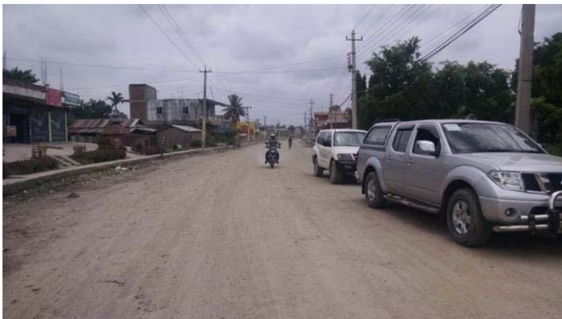
Figure 13 R2 road sub base completed section
