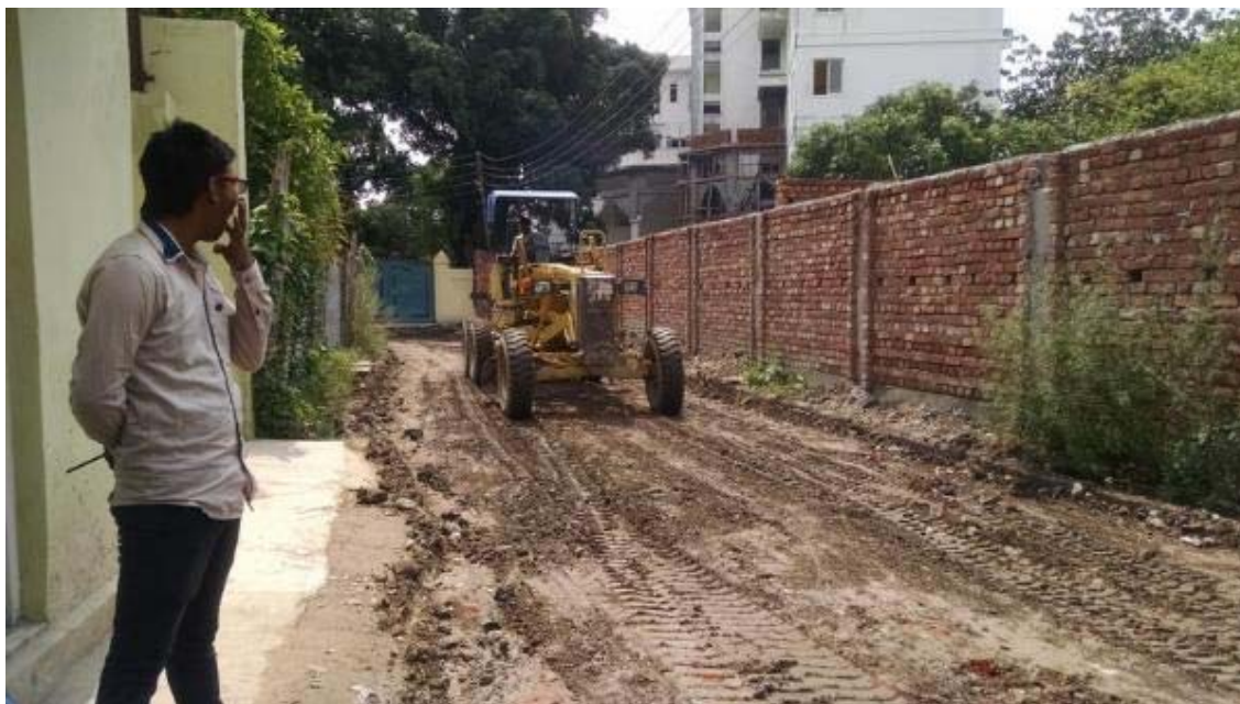
Figure 25 Subgrade preparation at Road R65
