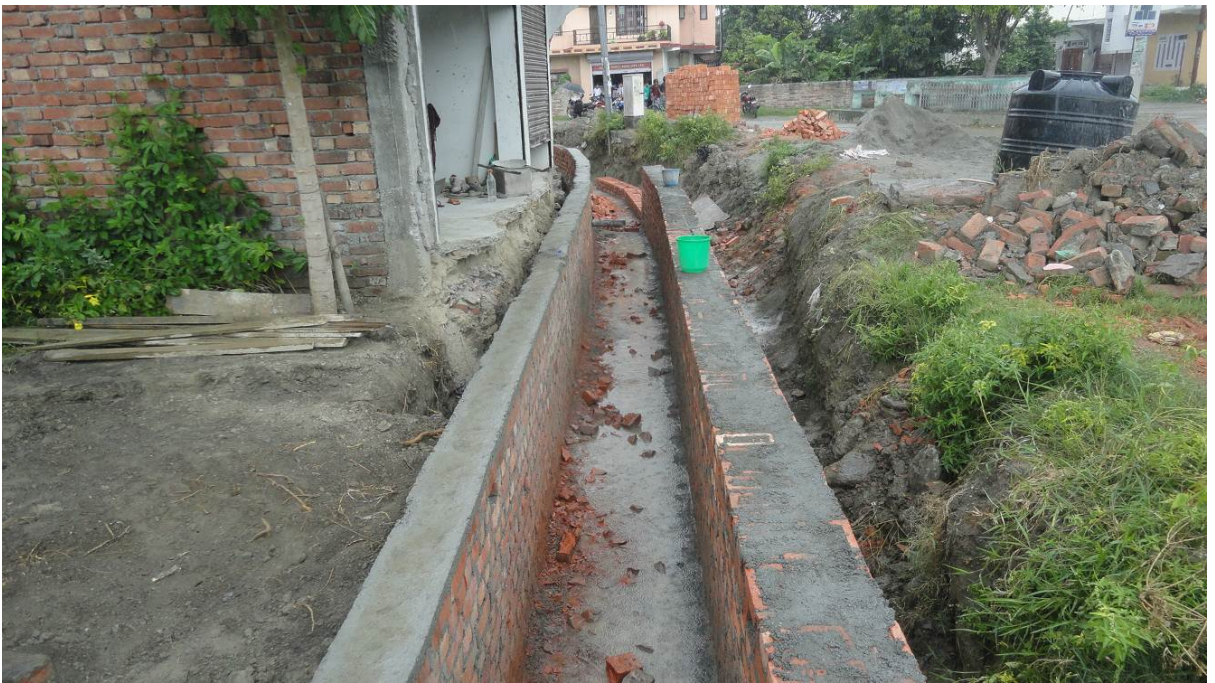
Brick Masonry Drain at Radha Krishna Chowk,B2
