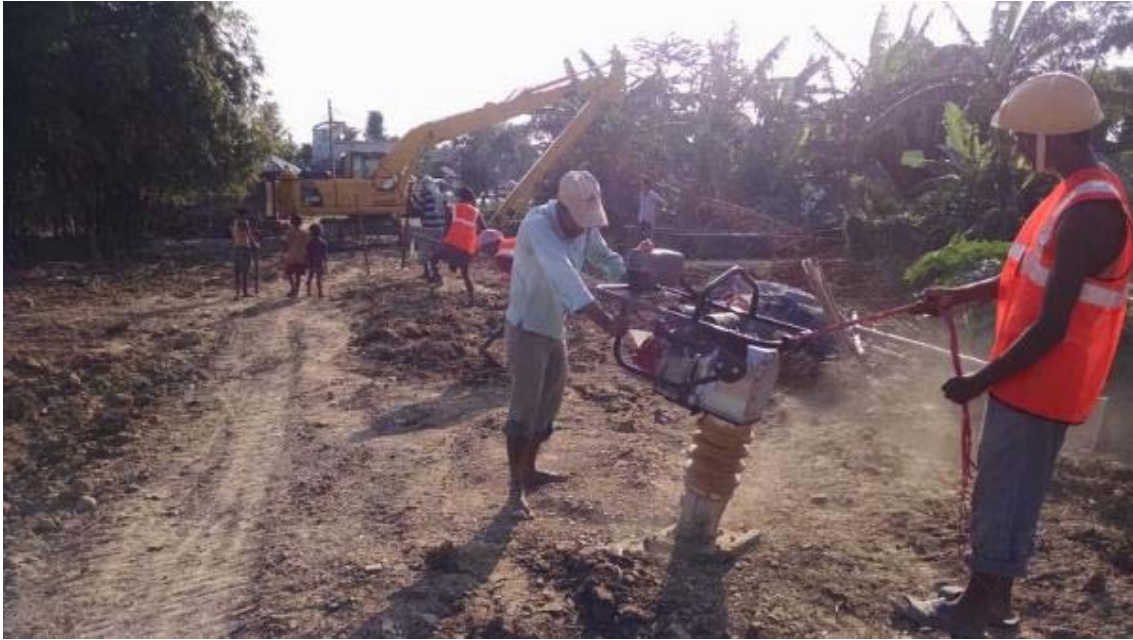
Figure 19 Backfilling and compaction at Hume pipe laying site T2 Trunk
