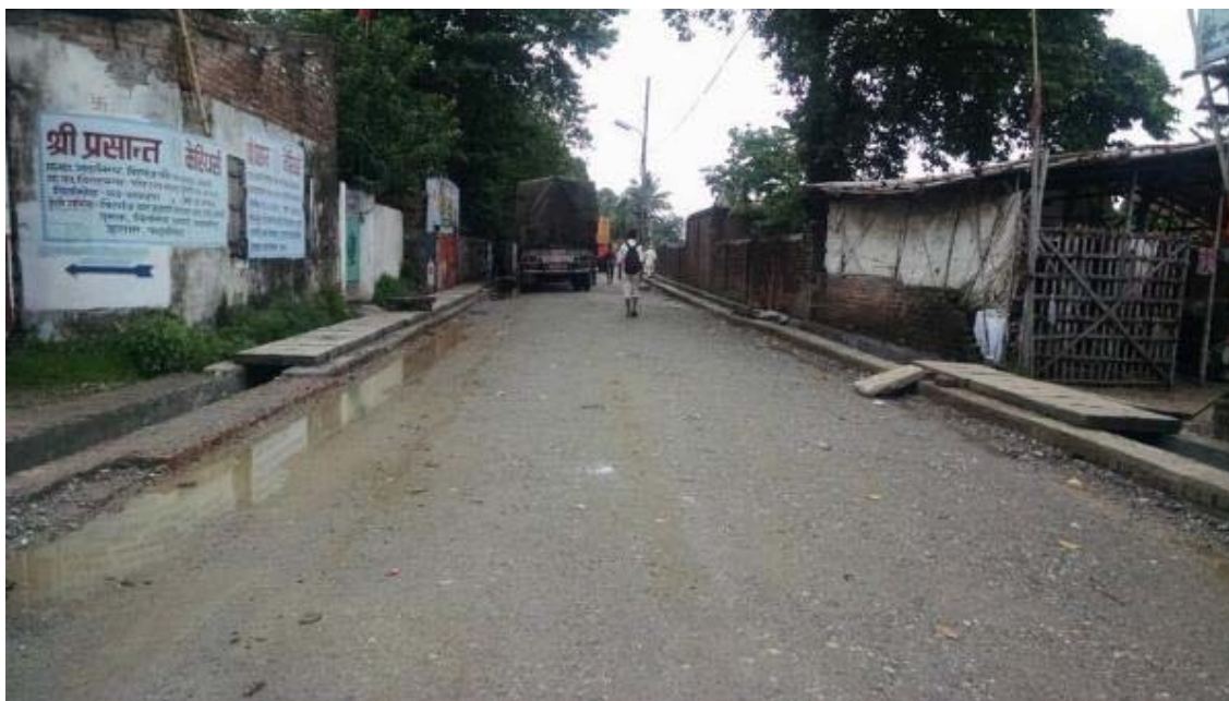
Figure 9 Sub base completed road section of R5
