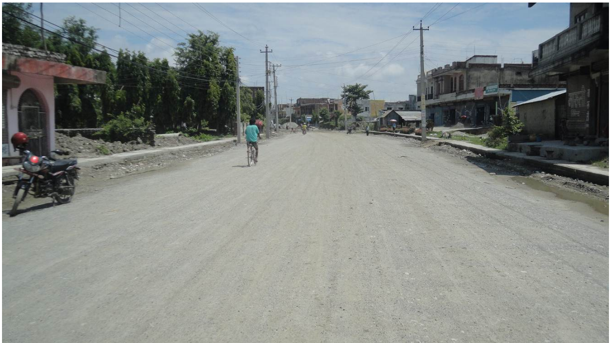
Sub-base prepared in a 100 m length at R2 Road
