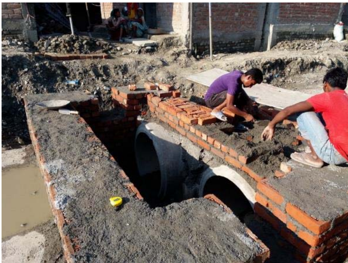
Figure 16 Manhole construction at Line B2
