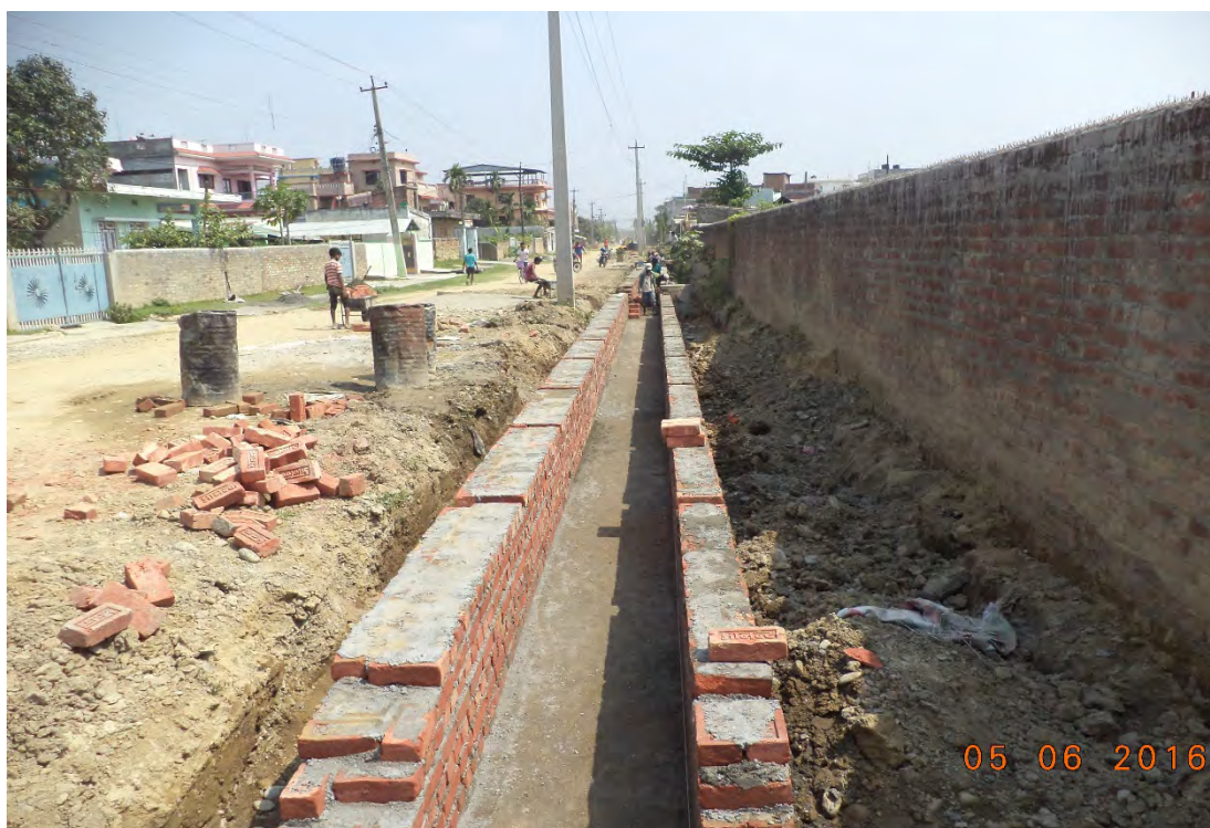
Road side drain Construction at R3 Road
