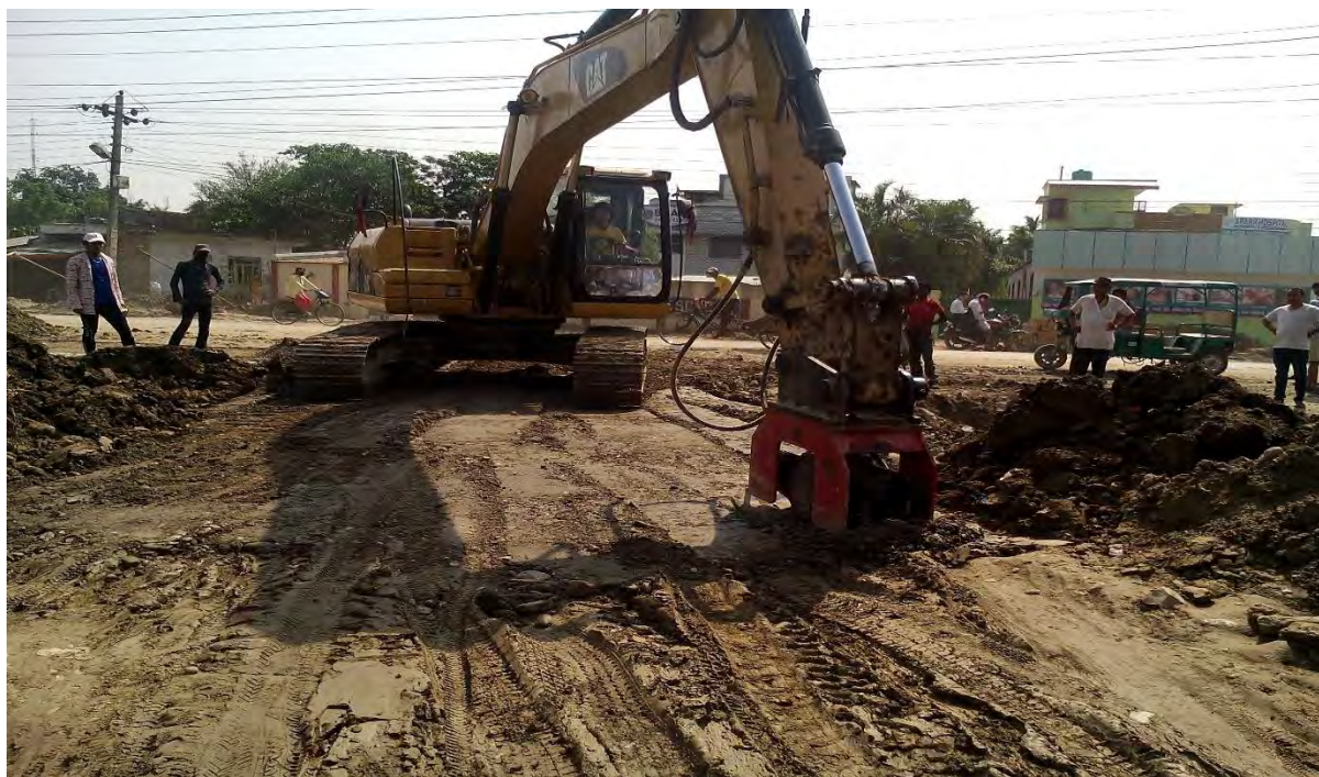
Figure 2 Compaction at Highway.|
