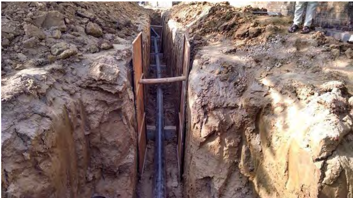
Figure 6 Shoring at HDPE pipe laying.
