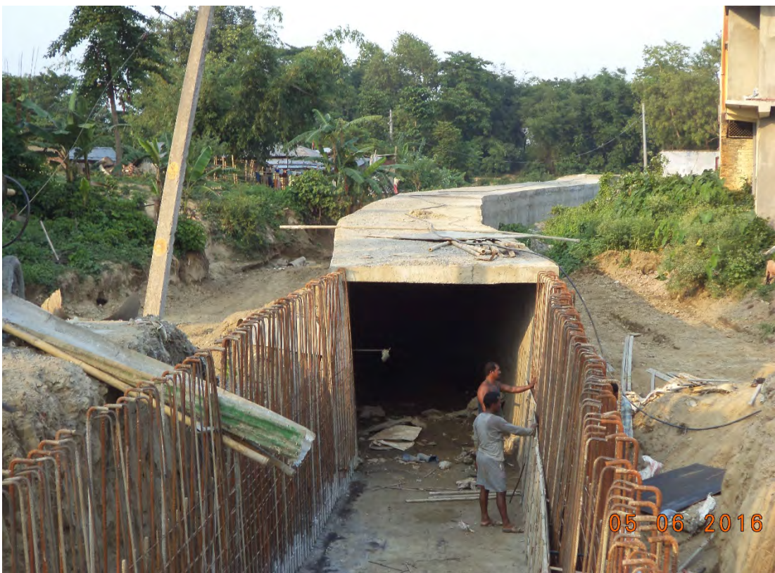
RCC Storm Water drain at S9
