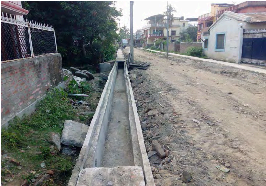
RCC Road side drain at R27 Road
