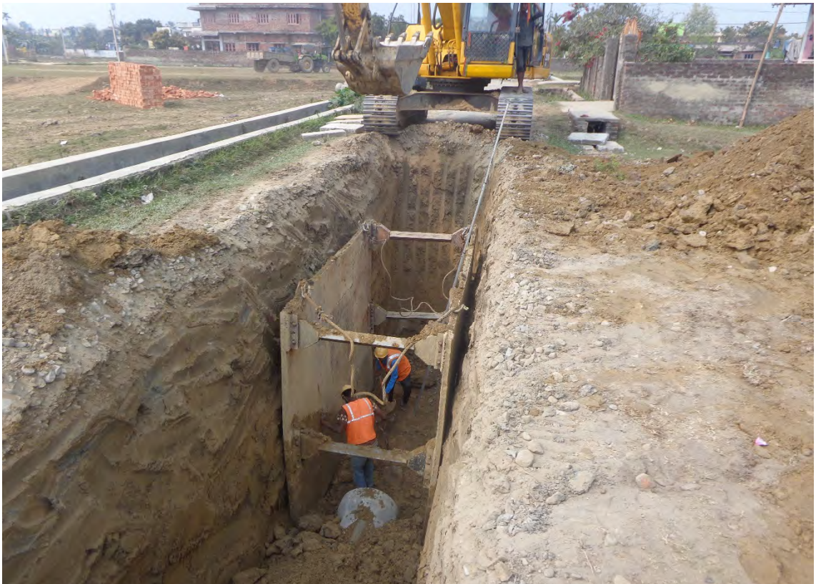
Hume pipe laying in sewer line
