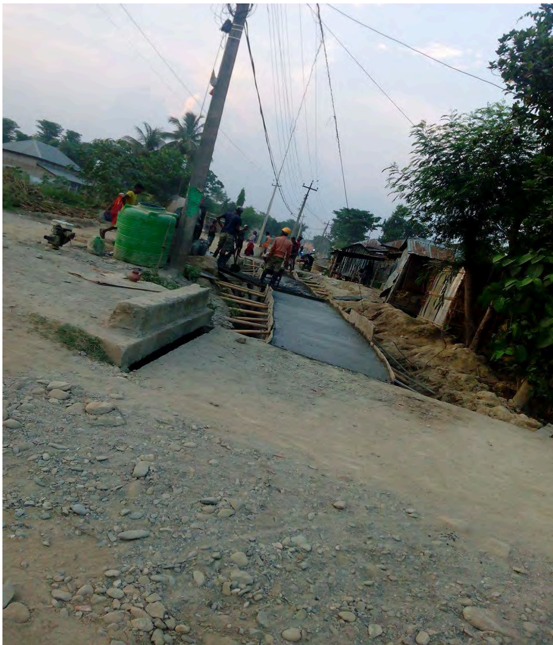
Drain cover Slab casting at R3 Road
