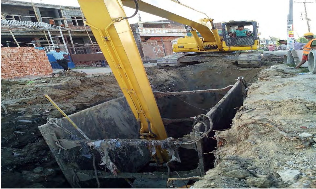
Figure 5 Shoring works at hume pipe laying.
