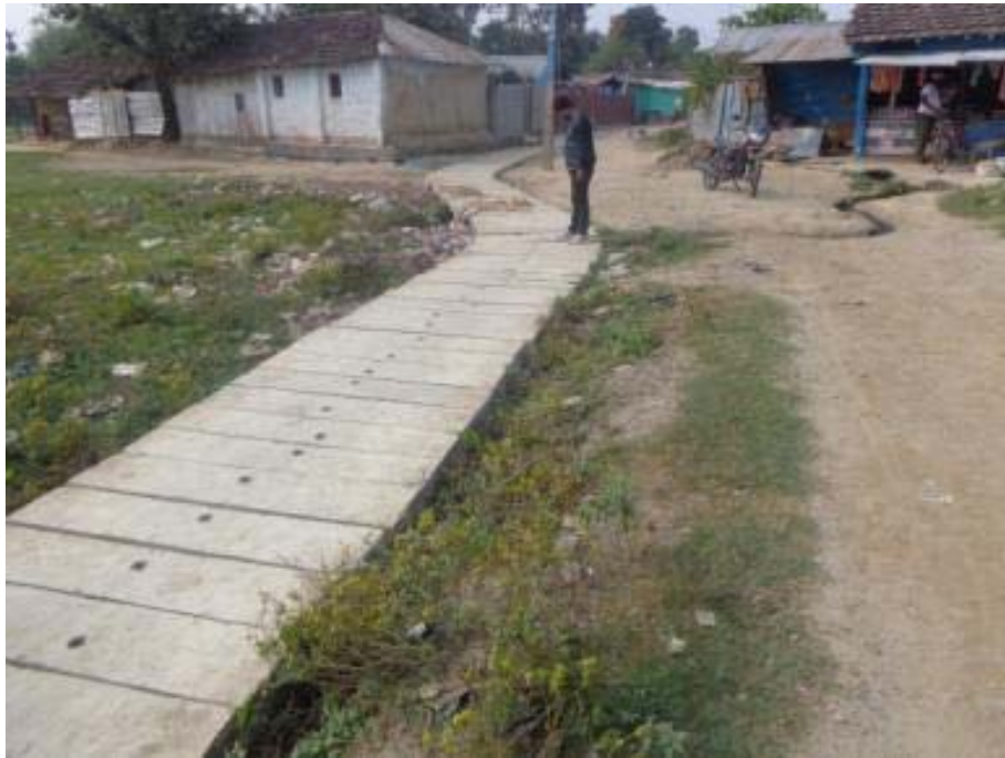
Completed Storm Drain at Pawan Marg (Rani), Southern Drainage System
