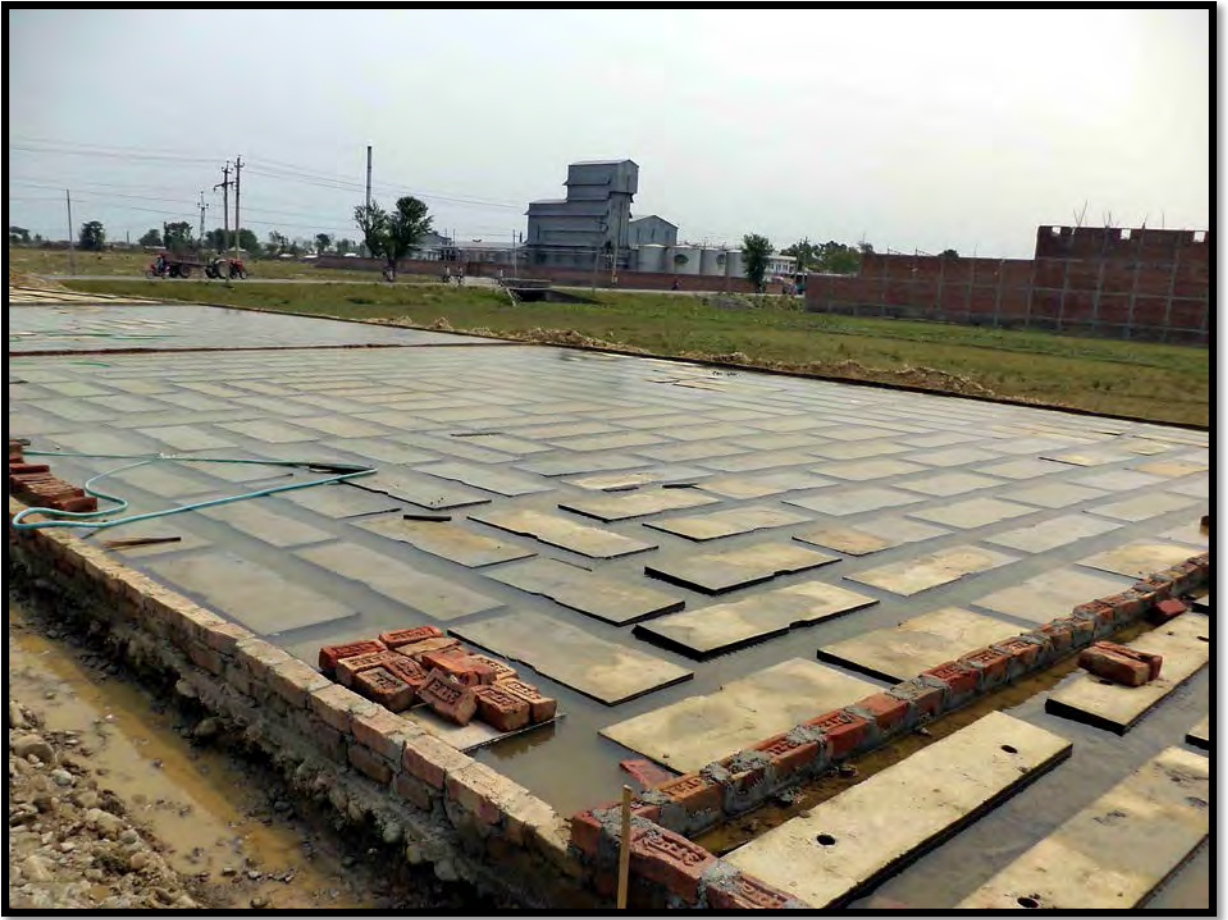
Precast Drain Cover Slab production at Contractor's yard
