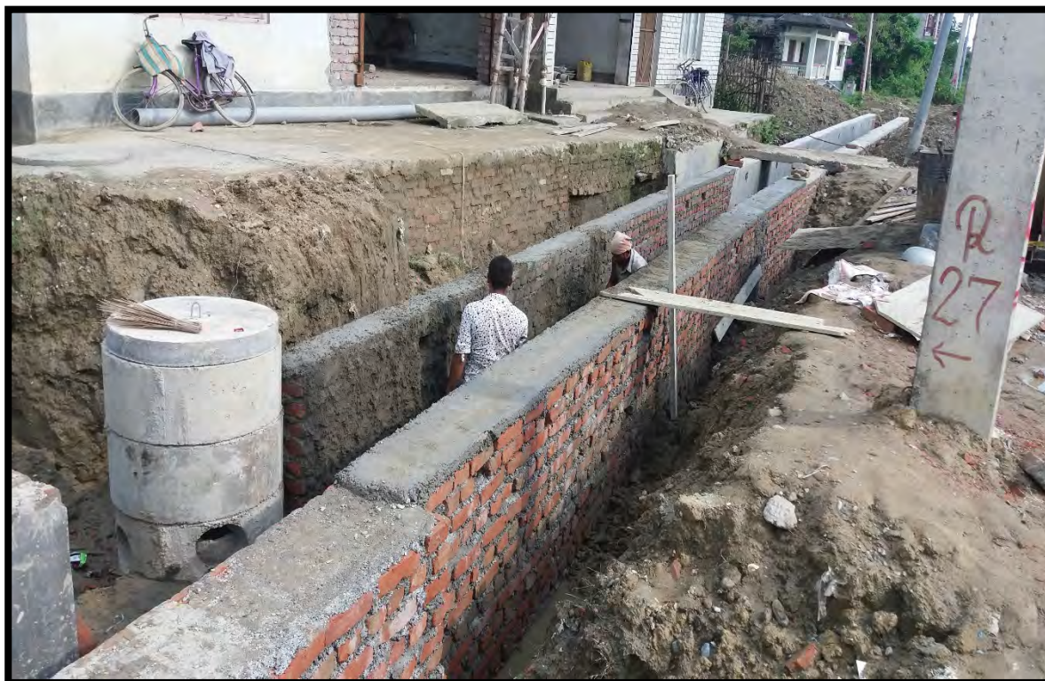
Road Side Drain at R3 (Dharambandh)
