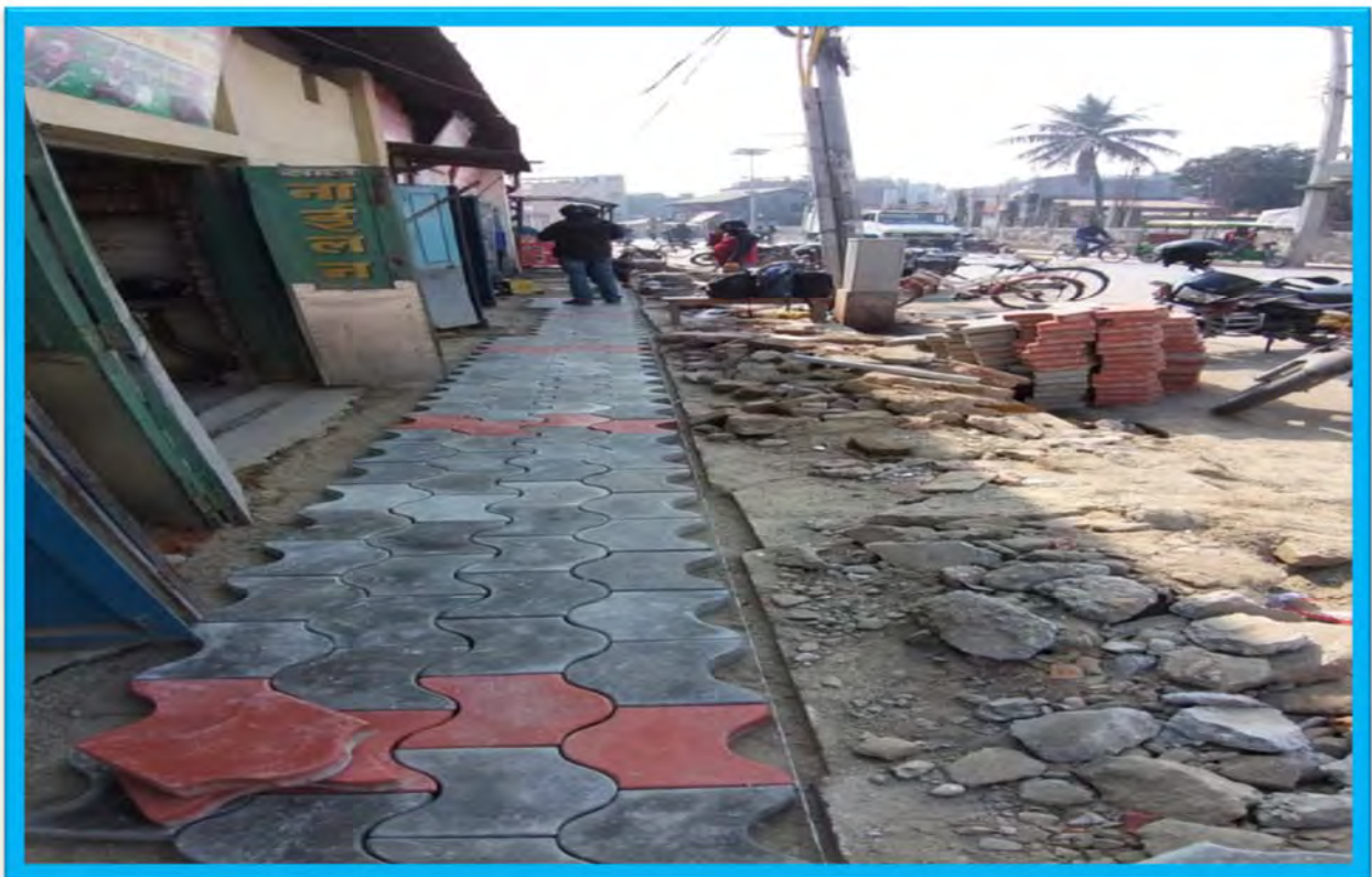
Interlock work at Devkota chowk East
