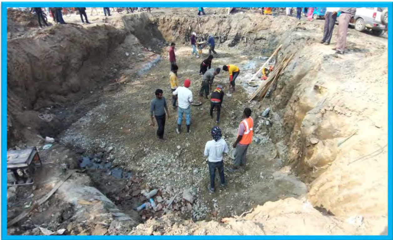
Soling work for culvert at Keshaliya Road
