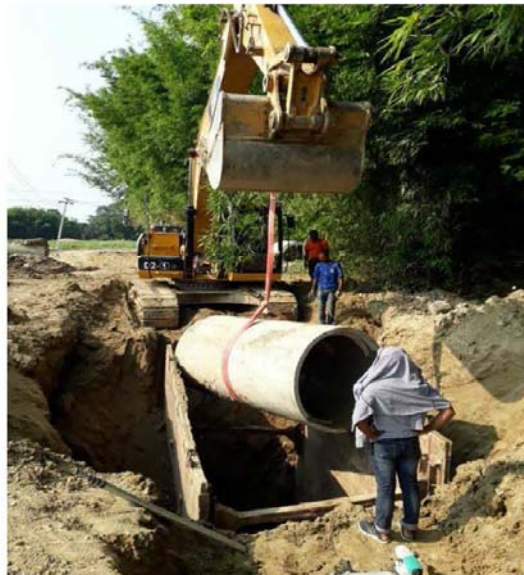
Laying of Hume pipe
