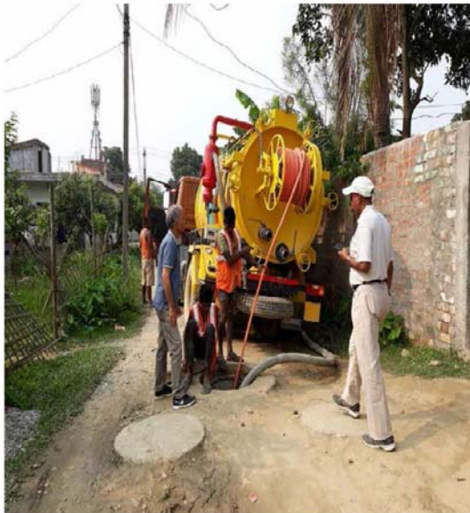
Sewer cleaning work using jetting machine
