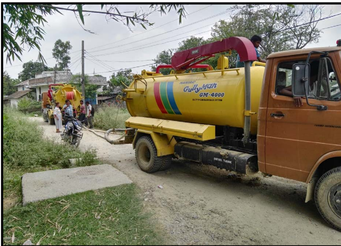
Manhole cleansing work of sewer line in R4 (T2 Line)
