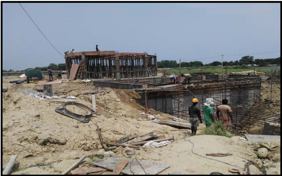
A view of Sump well and enclosure chamber at WWTP
