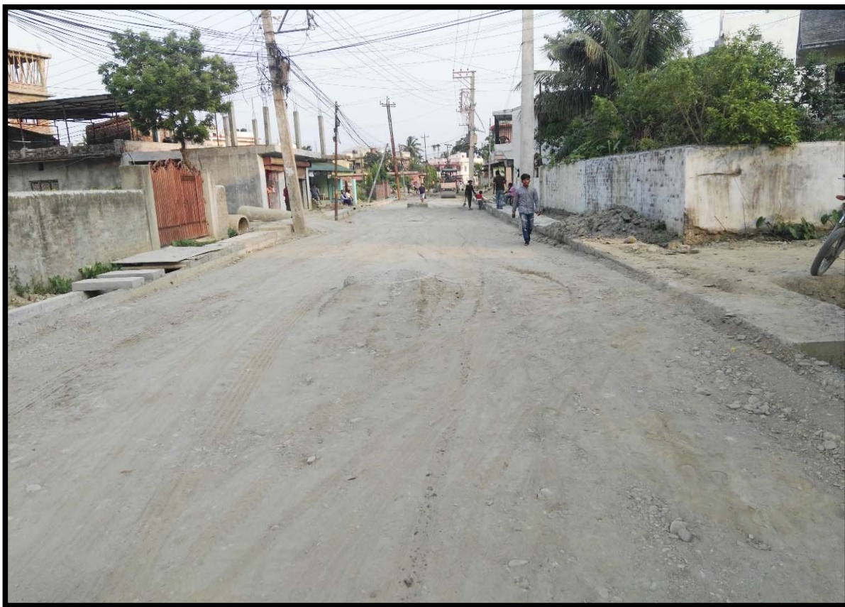
A view of R6 Lane (Shahi Marg) after sub base laid
