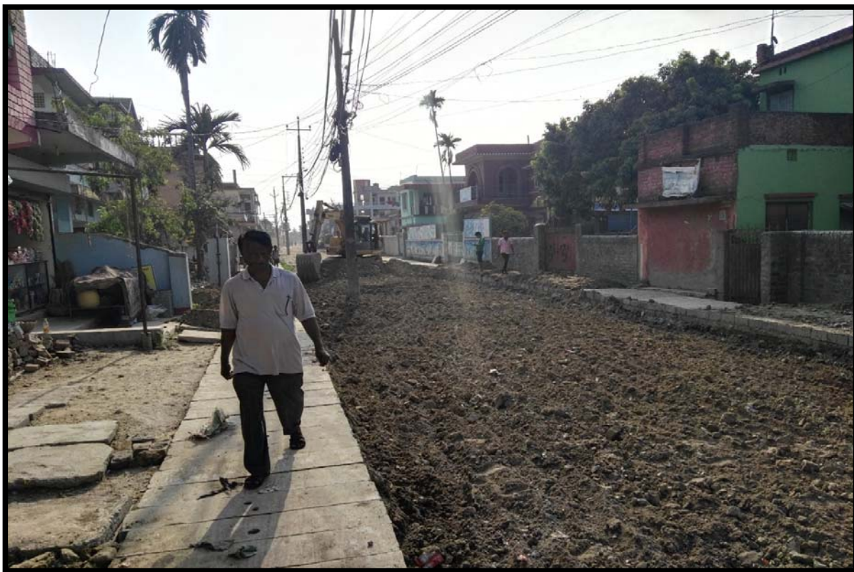
Sub grade preparation work in R29
