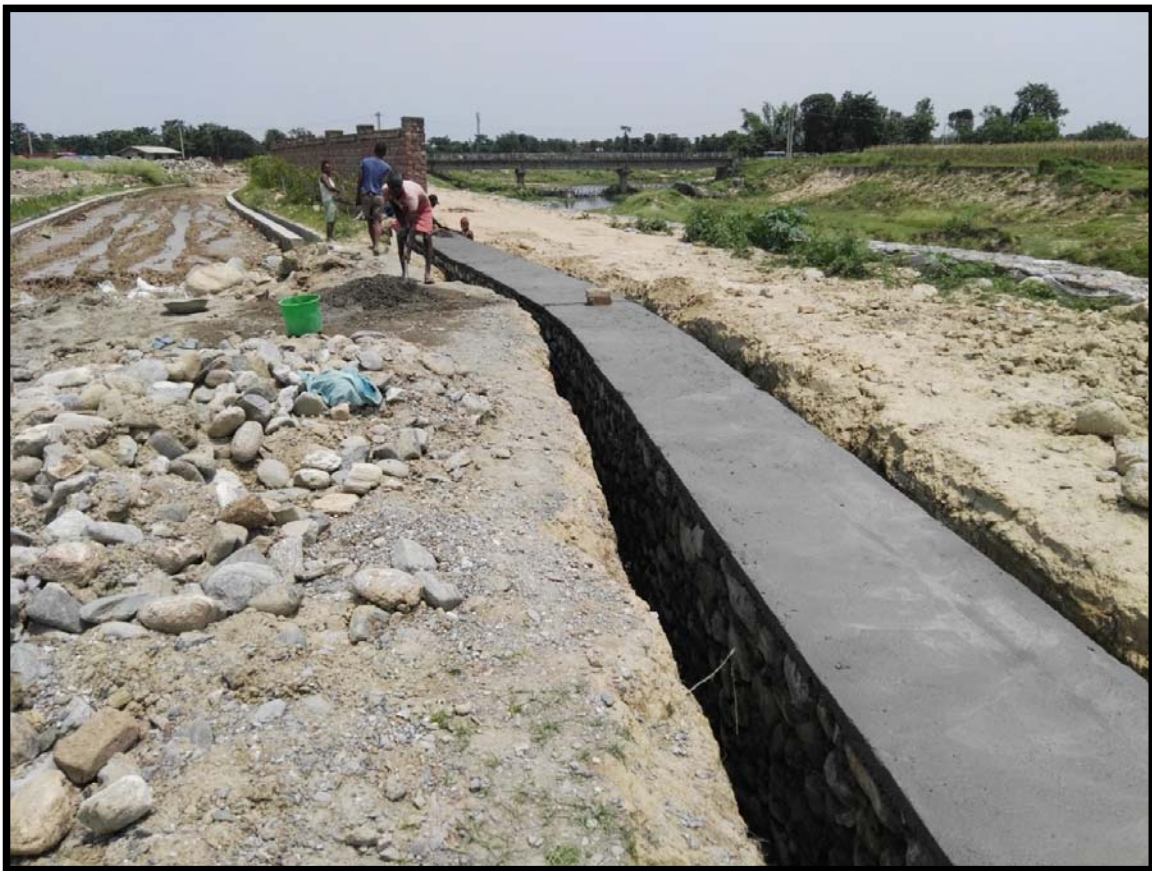
Reconstruction of boundary wall fallen down during flood last year at WWTP
