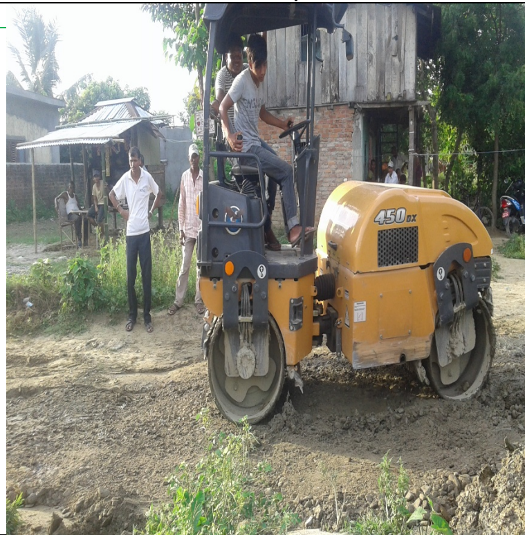
Compaction of subbase
