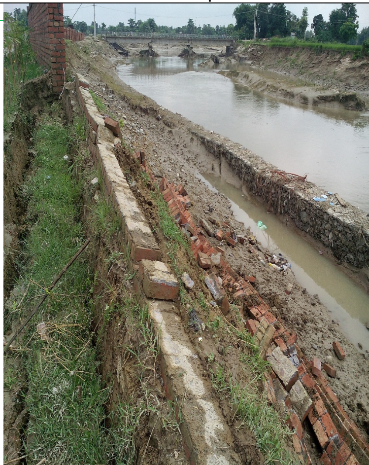
Broken wall at WWTP due of flood
