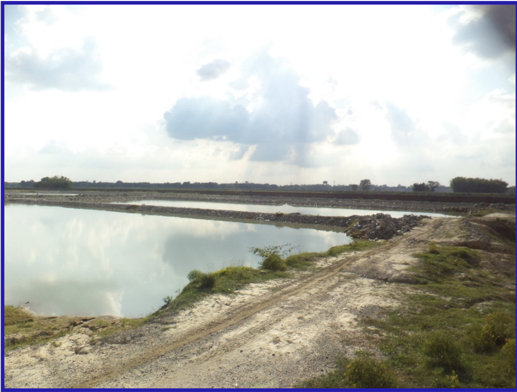
Anaerobic pond at WWTP
