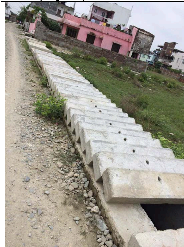
Placing Slabs over drain
