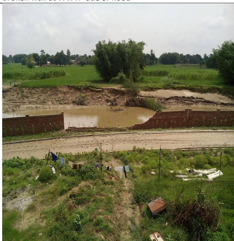
Effect of flood in WWTP wall
