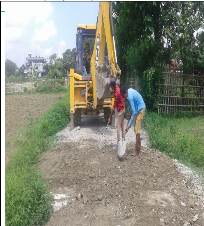
Laying of subbase
