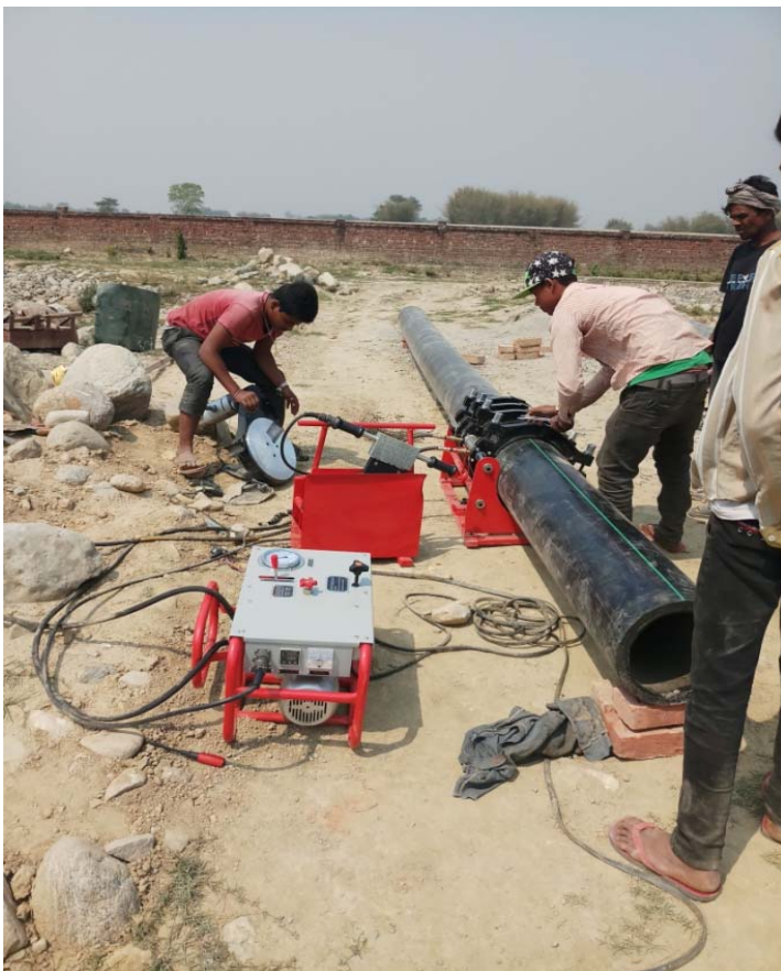
300 Diameter HDPE Pipe Laying in WWTP
