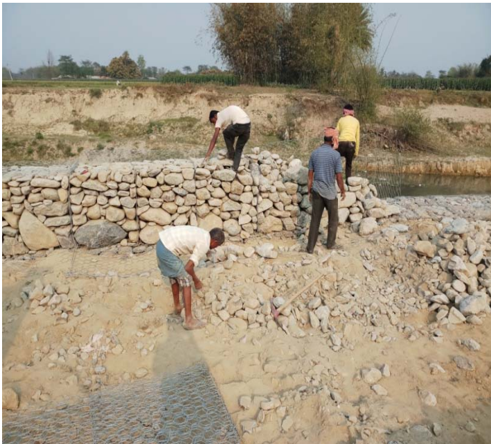
Gabion Work in WWTP
