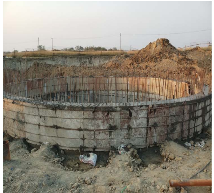
Shear Wall Concreting in Sump well
