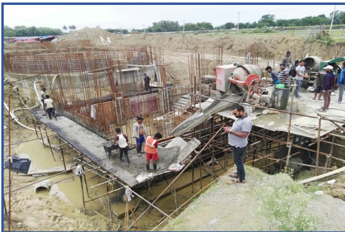
Enclosure Chamber shear wall and stair concreting
