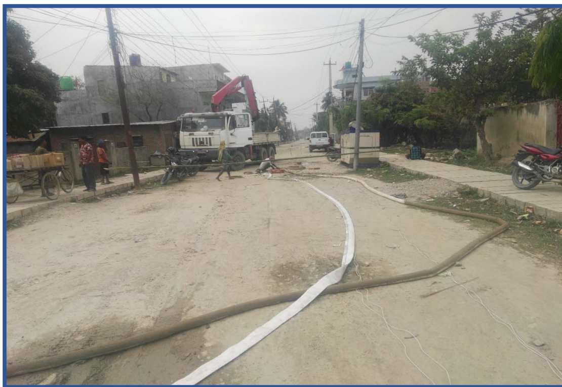
Dewatering and cleansing of sewer manhole
