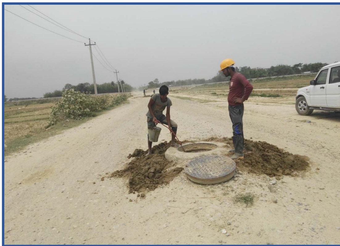
Cleansing of sewer manholes
