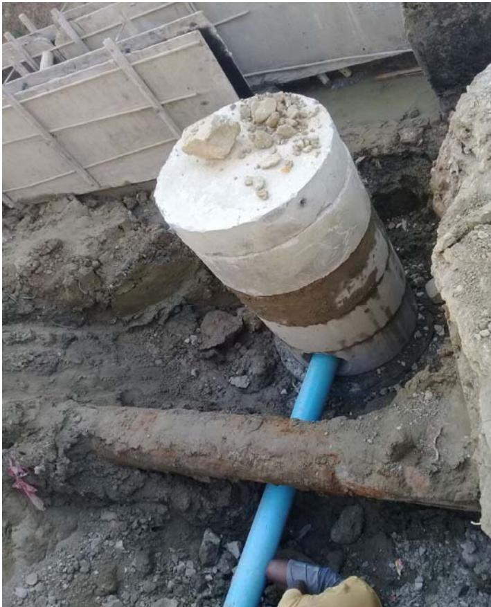
Sewer Inlet Installation
