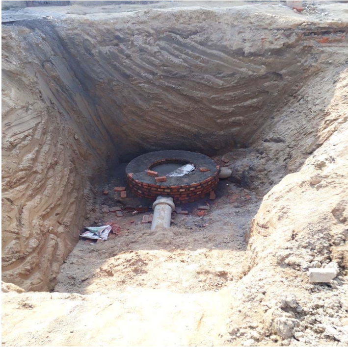
Brick Manhole Work
