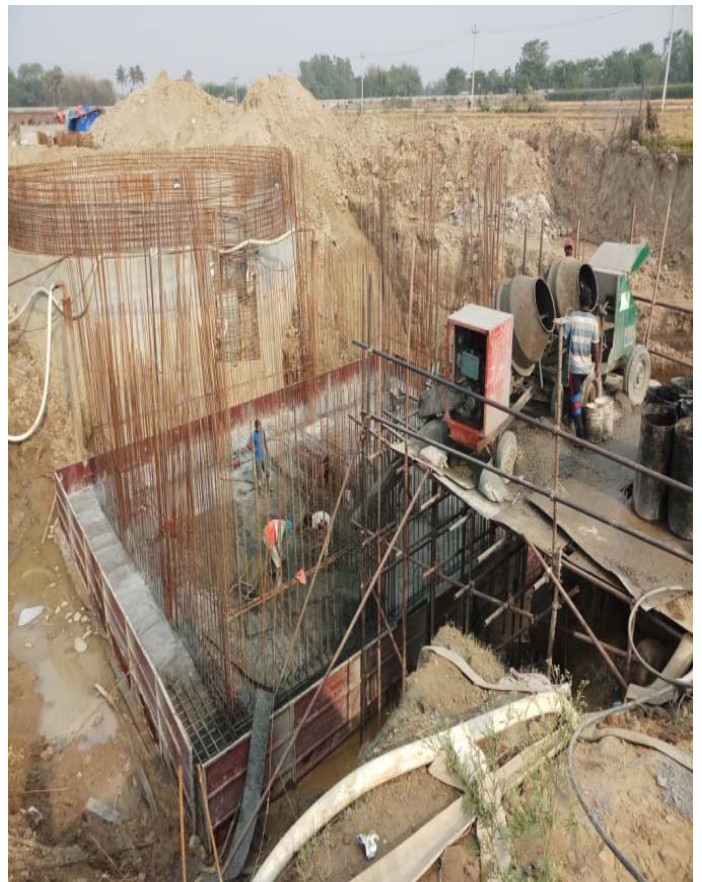
Raft Concreting in Enclosure Chamber
