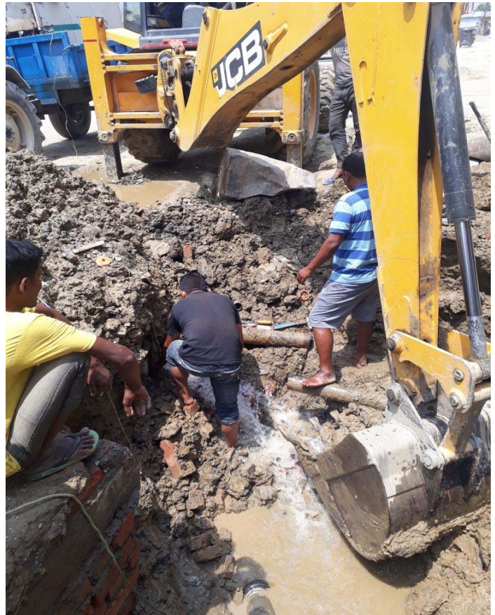
Drinking Water Pipe Maintenance
