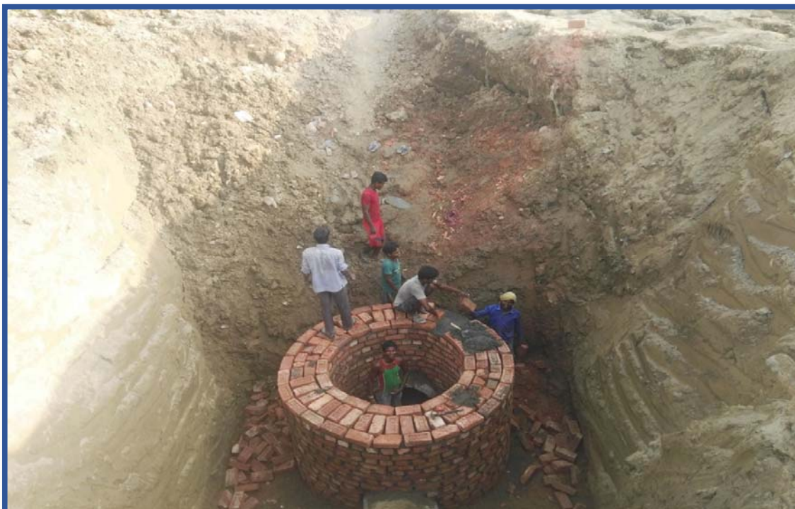
Repair of Sewer line pipe settled in R3 Lane
