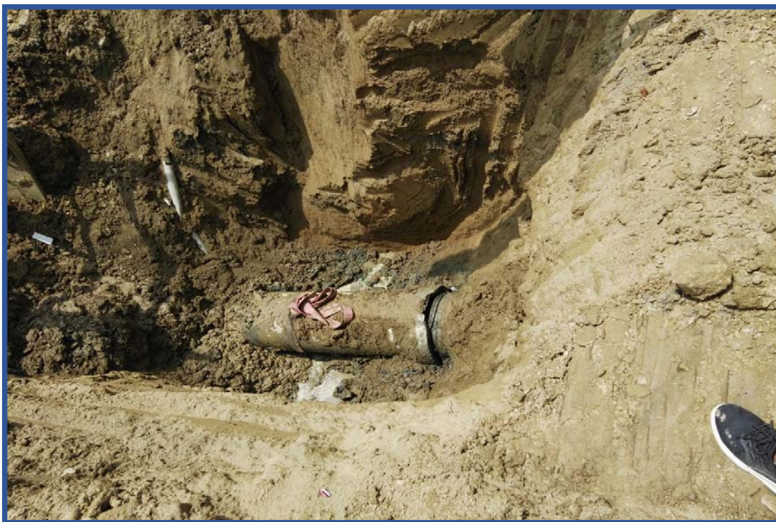
Sewer line pipe settlement in R3 Lane
