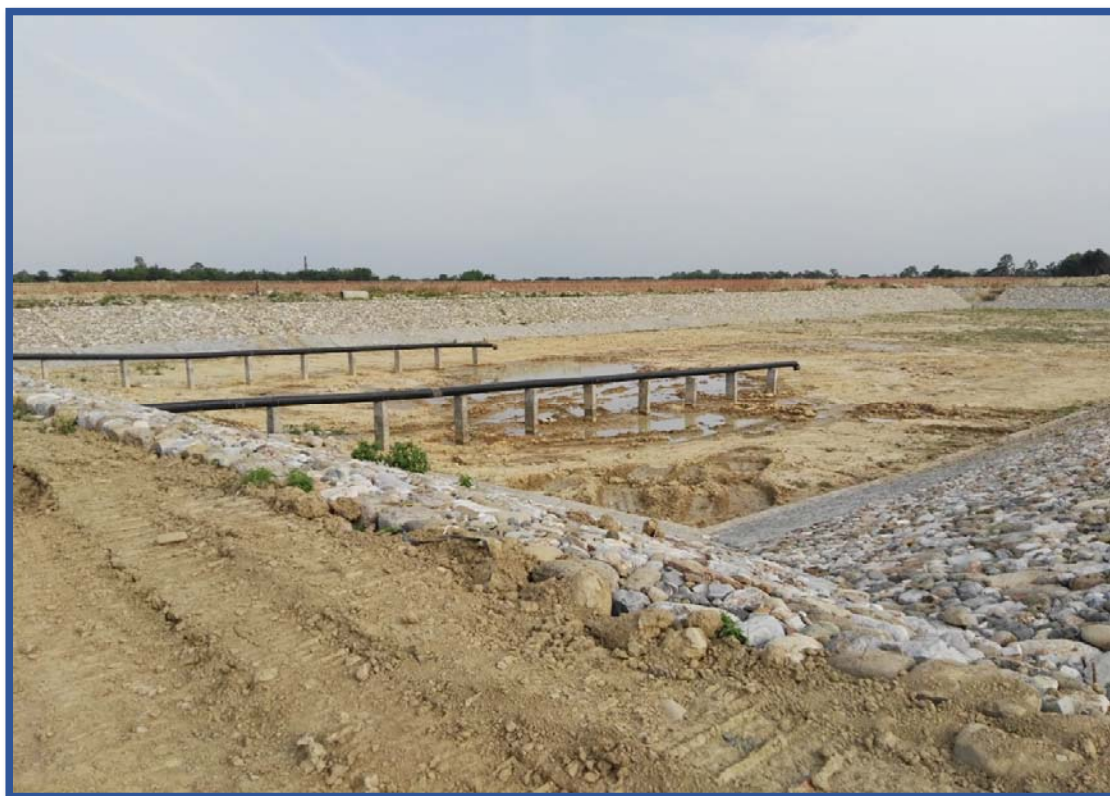
Pipe Laying in facultative pond
