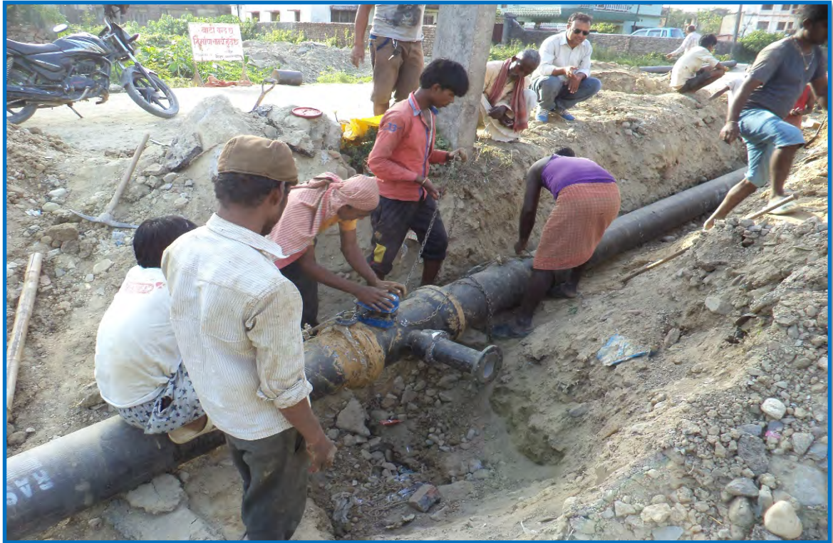
DI Pipe of Water Supply at R6 Road
