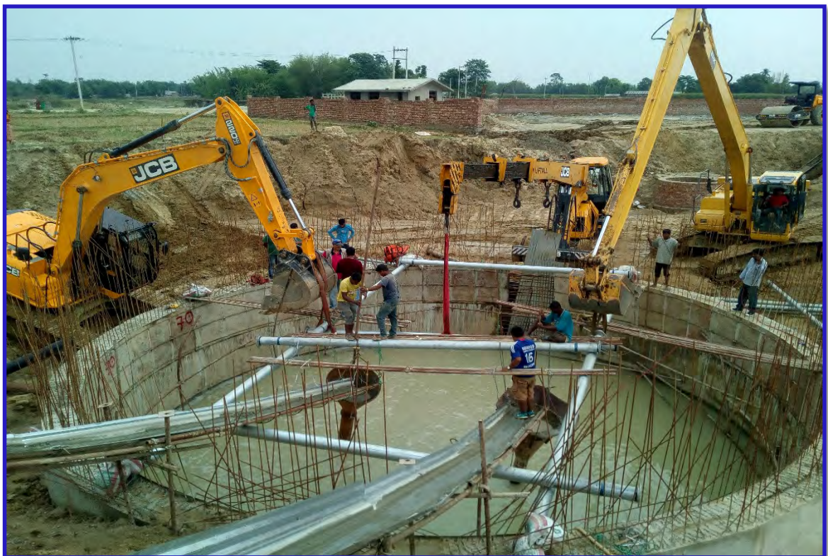
A view of Sump Well concreting in Bottom Plug underneath of water
