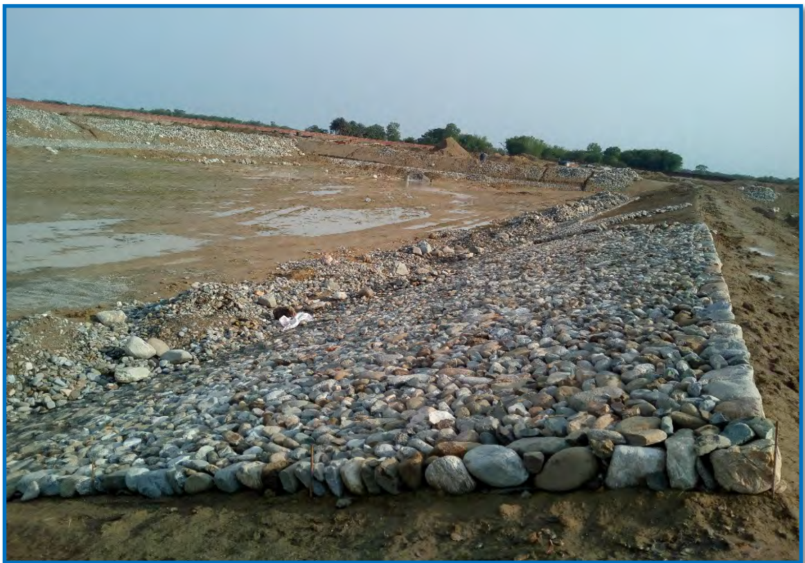
Rip Rap masonry work at WWTP
