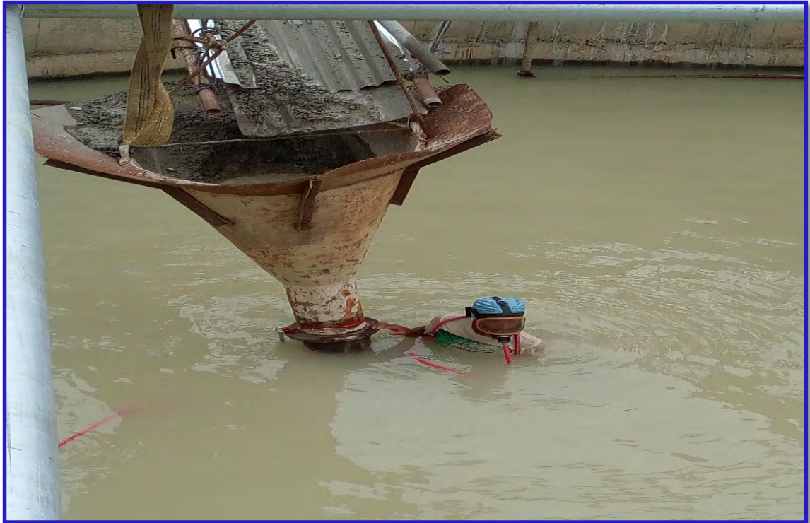
Concrete of Sump Well's bottom plug at WWTP
