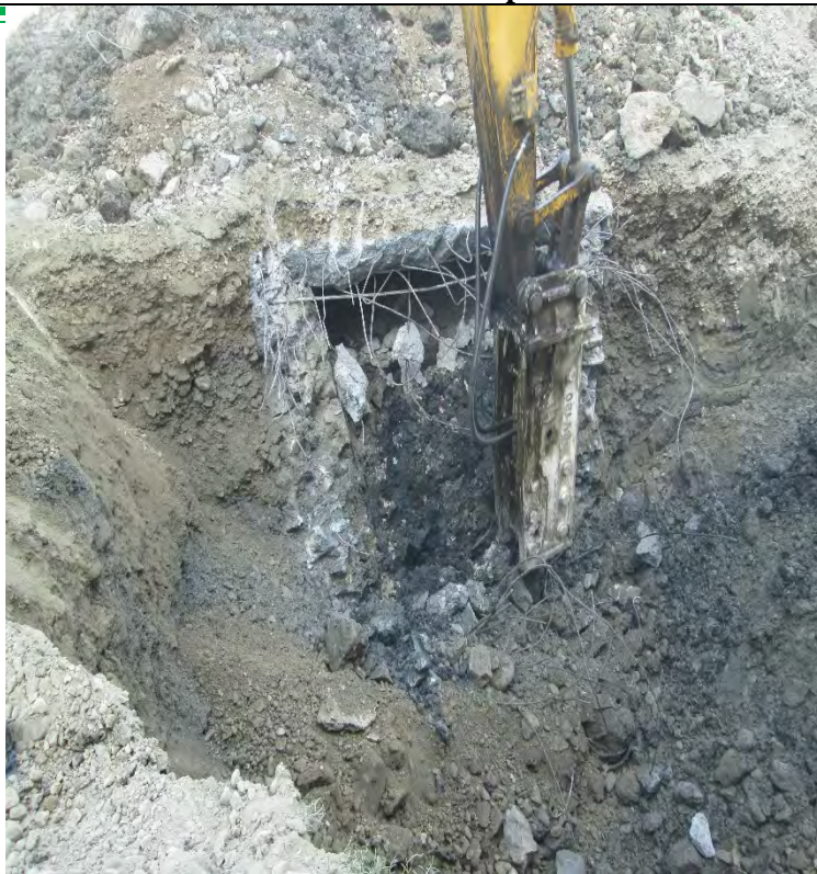
Using Breaker to Dismantle Box Culvert at T1 Trunc
