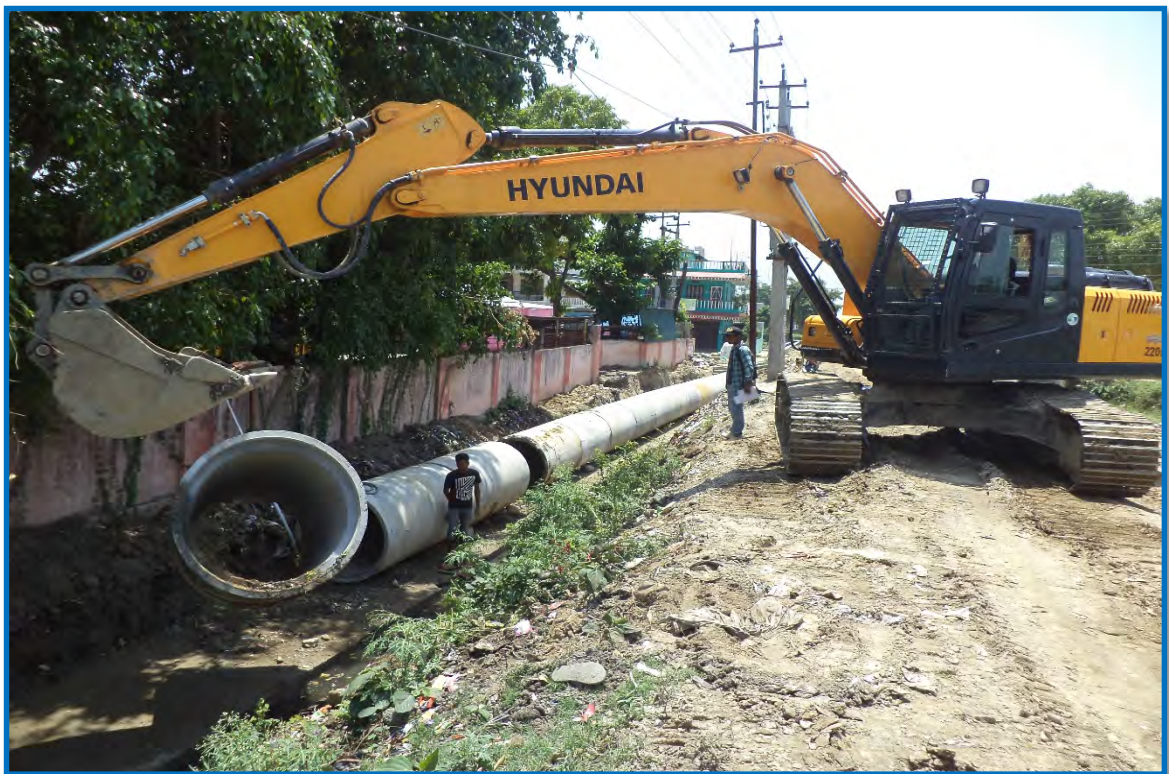
Storm Water Drain at CN3L1A stretch
