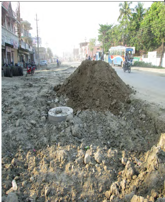
Backfilling Work in Highway T1 Trunc
