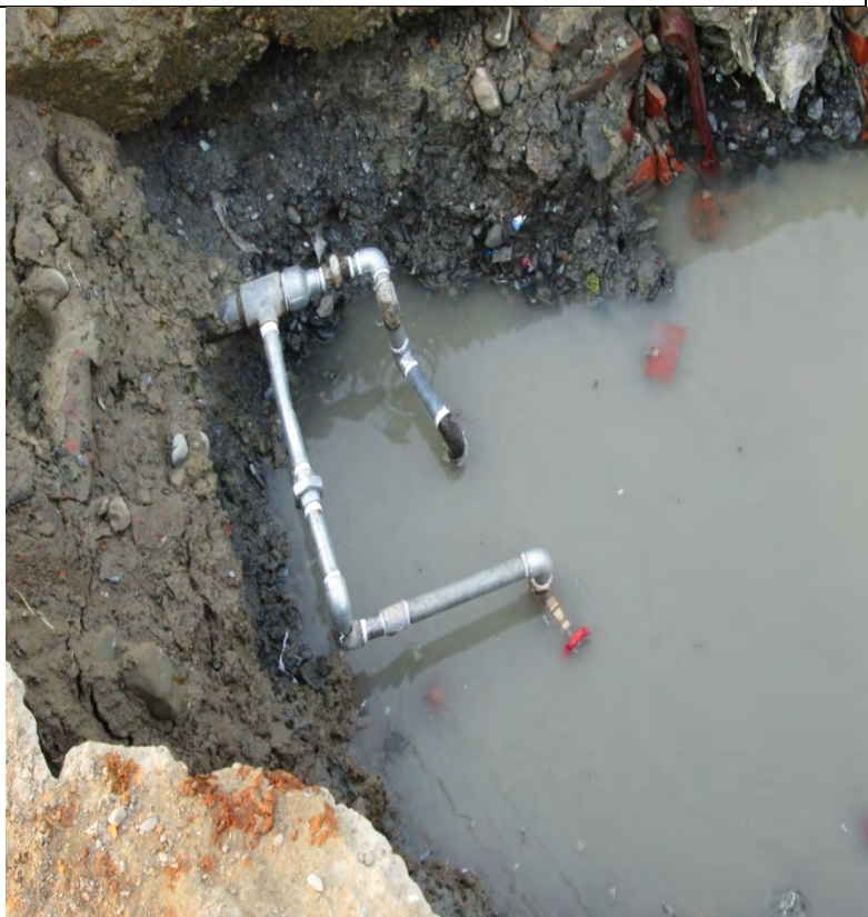
Maintainence of Drinking Water Pipe in T1 Trunc
