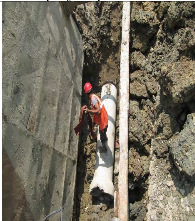
Hume Pipe laying at Koshi Highway (Trunk line)
