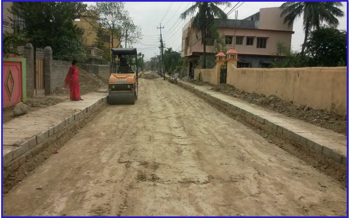
Subgrade preparation at R29 road
