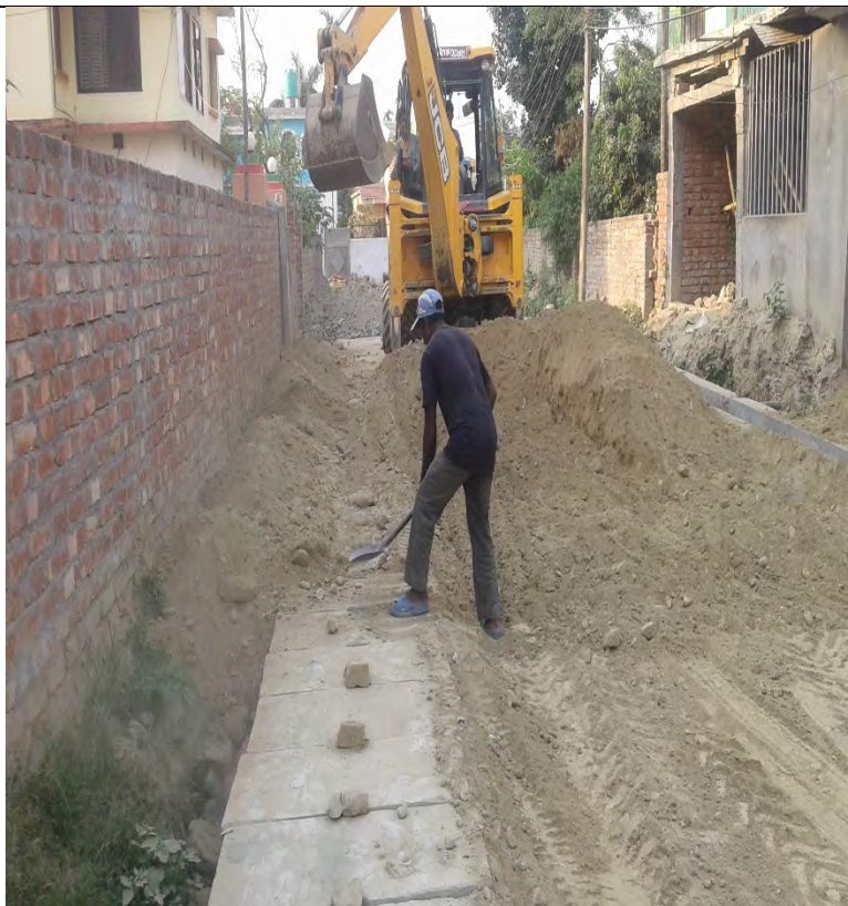
Backfilling work in road side drain under progress
