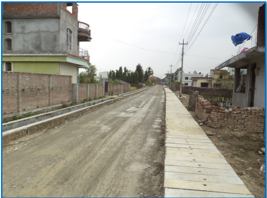
Sub base finishing at R21
