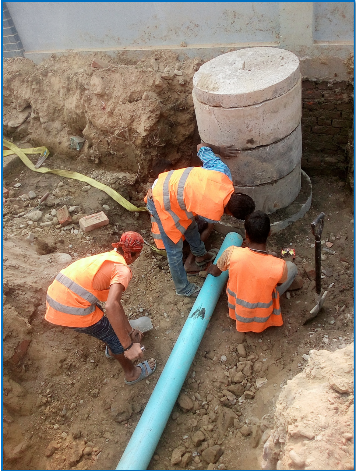
Sewer Inlet Connection at R9 Road
