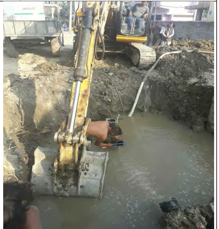
Maintenance of Drinking Water Pipe in T1 Trunc
