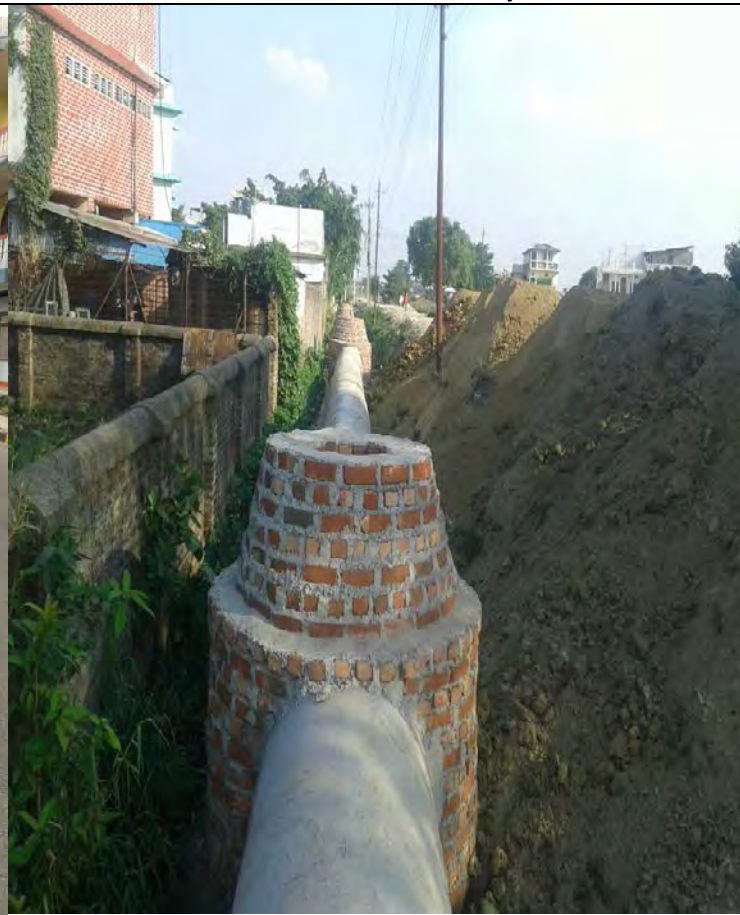
1000mm dia hume pipe laying at CN3L1A
