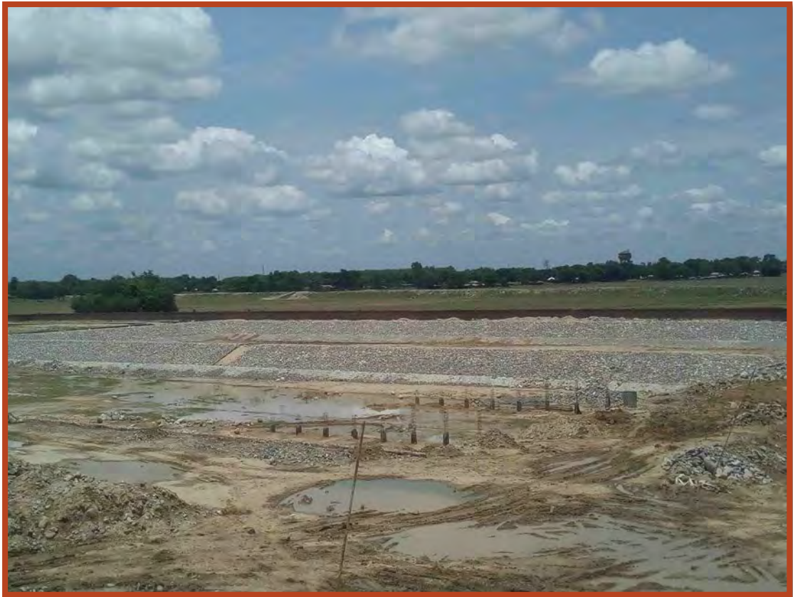
Rip Rap work at WWTP for Facultative pond
