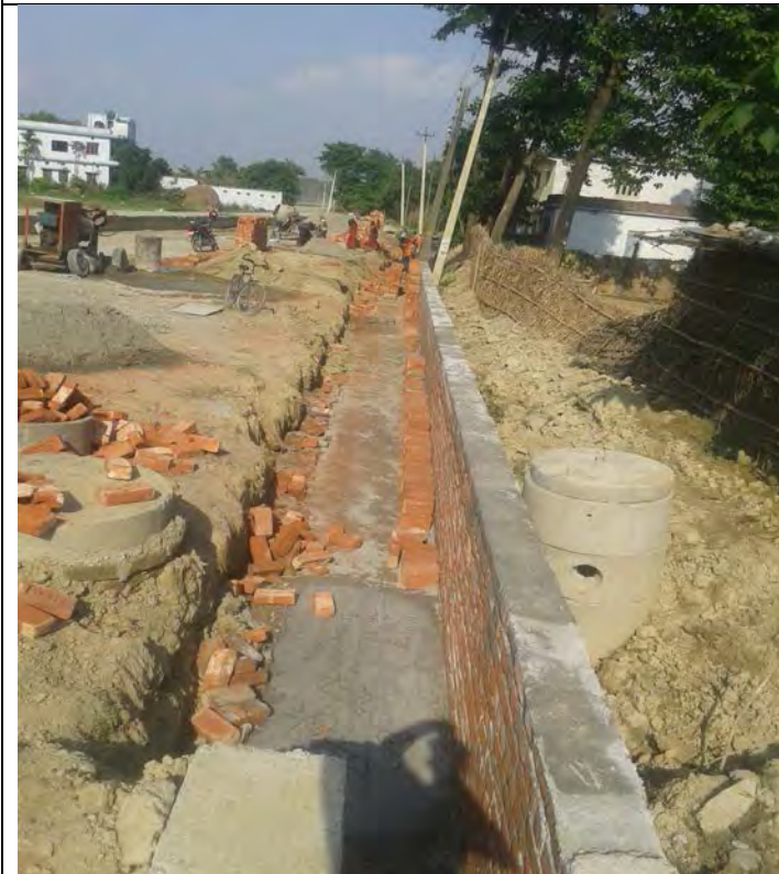
Construction of Road side Drain
