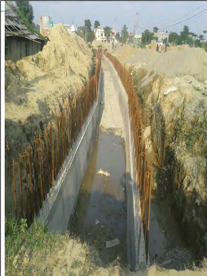
RCC Storm Drain at Line A1L2
