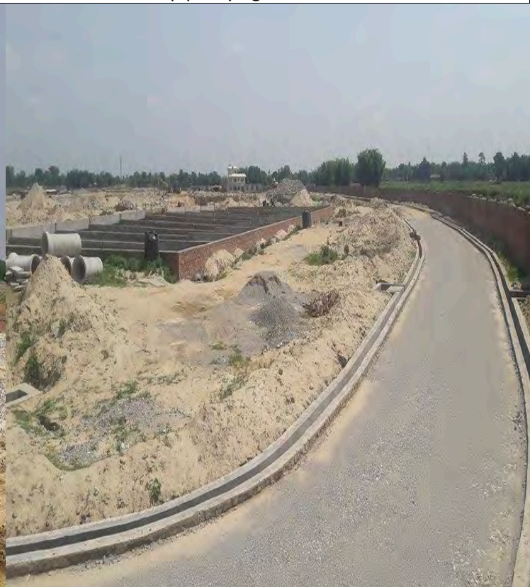
Sludge Drying BED
