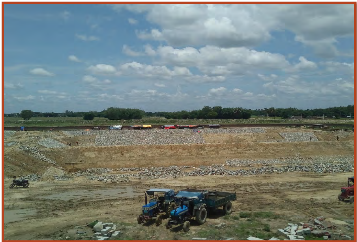
Rip Rap work at WWTP for Facultative pond
