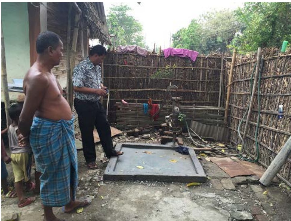
Figure 4. Platform for existing tubewells
