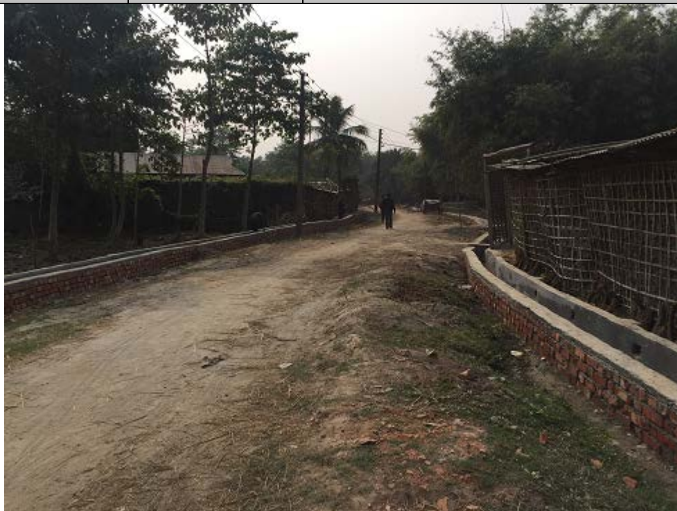
Figure 1. Pucca drains constructed under CDP
