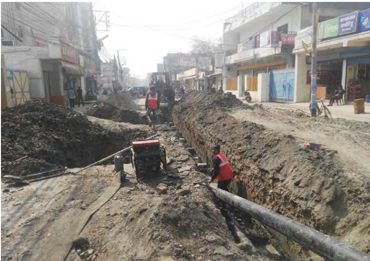
Sewer line placement Works at R2
