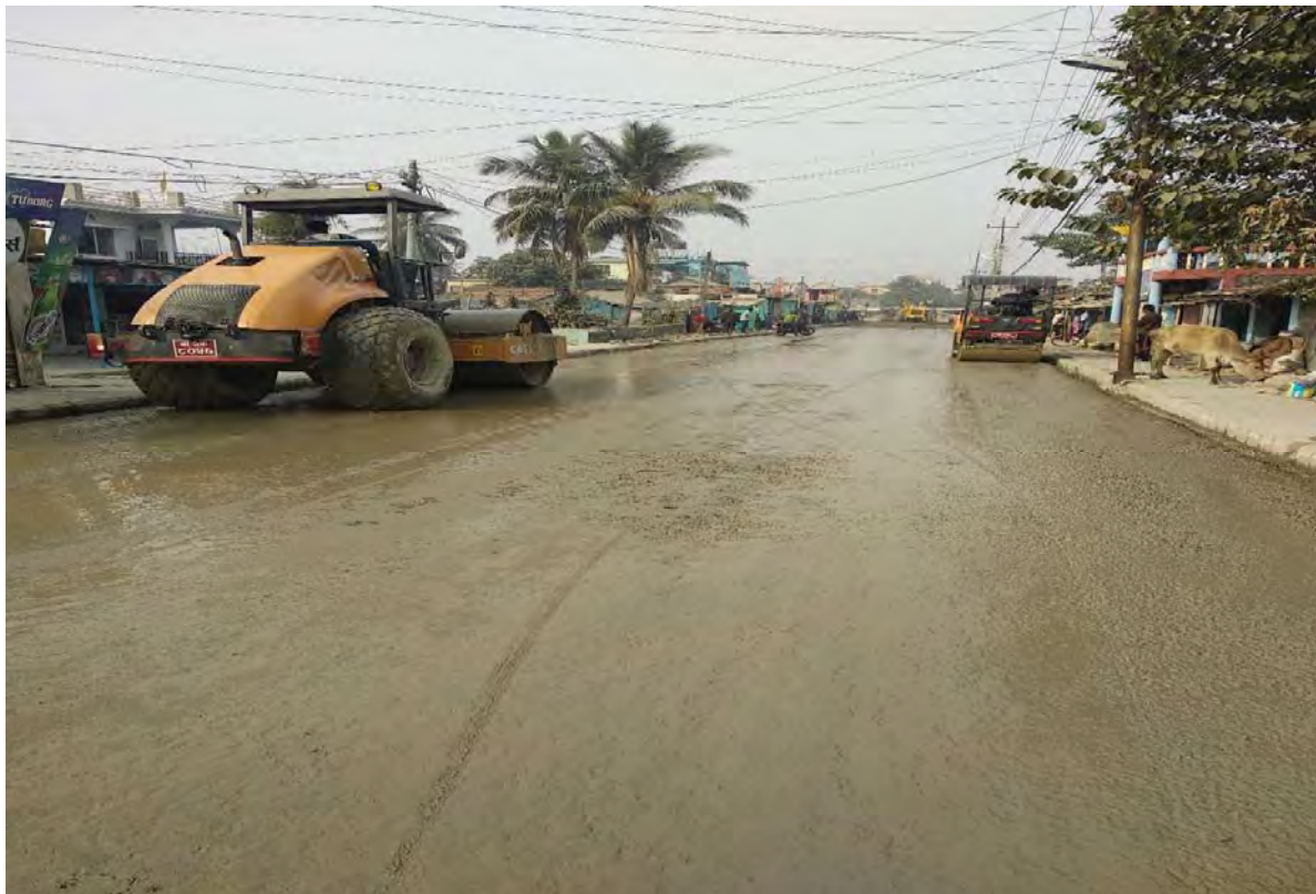
Base finishing Works at B2
