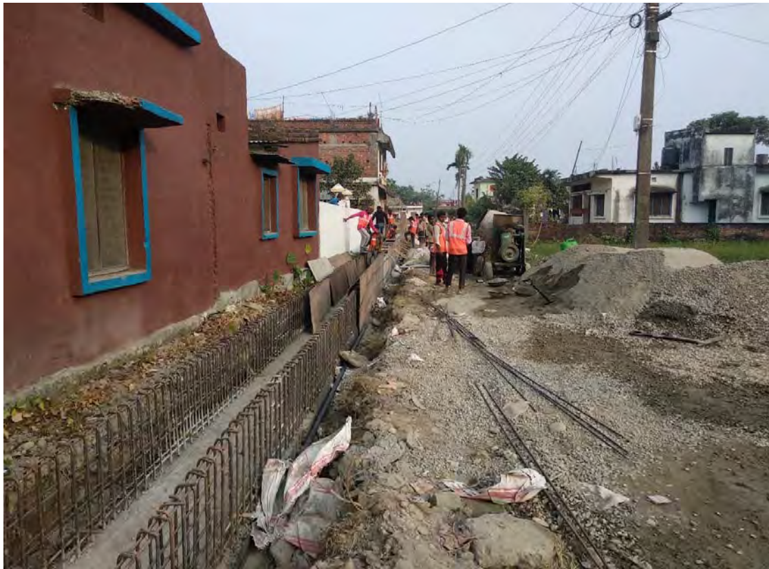
Road Drain work at R6
