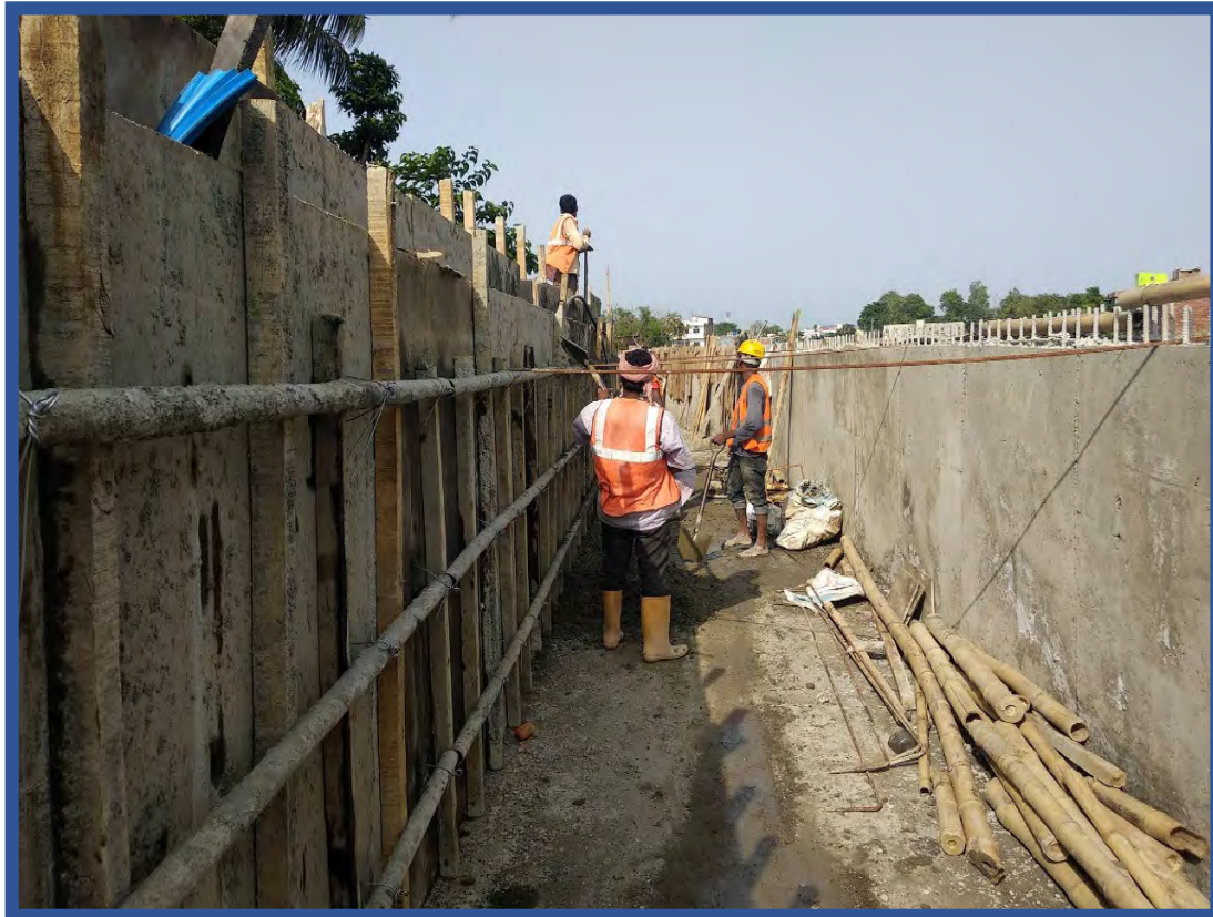
Shear Wall casting of Storm Drain at Chyangbari Nala
