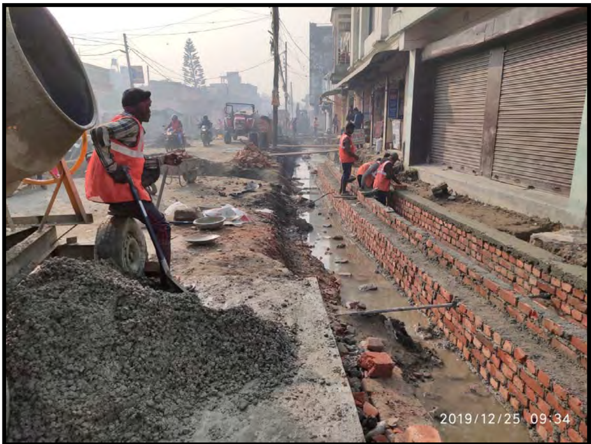
Brick Masonry drain at R2
