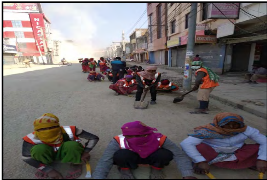
Brooming work before application of Prime coat at R2
