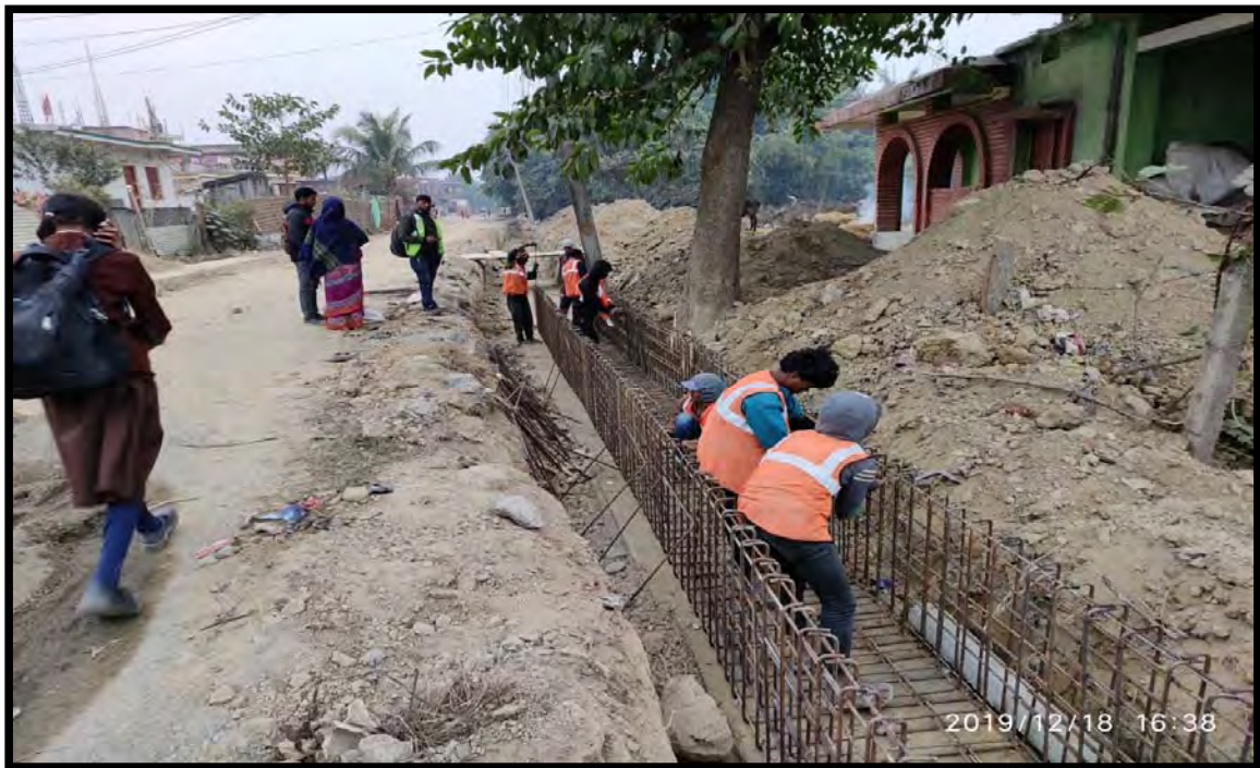
RCC Drain at R4 near N2 Junction
