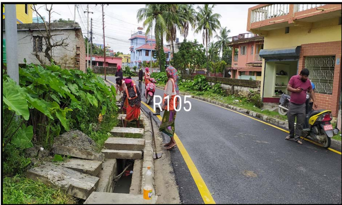
Drain cleansing R105
