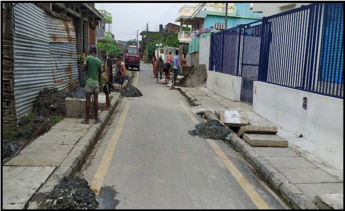
Drain cleansing at R9
