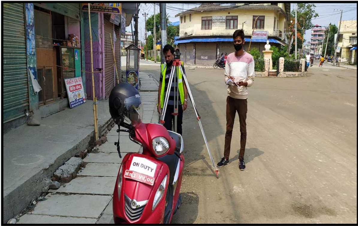
Base work at Devkota Chowk
