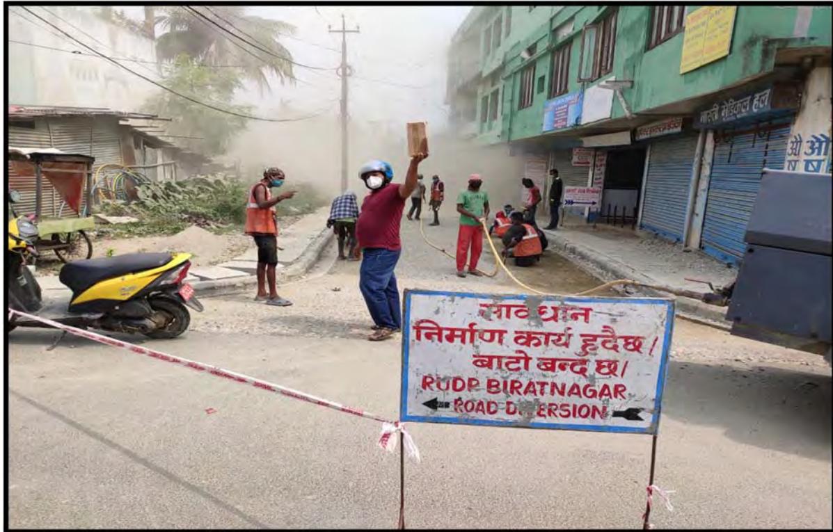
Brooming work at Sri Hospital road - T3Line10F
