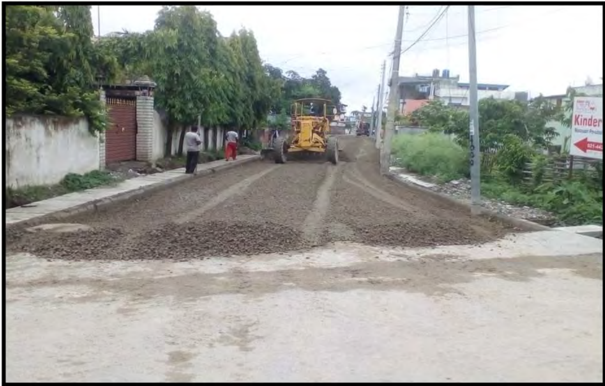
Base Laying at T3L25A
