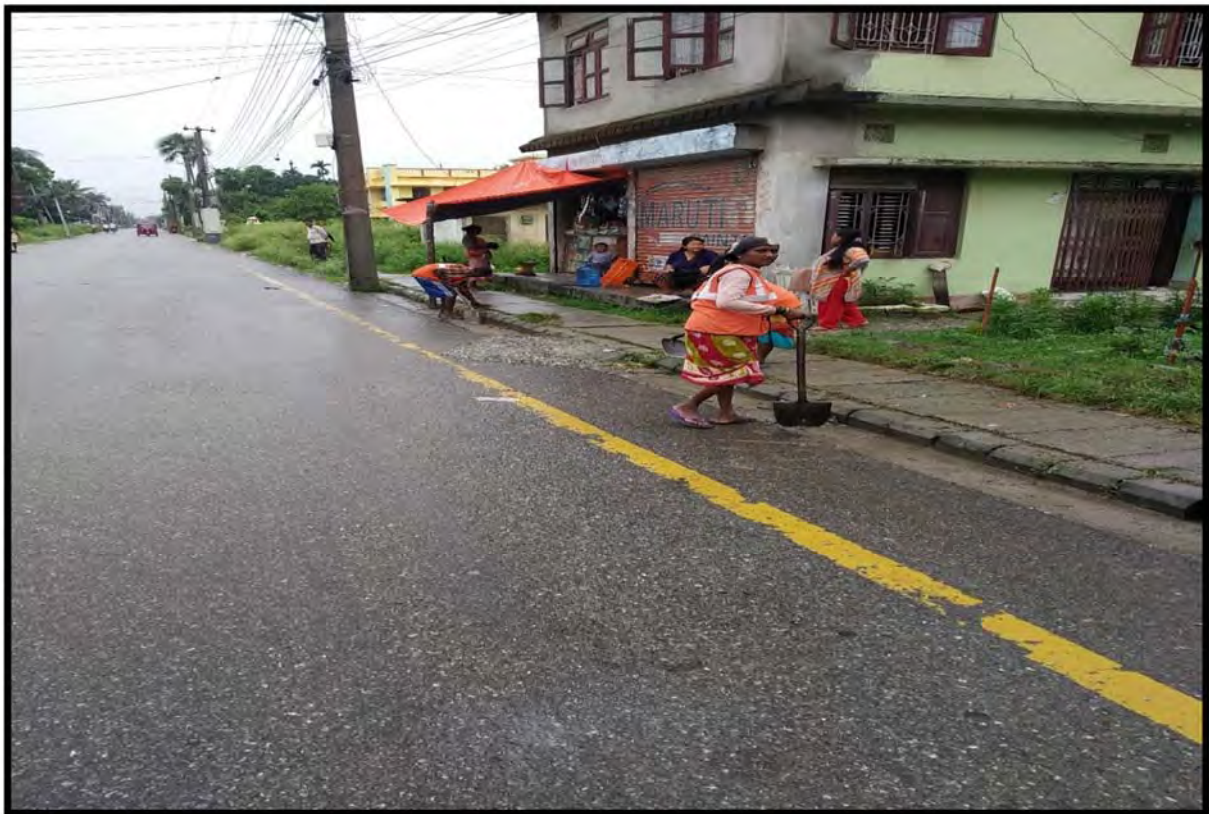
Gutter / Teak drain cleansing work at R114
