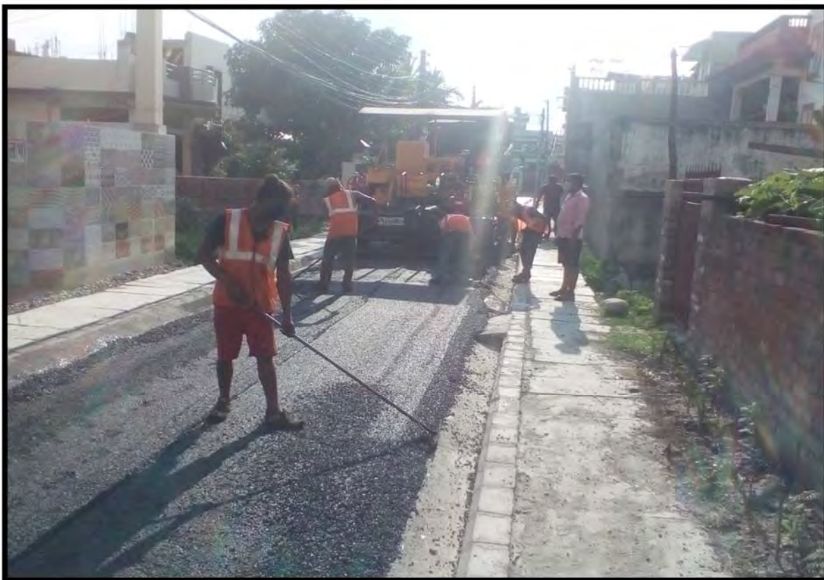
Asphalt laying at T2L18A
