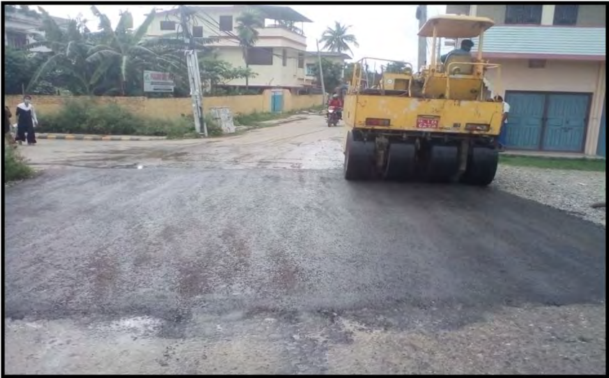
Maintenance work at Panchali Marga (R114)
