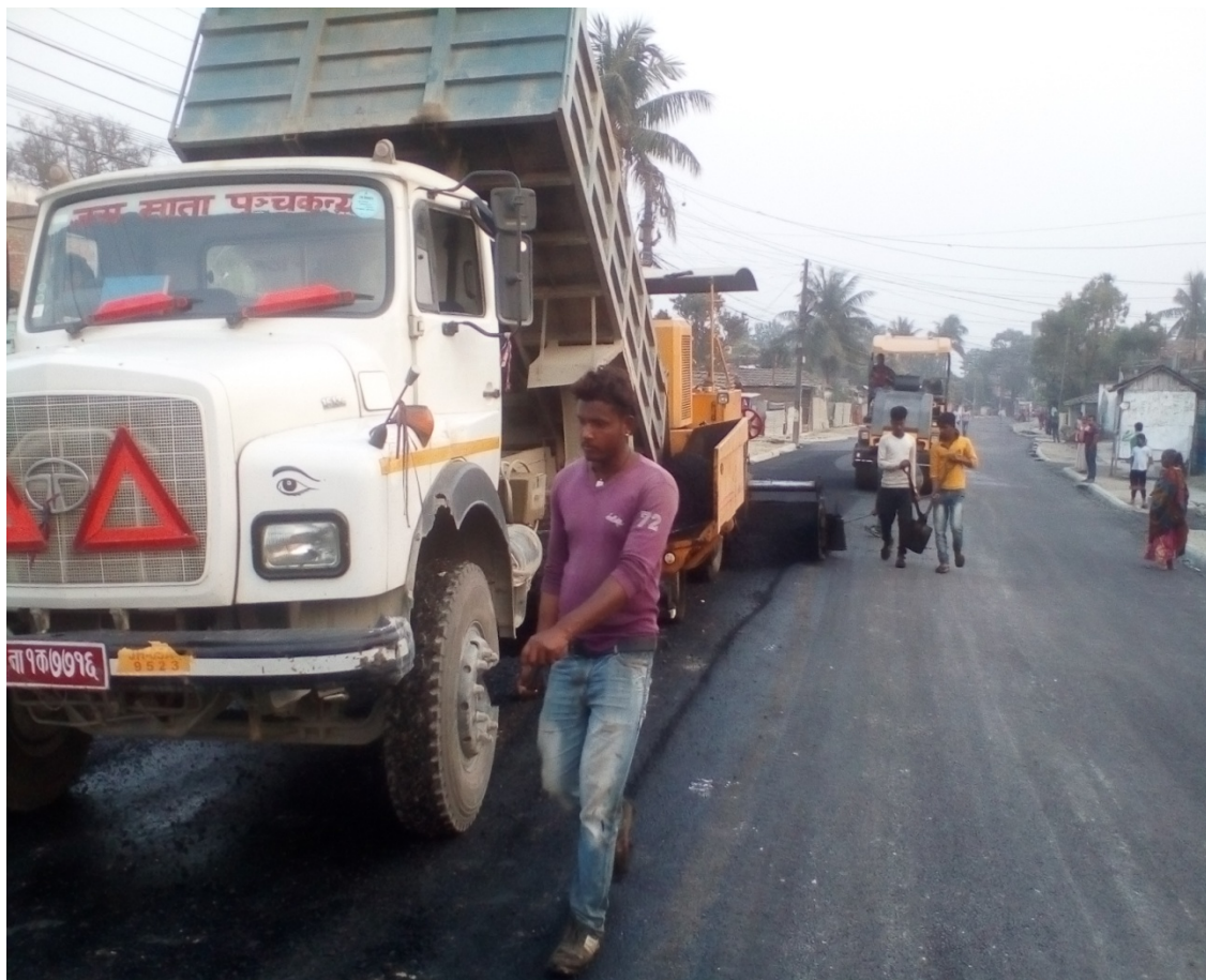
Asphalt work at T3 Trunk
