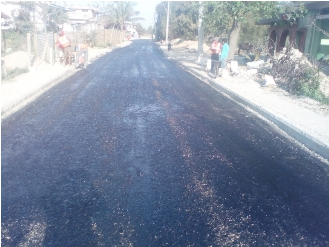
Prime coat work at R4
