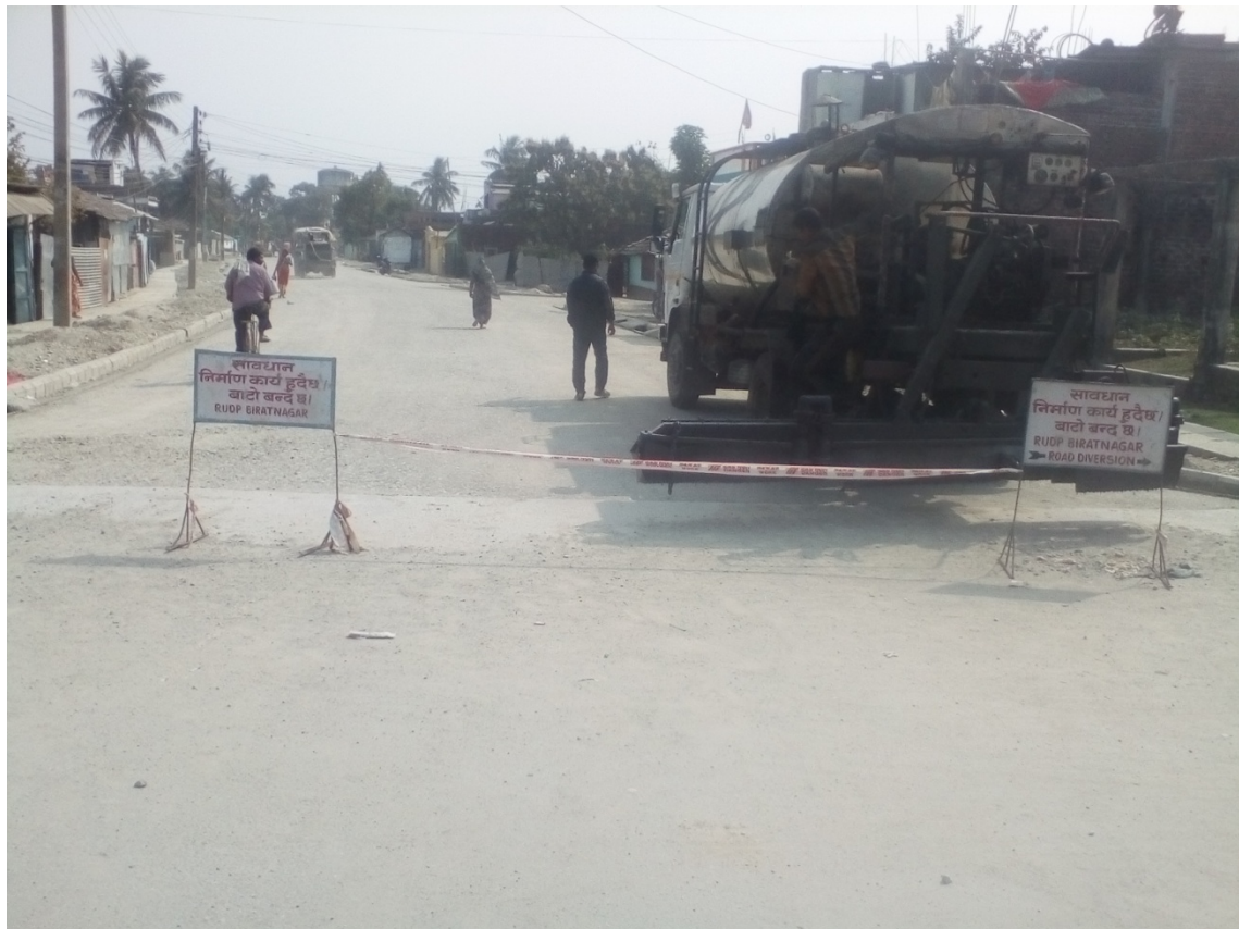
Commencement of Prime work at R2 (Tinpaini to Pani Tanki)
