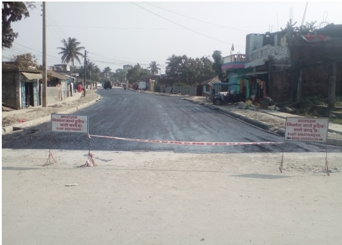
Prime coat work at R2 (Tinpaini to Pani Tanki)
