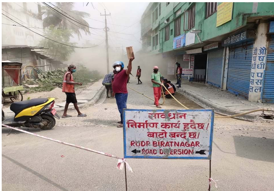
Surface Preparation for prime works at R6
