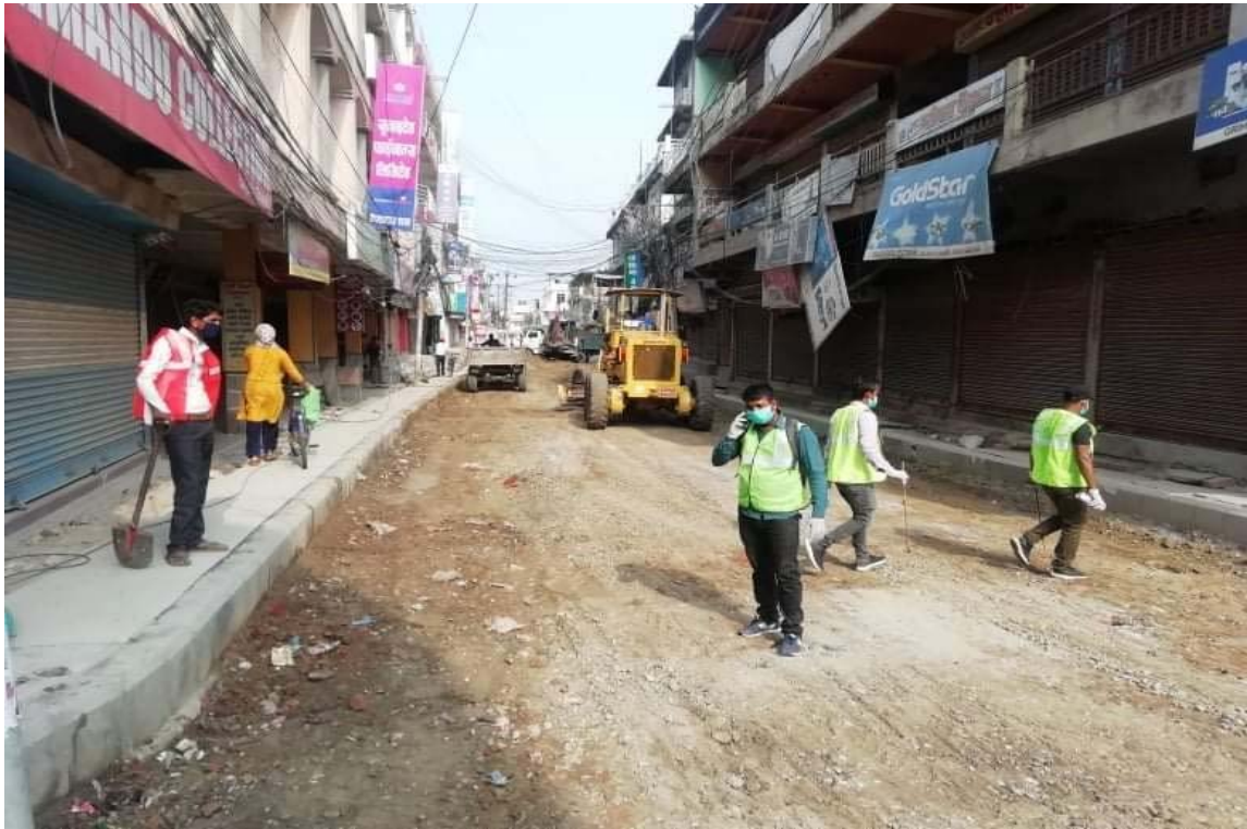
Sub Grade work at T2L24D
