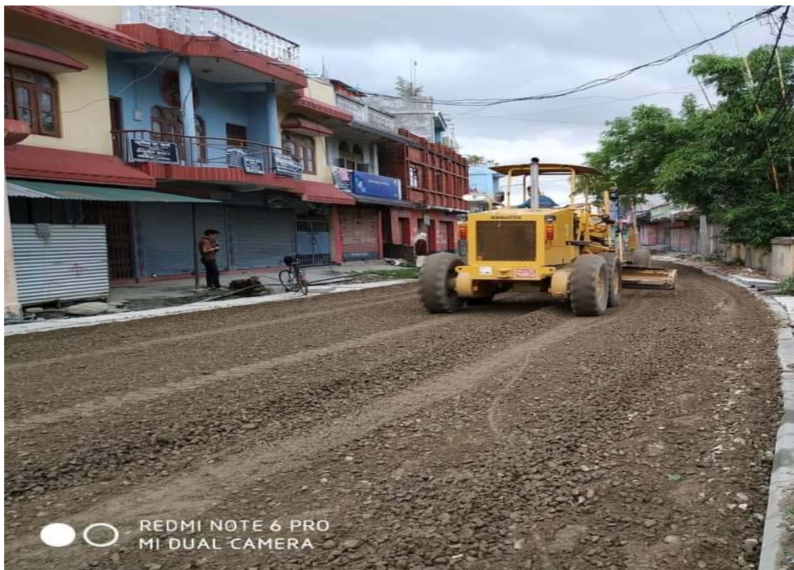
Base work at T3 Trunk
