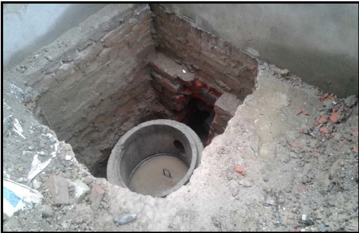
Placement of House Connection Chamber (HCC) at T3L12
