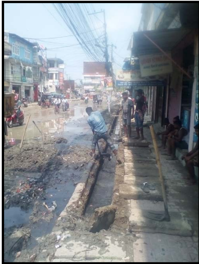
Cleaning of existing drain
