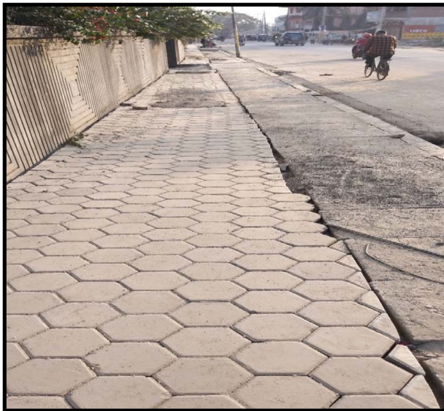
Interlocking work on footpath at R2
