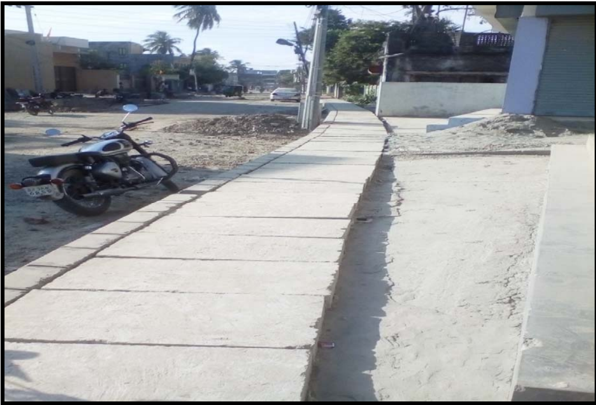
Drain cover slab & kerb stone works at R3
