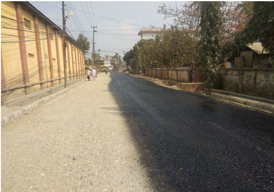
Prime coat Works at T3L6
