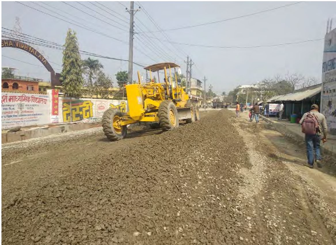
Base laying work at T3L6
