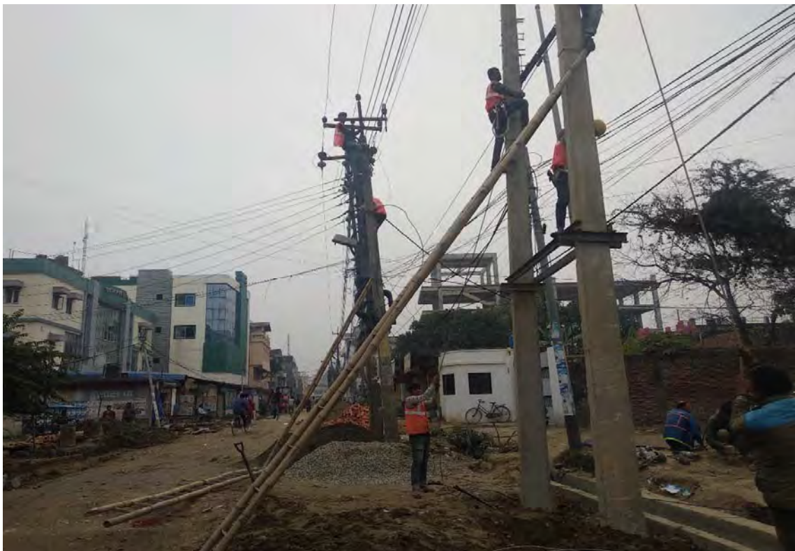
Relocation of electric poles at T3L6A
