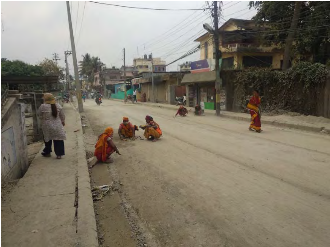
Brooming work before application of prime coat at R86
