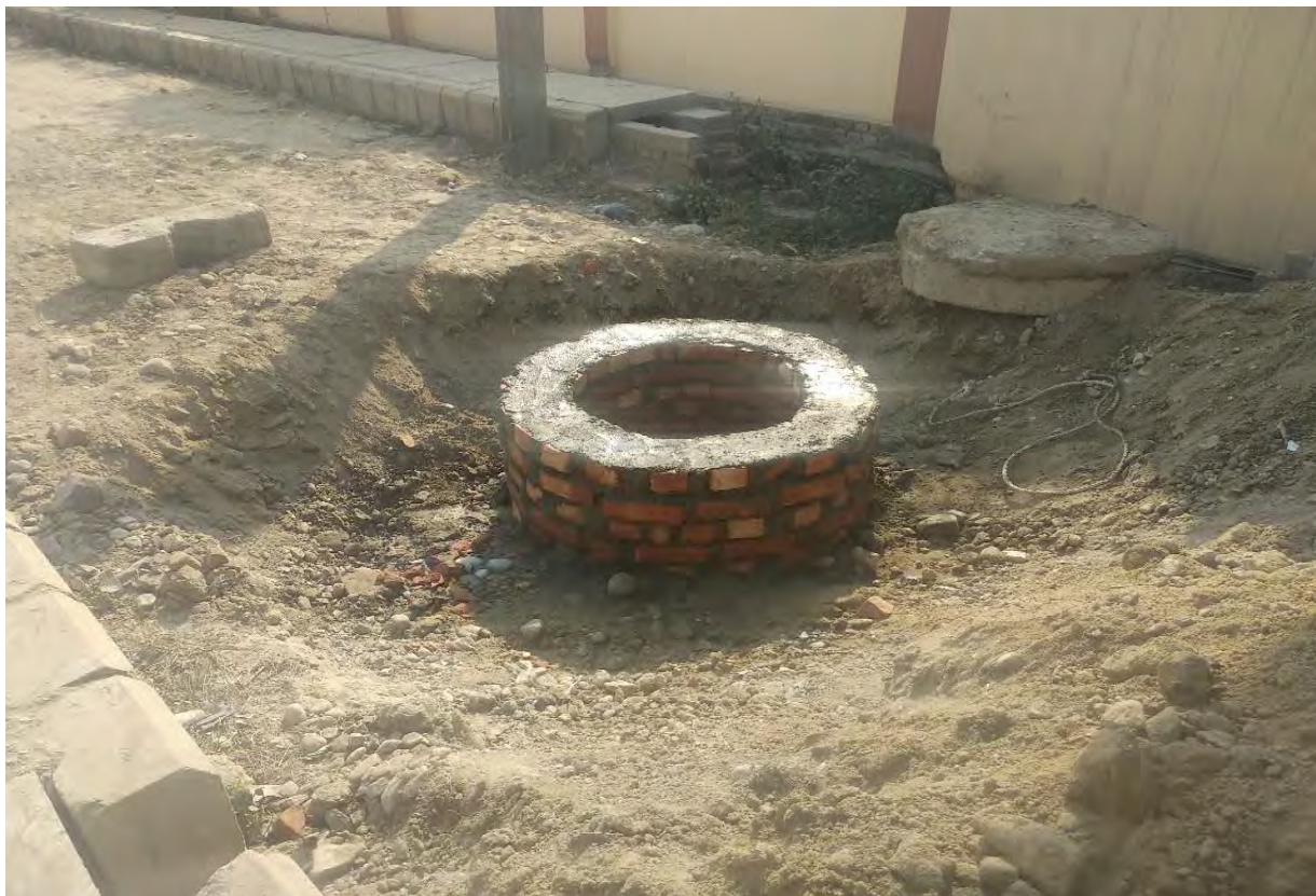
Raising of Sewer Manhole to achieve required design level at R77
