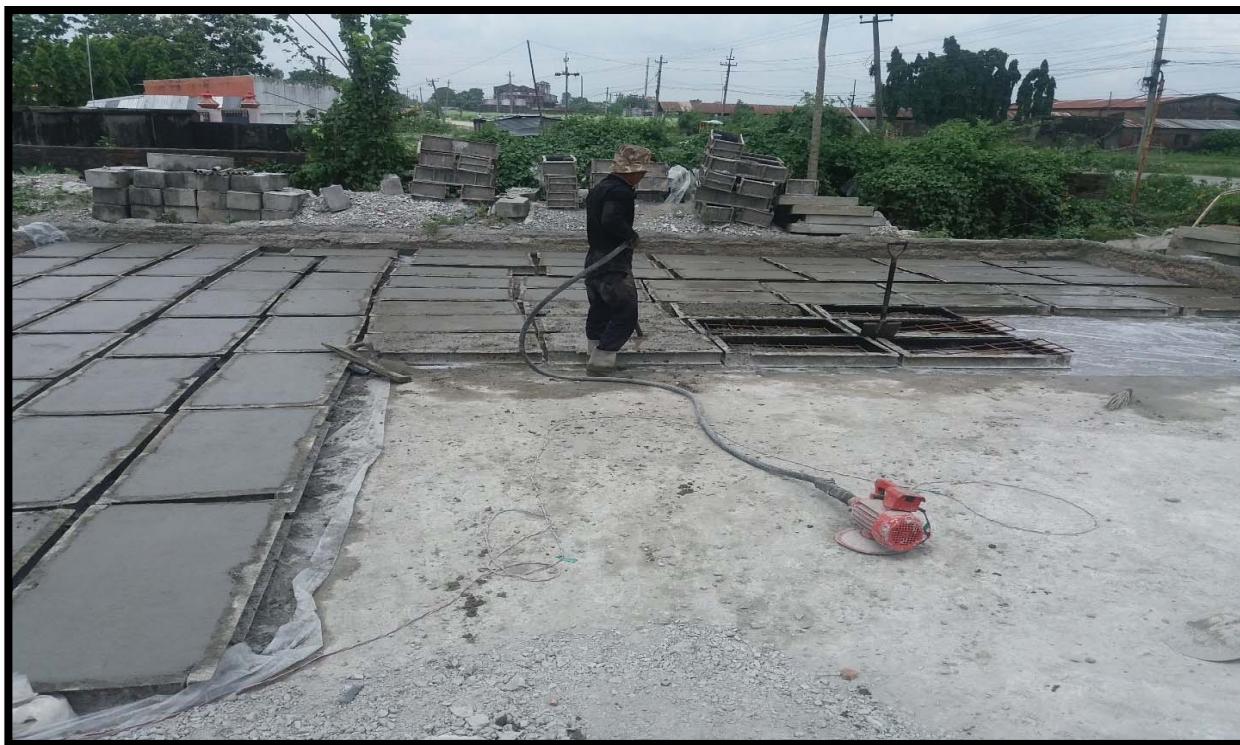
Production of precast slab at Precast Yard
