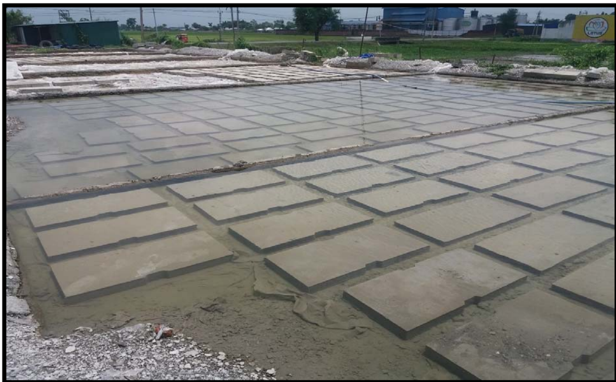
Curing of Precast slab at Precast Yard
