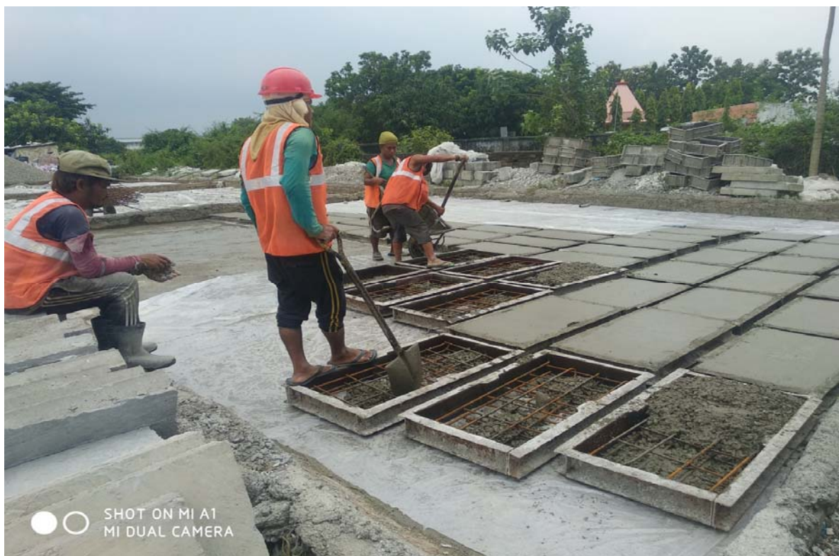
Precast element's casting at Contractor's yard
