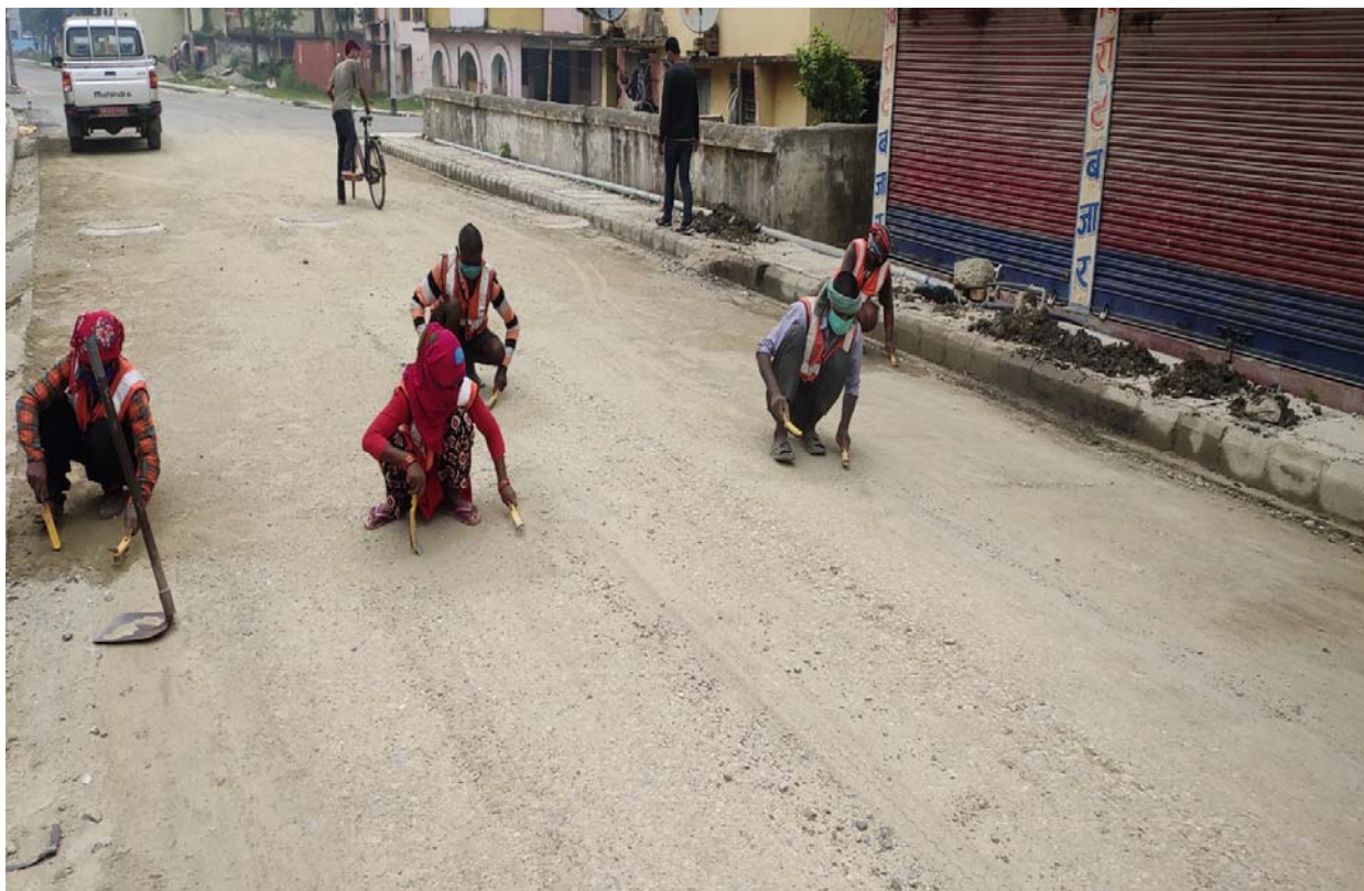
Brooming work at T3 Trunk
