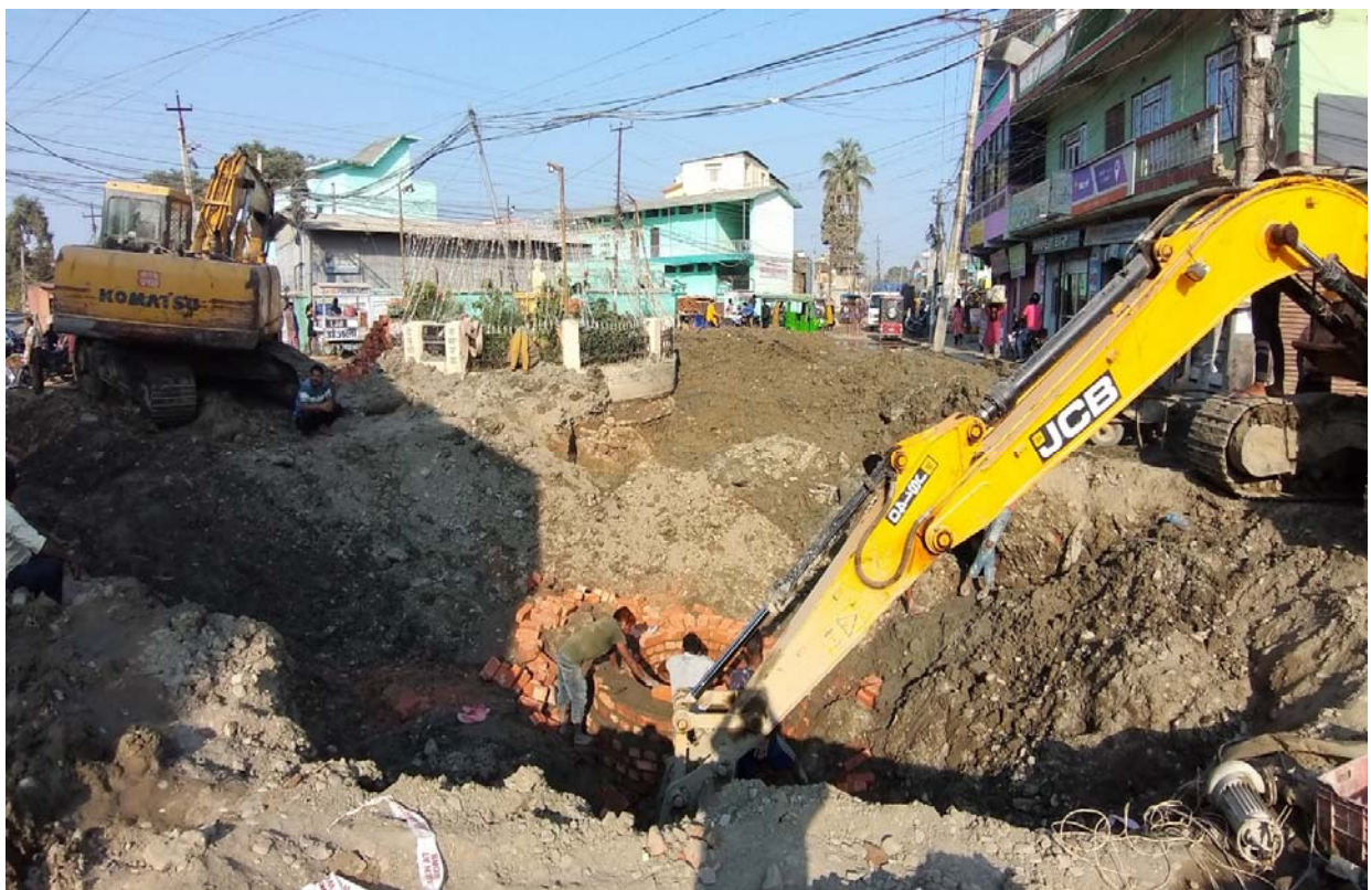
Brick Manhole of Sewer line at T3Line7
