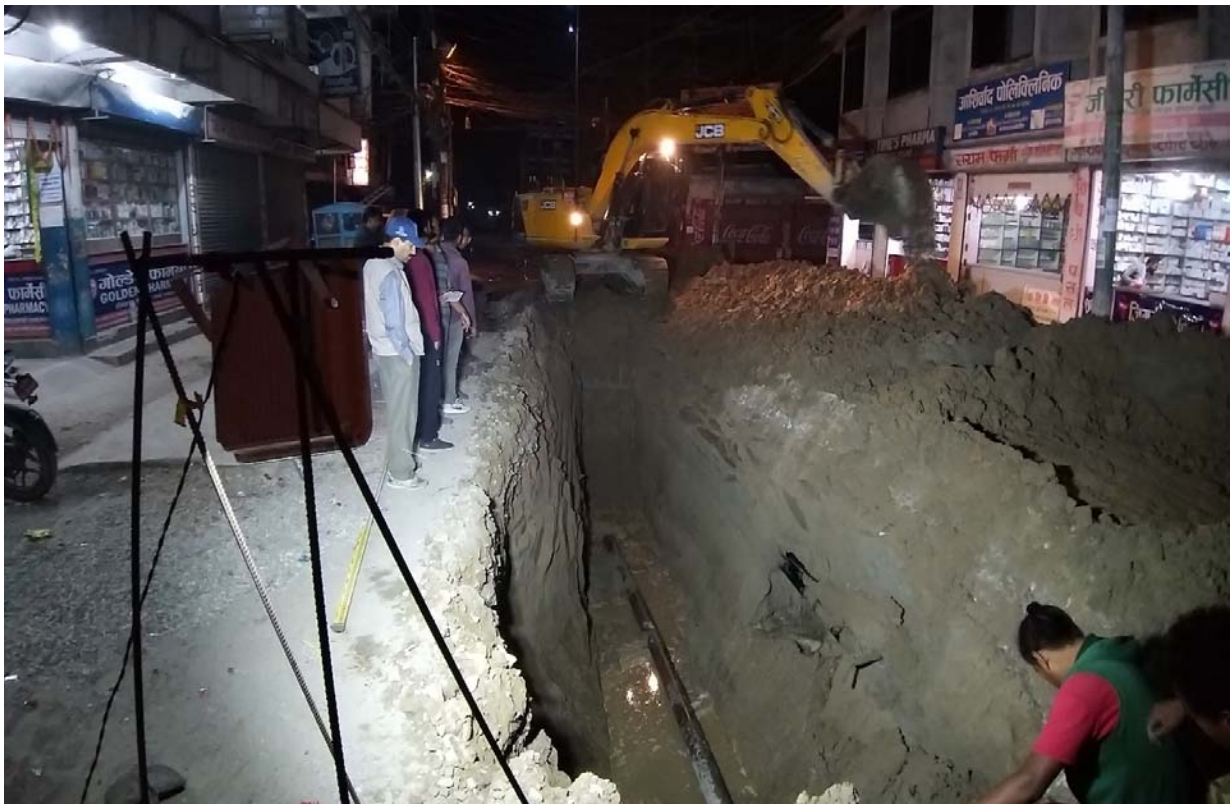
Laying of Sewer pipes at T3Line7
