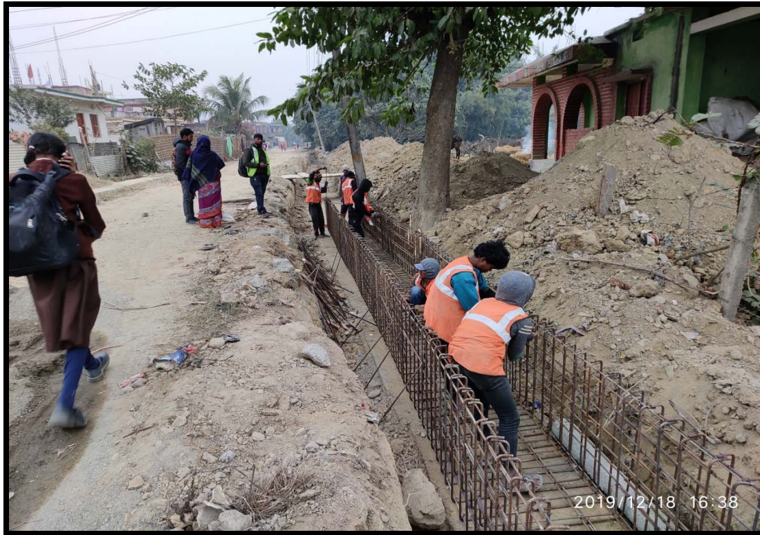
Photo 5: Road side drain under construction
