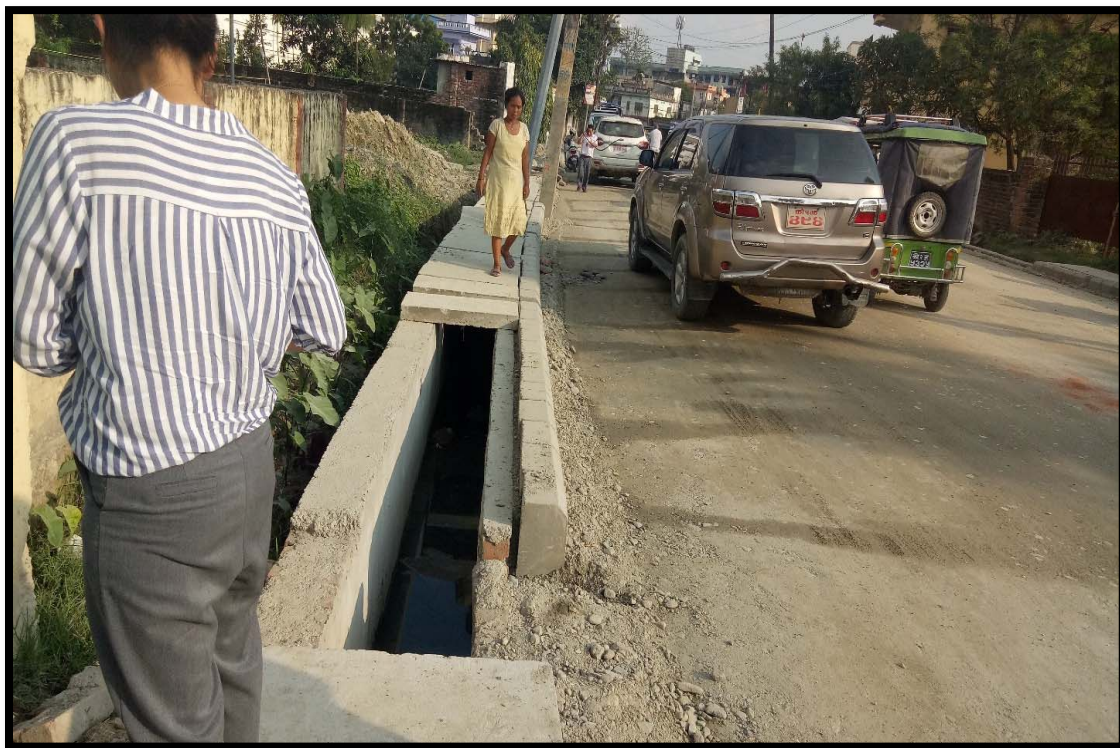
Photo 4: Ongoing Installation of side drain cover and laying of base course
