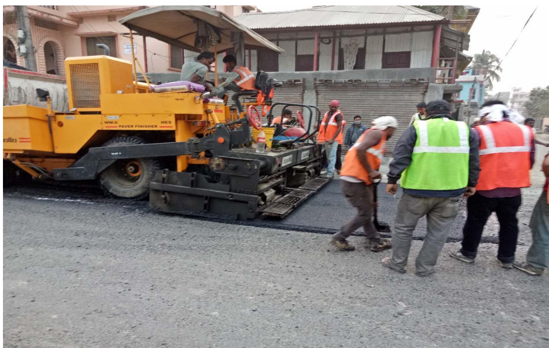
Photo 3: Asphalt pavement work under progress
