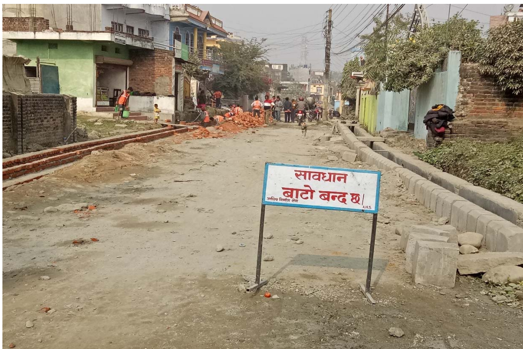
Photo 3: Road Side Drain Under construction
