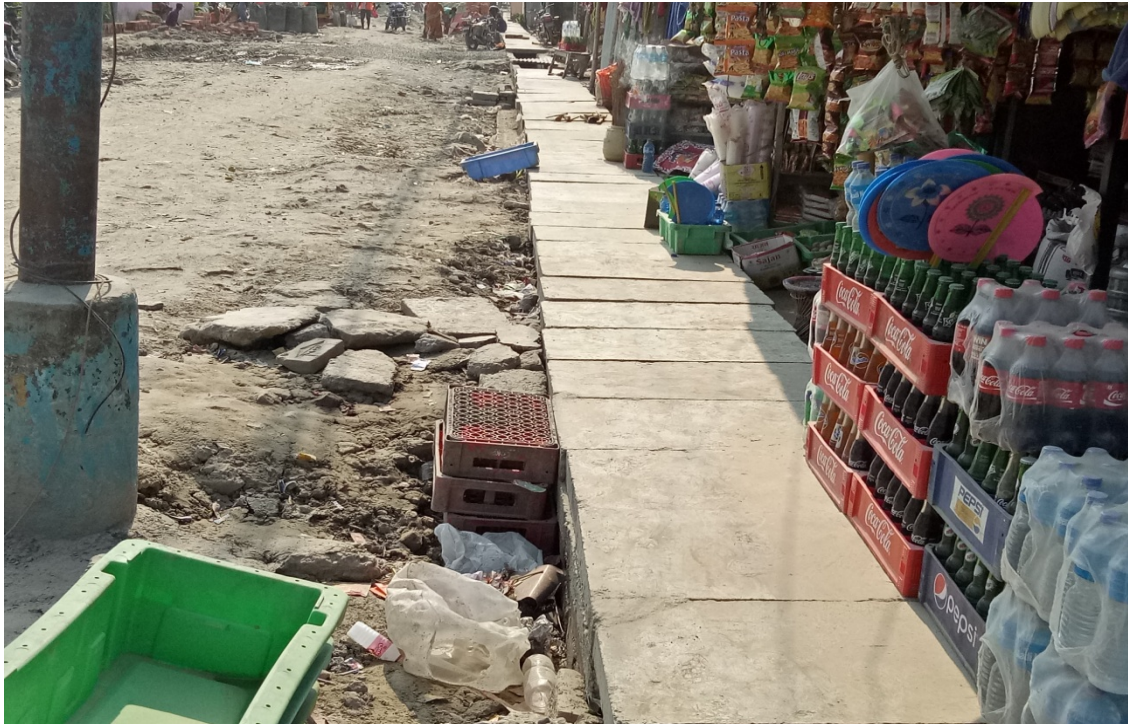
Photo 3: Road section with drain cover at DSP road section
