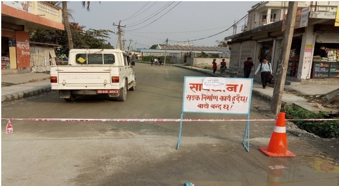
Photo 1: Sign board and barricade in Road section after laying of base course and making ready for asphalt concreting
