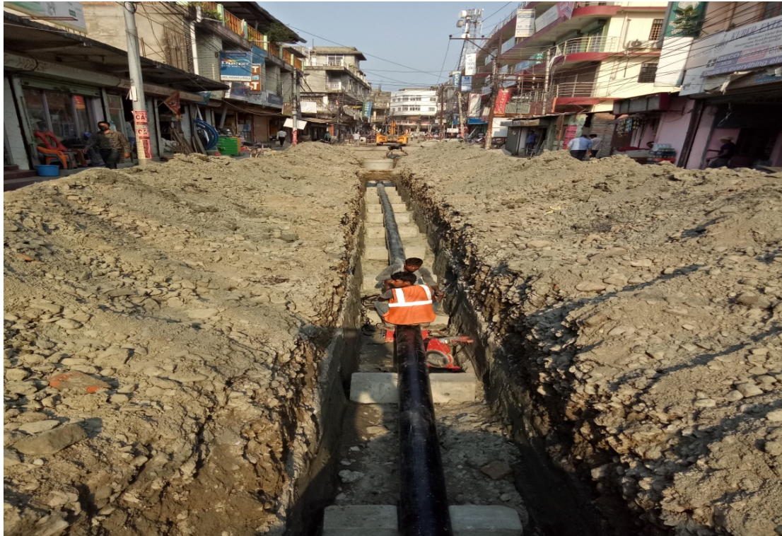
Photo 5: Laying of Sewrerage line along Hanuman Das road section
