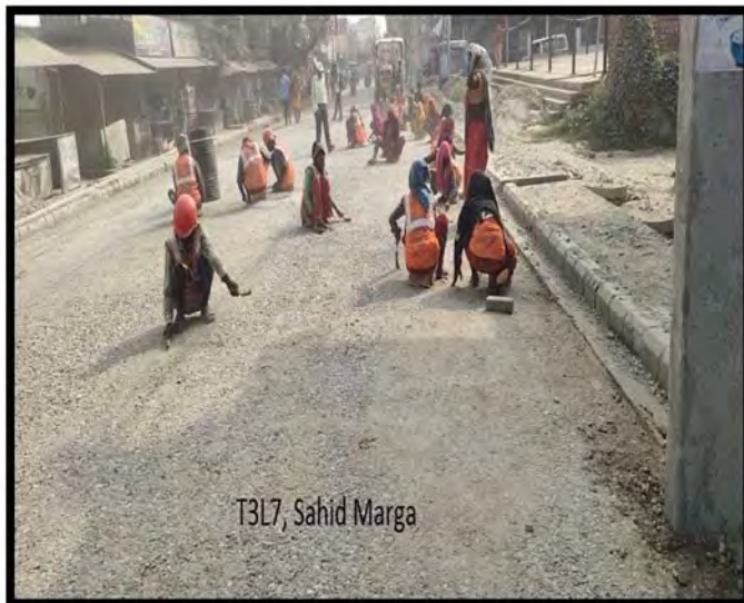
Road cleaning for to spread Asphalt in Sahid margha
