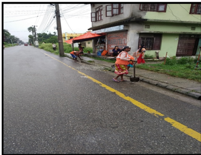
Gutter / Teak drain cleansing work at R114
