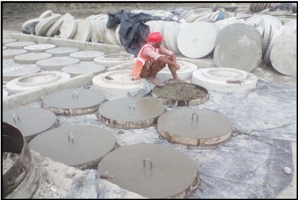
Precast element's casting at contractor's yard
