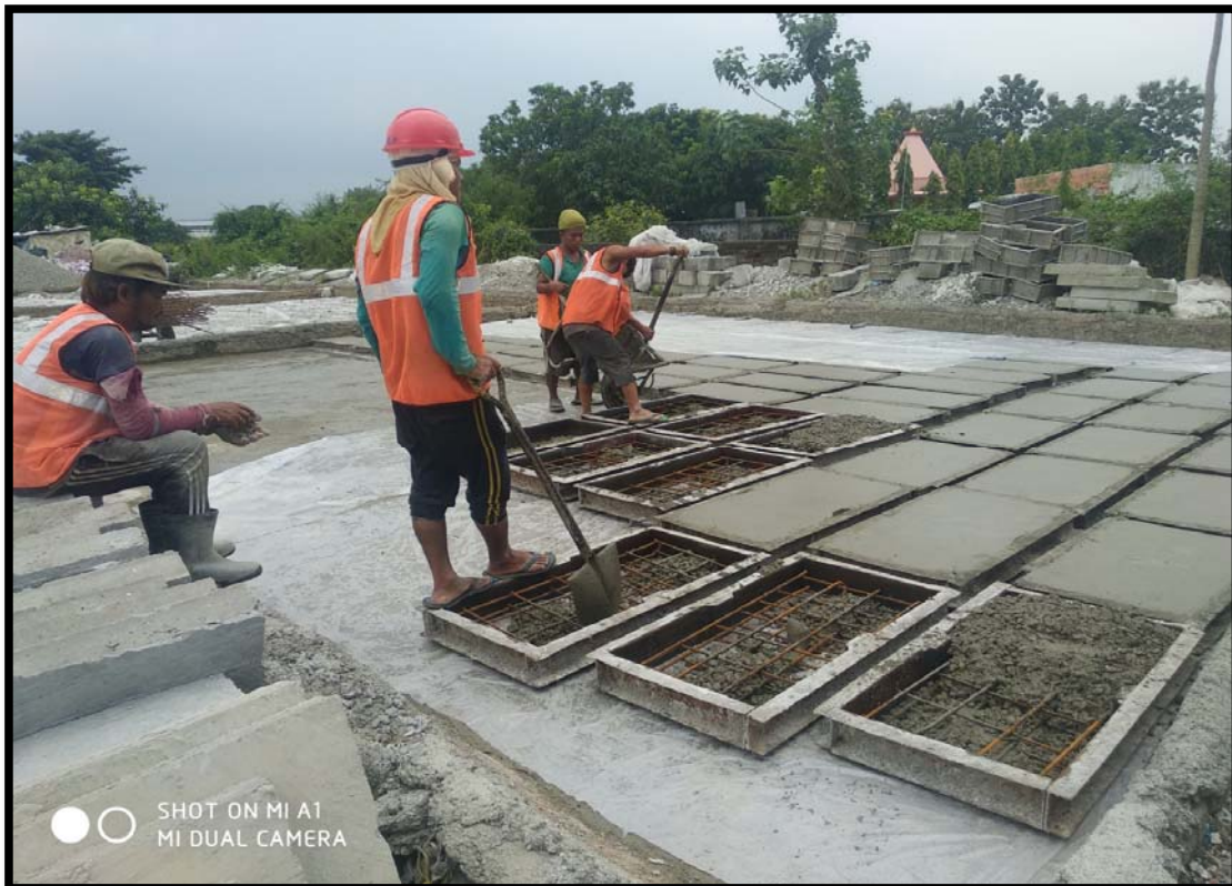
Precast element's casting at Contractor's yard
