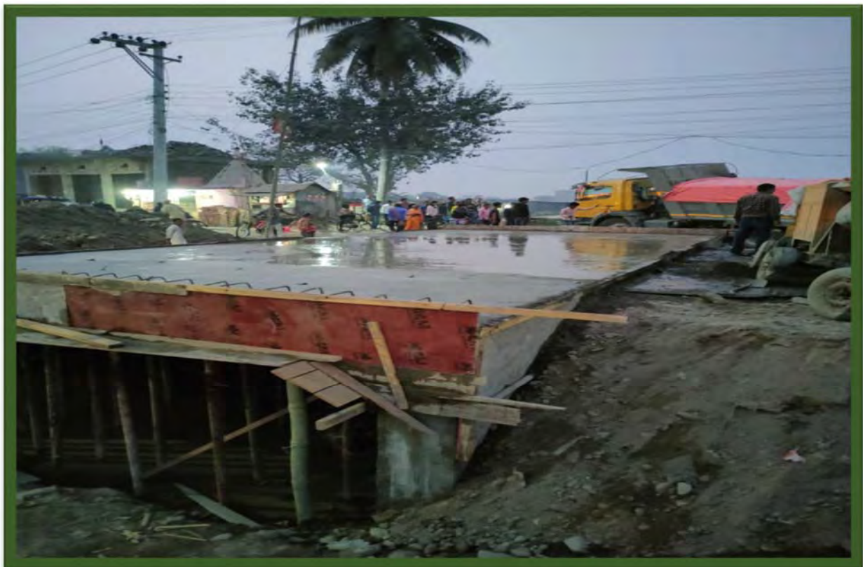
Culvert at Keshaliya road Canal
